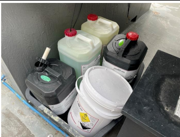
Photo 01. Class 5.1 and Class 8 chemicals stored in same container in cooling tower area.
