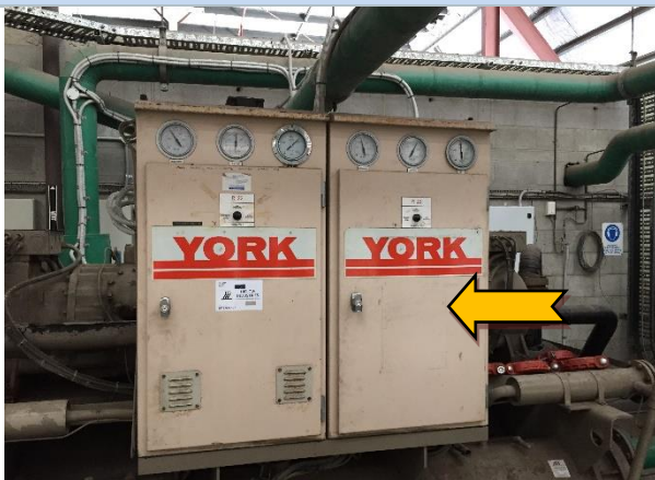
Photo 47 Interior: level 13, plant room, 'York' air conditioning unit – ozone depleting R22 Hydrochlorofluorocarbon (HCFC) refrigerant.
