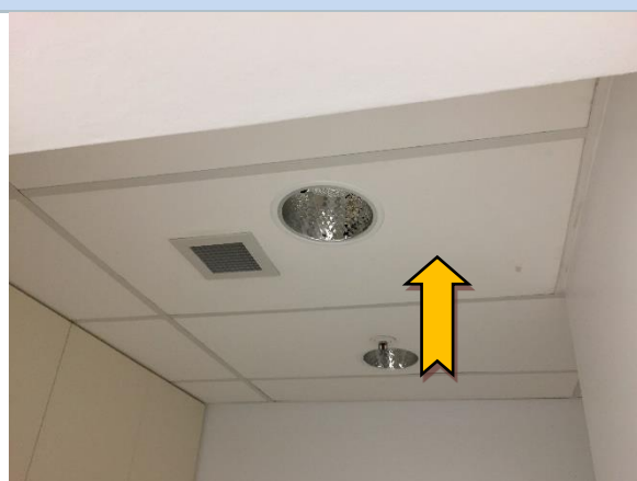
Photo 23 Interior: ground level to level 12, kitchenette, ceiling – suspected SMF compressed ceiling tiles.
