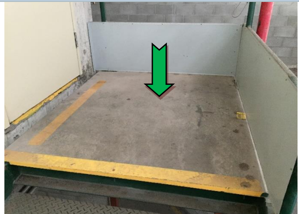
Photo 34 Interior: level 7, landing adjacent lift motor room, floor – non-asbestos containing compressed cement sheeting.
