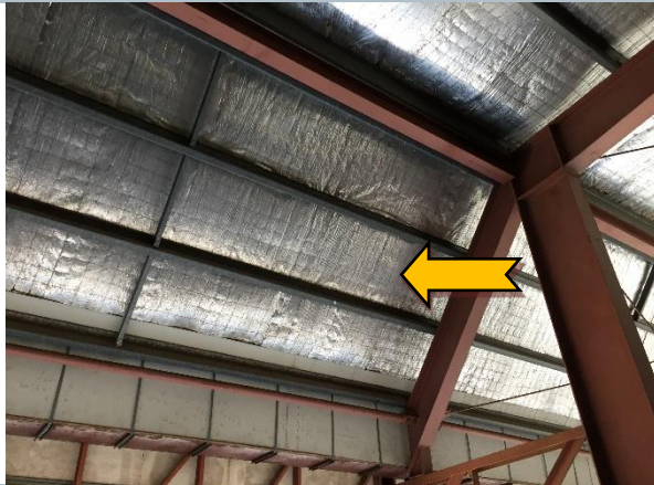
Photo 43 Interior: level 7, plant room, ceiling – suspected SMF sarking insulation.
