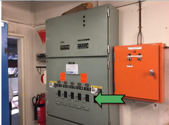
Photo 7 Interior: level 13, lift motor room, switchboard – non-asbestos containing arc shields.
