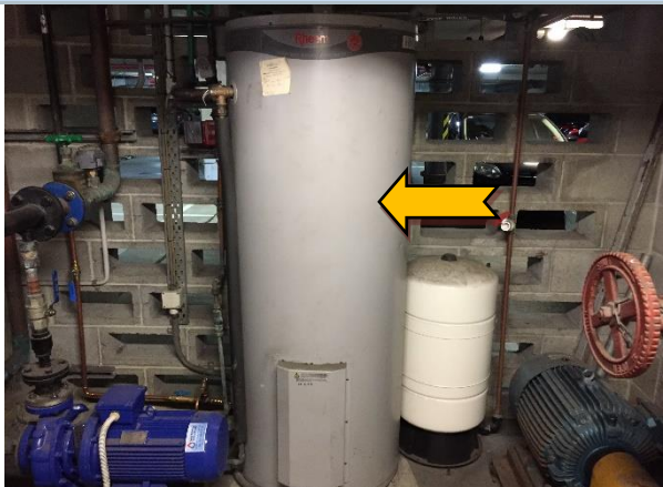
Photo 57 Interior: B2, Pump and Sprinkler rooms, 'Rheem' hot water heater – suspected SMF internal insulation material.
