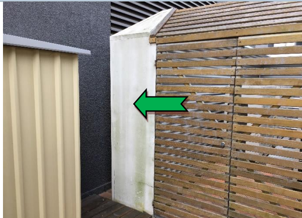
Photo 3 Exterior: level 3, air conditioning unit enclosure, external walls – non-asbestos containing fibre cement sheet.
