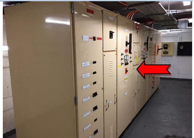
Photo 54 Interior: B2, MDF and switch rooms throughout, switchboard – suspected asbestos containing arc shields.
