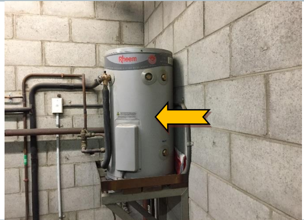
Photo 44 Interior: ground level to level 6, air handling rooms, 'Rheem' hot water heater – suspected SMF internal insulation material.
