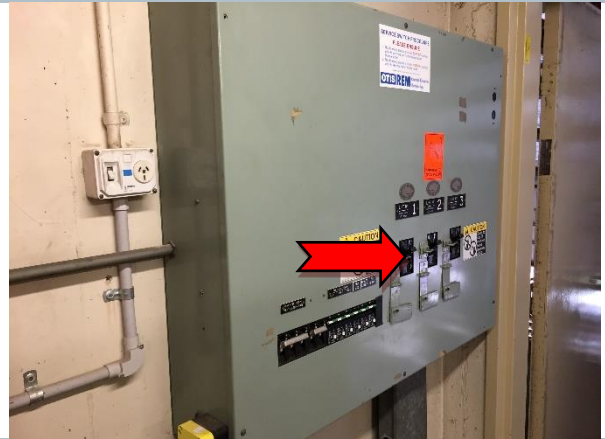
Photo 32 Interior: level 7, lift motor room, switchboard – suspected asbestos containing arc shields.
