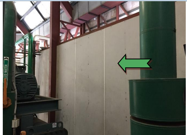
Photo 12 Interior: level 13, plant room, partition wall – non-asbestos containing fibre cement sheet.
