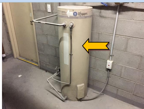
Photo 21 Interior: level 12, air handling room, 'Rheem' hot water heater – suspected SMF internal insulation material.
