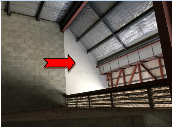
Photo 35 Interior: level 7, plant room, internal walls – suspected asbestos containing fibre cement sheet.
