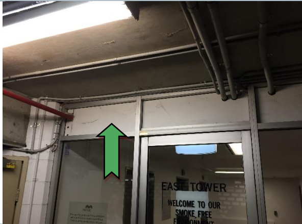
Photo 55 Interior: B1 and B2 East Tower and West Tower lift foyer Infill panels Fibre cement sheet
