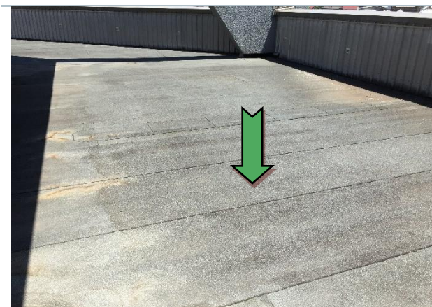
Photo 25 Exterior: level 7, roof top adjacent to plant room, waterproof membrane – non-asbestos containing bituminous membrane.
