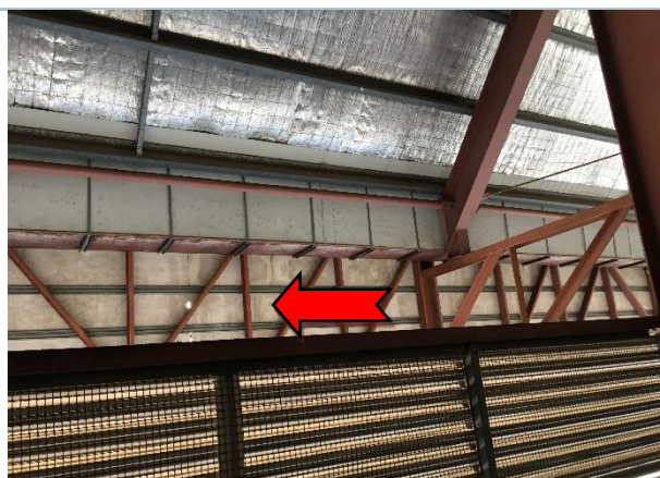
Photo 26 Exterior: level 7, plant room, external walls – suspected asbestos containing fibre cement sheet.
