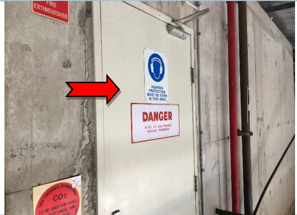
Photo 8 Interior: level 13, lift motor room, fire door - single (unlabelled) – suspected asbestos containing internal insulation material.
