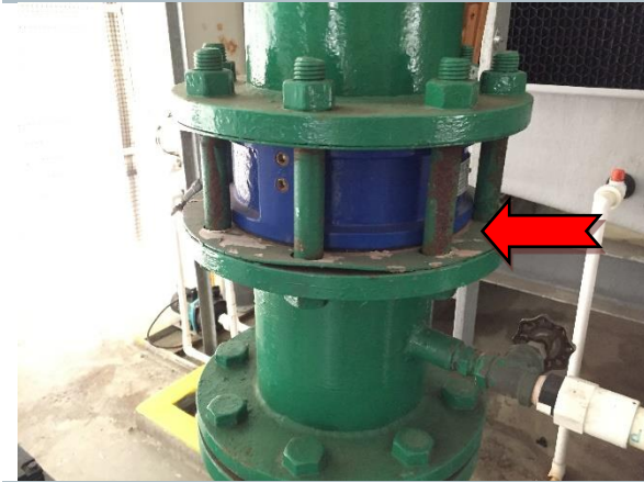
Photo 13 Interior: level 13, plant room, pipe work – asbestos containing gasket material.
