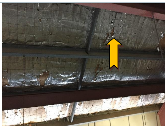
Photo 20 Interior: level 13, plant room, ceiling – suspected SMF sarking insulation.
