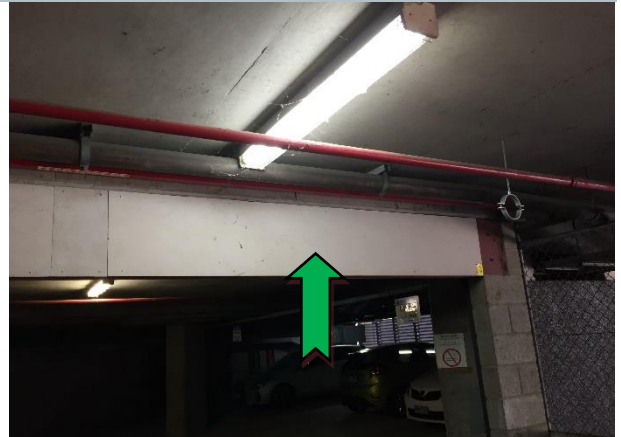
Photo 52 Interior: B1, West Tower carpark, above roller door, fascia – non-asbestos containing fibre cement sheet.
