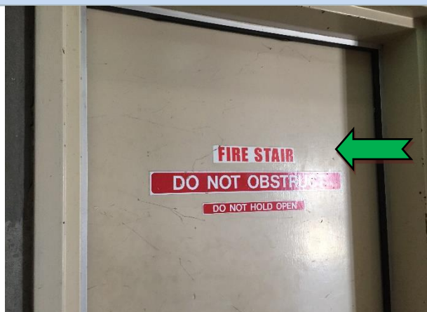
Photo 29 Interior: all levels, eastern fire stairwell, fire doors (1987) – non-asbestos containing internal insulation material.
