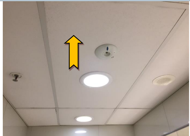
Photo 46 Interior: ground level, disabled amenities, ceiling – suspected SMF compressed ceiling tiles.
