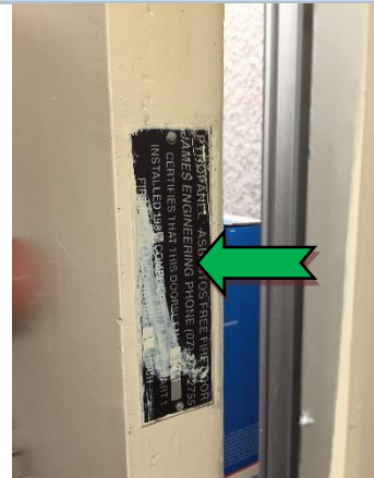
Photo 4 Interior: all levels, south eastern fire stairwell, fire doors (1987) – non-asbestos containing internal insulation material.
