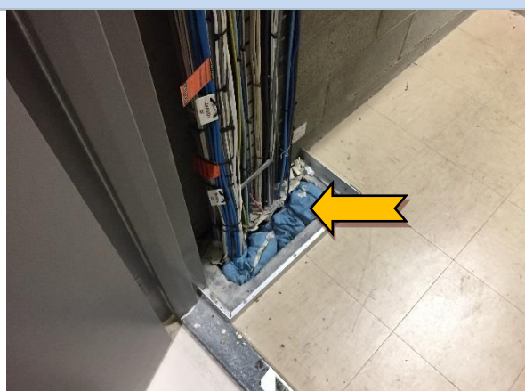
Photo 24 Interior: ground level to level 12, electrical server room, packer – suspected SMF pillow insulation.
