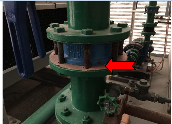
Photo 36 Interior: level 7, plant room, pipe work – asbestos containing gasket material.
