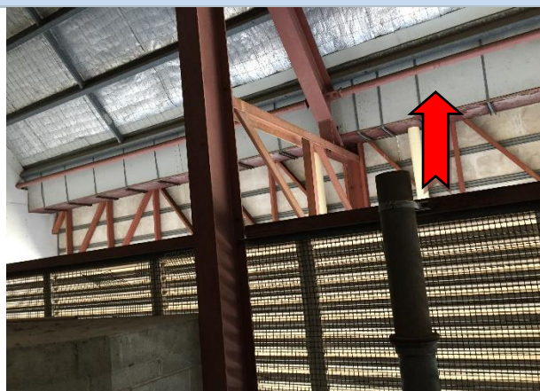
Photo 27 Exterior: level 7, plant room, soffit – suspected asbestos containing fibre cement sheet.
