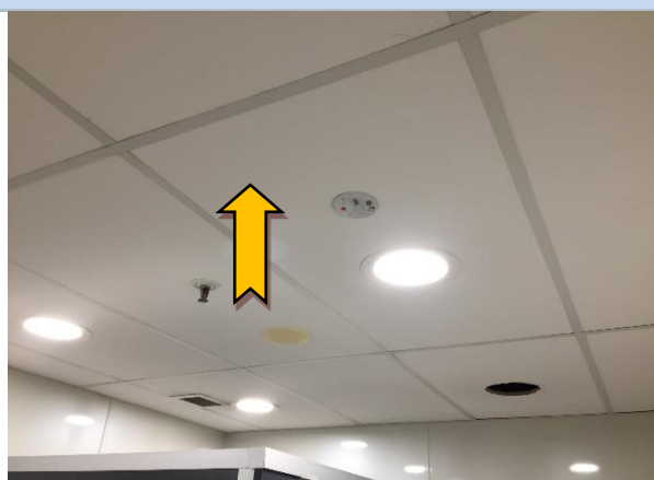
Photo 22 Interior: ground level to level 12, male amenities, ceiling – suspected SMF compressed ceiling tiles.
