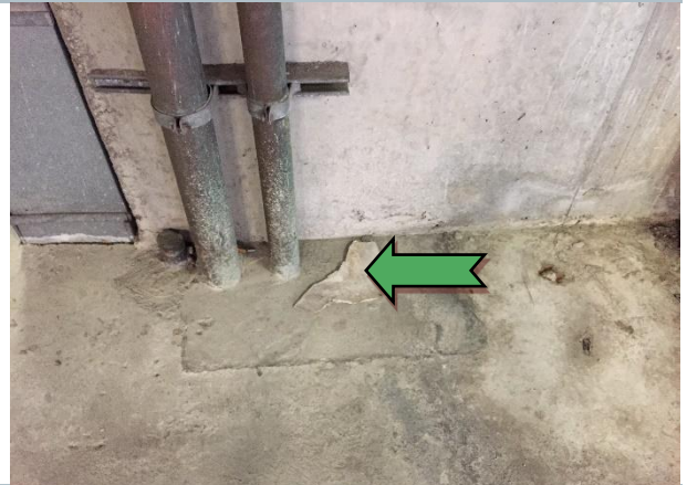
Photo 50 Interior: B1, West Tower lift foyer, near fire stairs 1, debris – non-asbestos containing fibre cement sheet.
