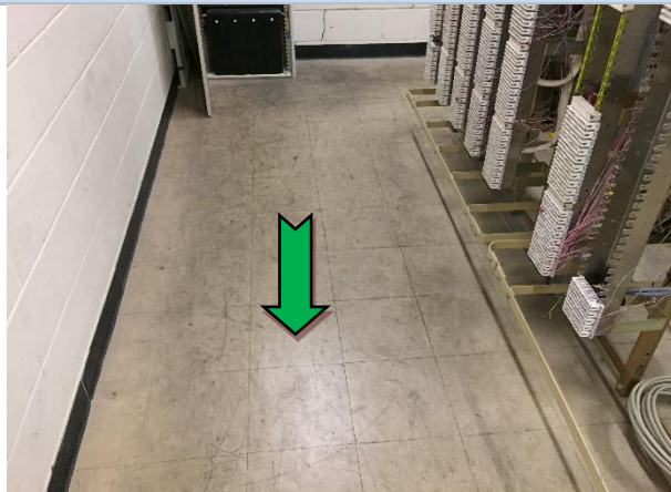
Photo 53 Interior: B2, MDF room, floor coverings (beige) – non-asbestos containing vinyl floor tiles.
