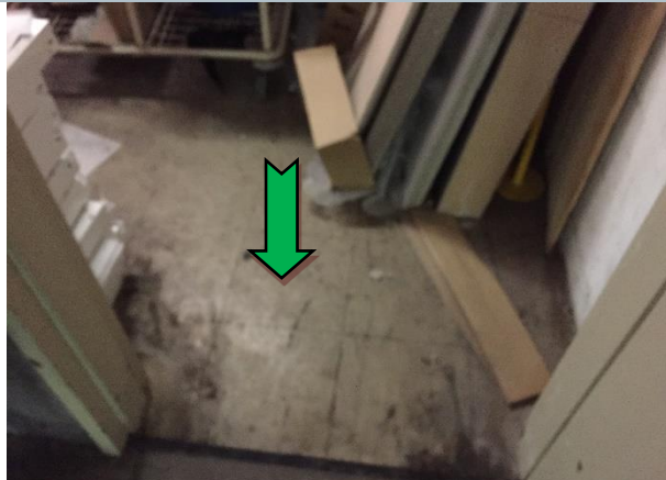
Photo 51 Interior: B1, West Tower storeroom adjacent switchroom, floor coverings (beige) – non-asbestos containing vinyl floor tiles.
