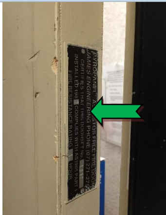
Photo 5 Interior: all levels, north western fire stairwell, fire doors (1987) – non-asbestos containing internal insulation material.
