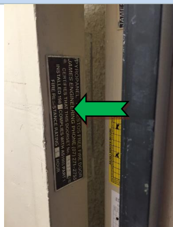
Photo 30 Interior: all levels, western fire stairwell, fire doors (1987) – non-asbestos containing internal insulation material.
