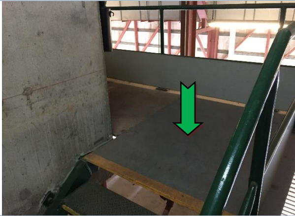
Photo 9 Interior: level 13, landing adjacent lift motor room, floor – non-asbestos containing compressed cement sheeting.
