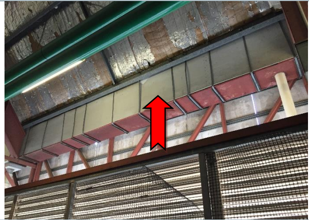
Photo 2 Exterior: level 13, plant room, soffit – suspected asbestos containing fibre cement sheet.
