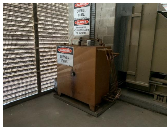
Photo 6 Diesel Generator Room, Diesel Fuel Storage
