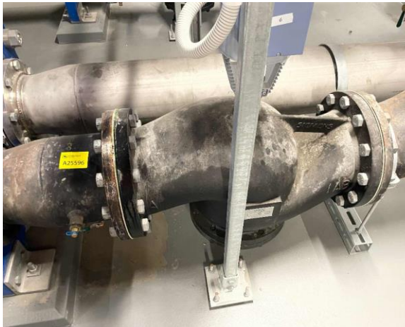
Line ID 4: Internal, Level 6, Chiller Room, to Condenser Water Pipework, Gasket Material - No Asbestos Detected
