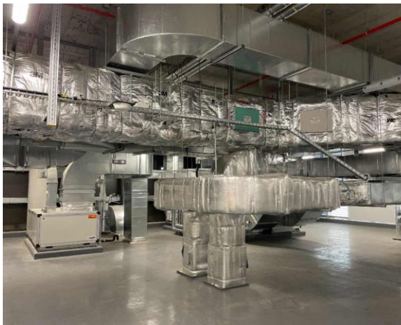
Line ID 26: Internal, Level 32, Plant Room Throughout, Air Conditioning Ductwork, Insulation Material - Suspected SMF
