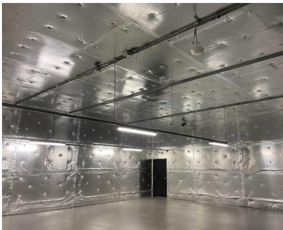
Line ID 28: Internal, Level 6, Generator Room, Throughout Wall and Ceiling Lining, Insulation Material - Suspected SMF
