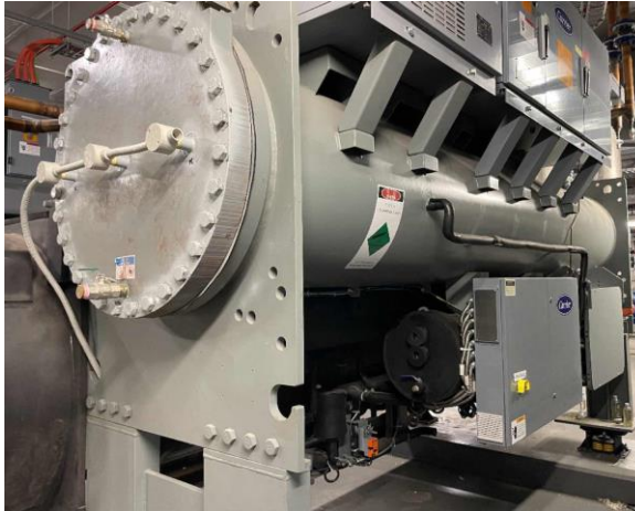
Line ID 36: Internal, Level 6, Chiller Room, Chillers, R1233ZD Refrigerant - Non ODS Refrigerant
