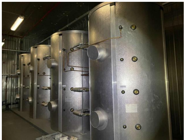
Line ID 29: Internal, Level 6, HWP Room, Large Rheem Hot Water Units, Internal Insulation - Suspected SMF
