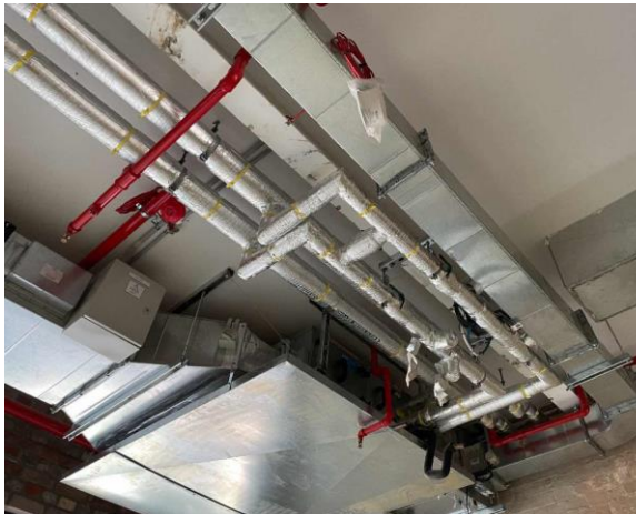
Line ID 20: Internal, Ground Level, Turbot St Heritage Building, Underside of Ceiling, Pipework, Insulation Material - Suspected SMF
