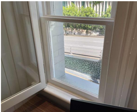
Line ID 11: Internal, Level 1, Turbot St Heritage Building, Throughout, Original Window Frames, White Paint - Lead Detected (13% w/w)
