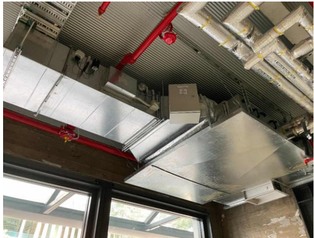
Line ID 19: Internal, Ground Level, Turbot St Heritage Building, Underside of Ceiling, Air Conditioning Ductwork, Insulation Material - Suspected SMF
