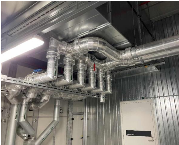
Line ID 24: Internal, Level 15, Plant Room, Pipework, Insulation Material - Suspected SMF
