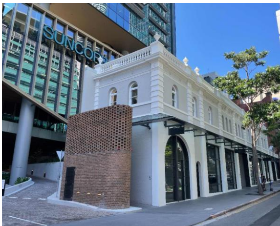
Line ID 6: External, Ground Level and Level 1, Turbot St Heritage Building, Throughout Perimeter, Walls, Beige Paint - Lead Detected (0.072% w/w)
