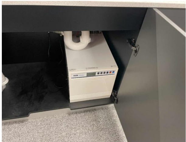
Line ID 33: Internal, Level B1, Security Room Adjacent Entrance Driveway, Below Sink, Zip Boiler, Internal Insulation - Suspected SMF
