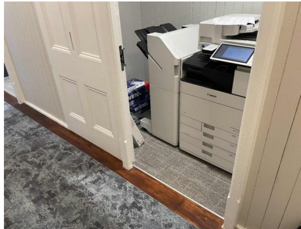
Line ID 10: Internal, Level 1, Turbot St Heritage Building, Throughout, Original Timberwork, White Paint - Lead Detected (4.5% w/w)
