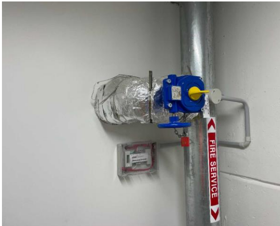
Line ID 18: Internal, All Levels, Stairwells, Hydrant Pipework, Insulation Material - Suspected SMF
