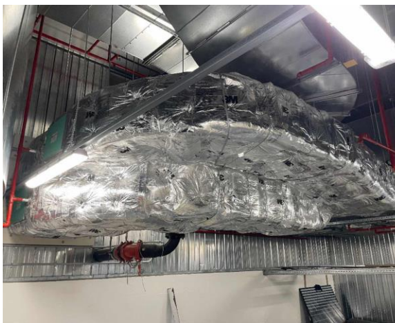
Line ID 22: Internal, Level 15, Plant Room, Air Conditioning Ductwork, Insulation Material - Suspected SMF
