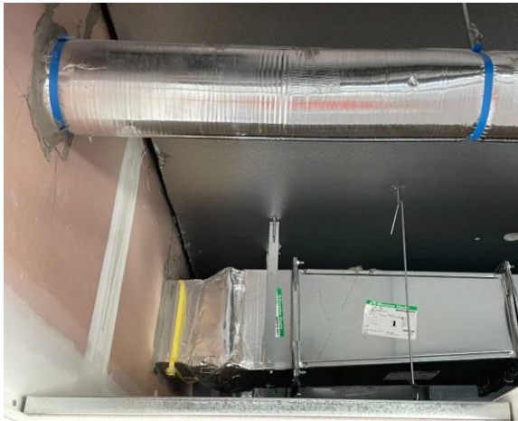
Line ID 14.1: Internal, All Levels, Office Areas, Ceiling Space, Ductwork and Pipework, Insulation Material - Suspected SMF
