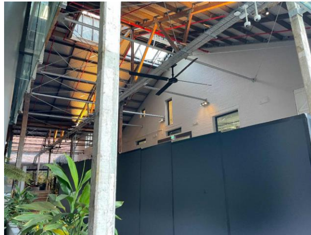
Line ID 5: External, Ground Level, Turbot St Heritage Building, Eastern Undercover Area, Timberwork, White Paint - Lead Detected (3.4% w/w)
