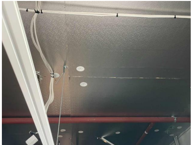
Line ID 15: Internal, All Levels, Office Areas, Ceiling Space, Lining, Insulation Material - Suspected SMF
