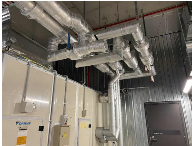
Line ID 31: Internal, Level 6, Plant Room Throughout, Pipework, Insulation Material - Suspected SMF
