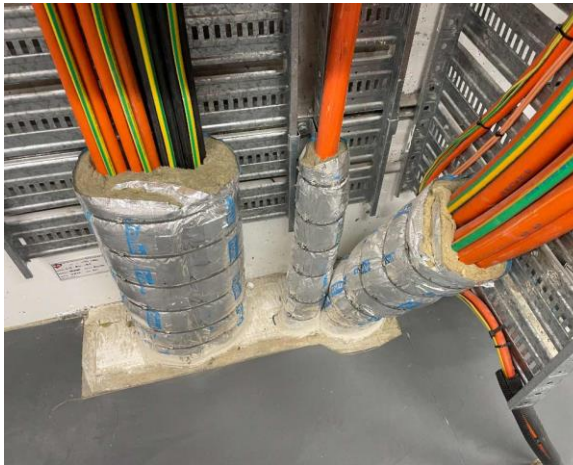
Line ID 13: Internal, All Levels, Electrical Room Throughout, Cable Conduits, Insulation Material - Suspected SMF
