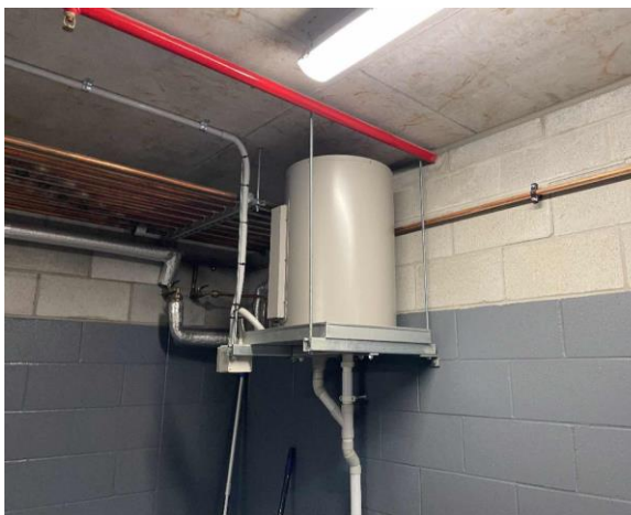
Line ID 34: Internal, Level B1, Waste Room, South Side, Hot Water Heater, Internal Insulation - Suspected SMF
