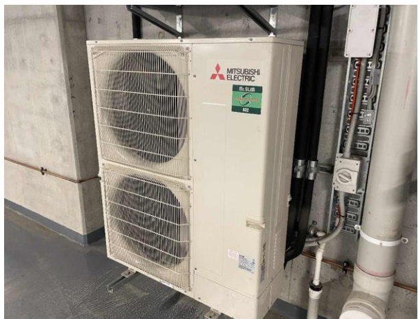
Line ID 35: Internal, All Levels, Plant Areas, Various Areas, Air Conditioning Units, R32 Refrigerant - Non ODS Refrigerant
