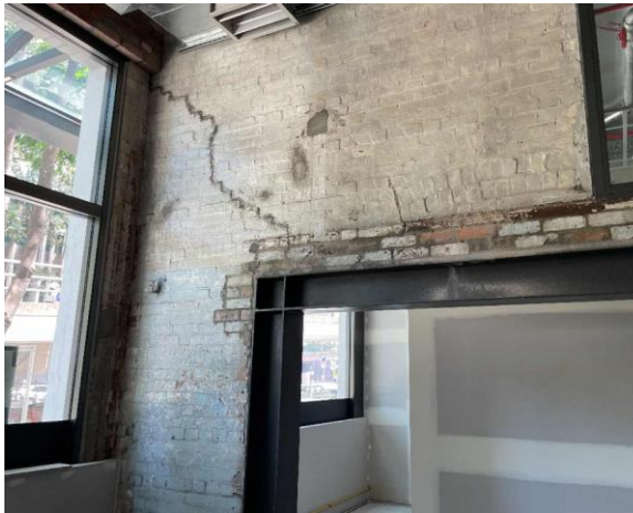
Line ID 7: Internal, Ground Level, Turbot St Heritage Building, North Tenancy, Walls, Green Paint - Lead Detected (0.15% w/w)
