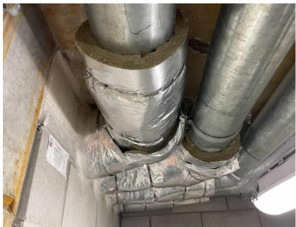
Line ID 17: Internal, All Levels, Service Areas and Risers Throughout, Pipework, Insulation Material - Suspected SMF
