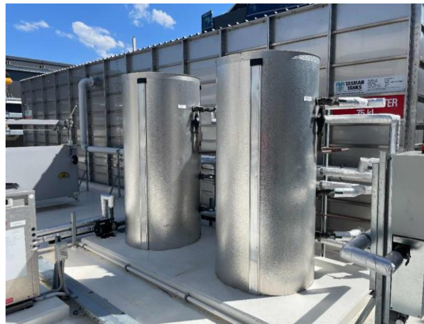
Line ID 12: External, Level 32, Roof Plant Area, Adjacent to Water Tank, Hot Water Units, Internal Insulation - Suspected SMF
