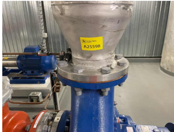
Line ID 3: Internal, Level 6, Chiller Room, to Chilled Water Pump Pipework, Gasket Material - No Asbestos Detected
