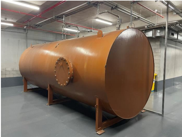
Photo 01. Level B2, Diesel Tank Room (large tank) – fuel tank.
