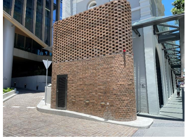
Photo 08. Exterior, Lower Ground Level, Turbot Street driveway – exhaust plenum.
