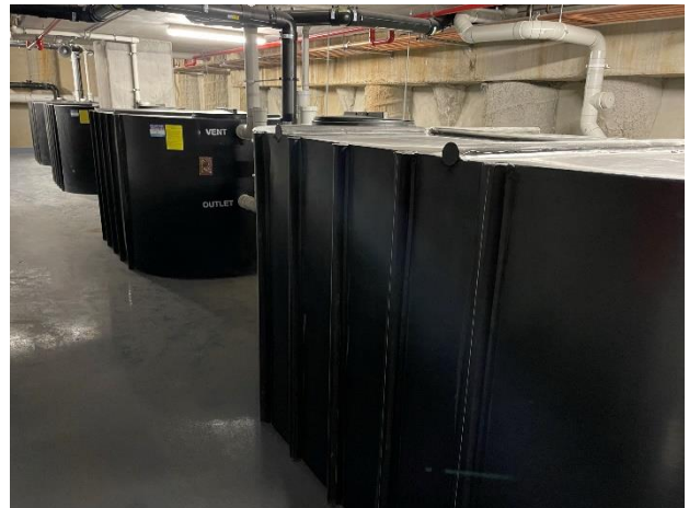
Photo 06. Level B1, Grease Arrestor Room – grease traps.
