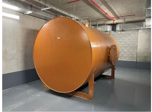
Photo 02. Level B2, Diesel Tank Room (small tank) – fuel tank.
