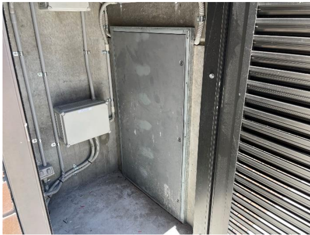
Photo 09. Exterior, Lower Ground Level, Turbot Street driveway – exhaust plenum hatch.
