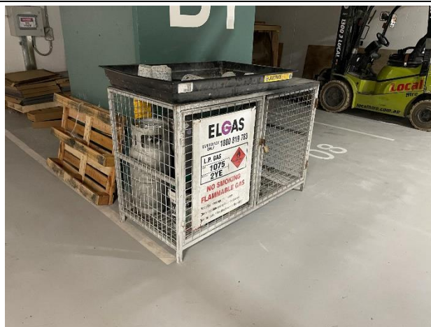
Photo 06. LPG cage in Loading Dock.
