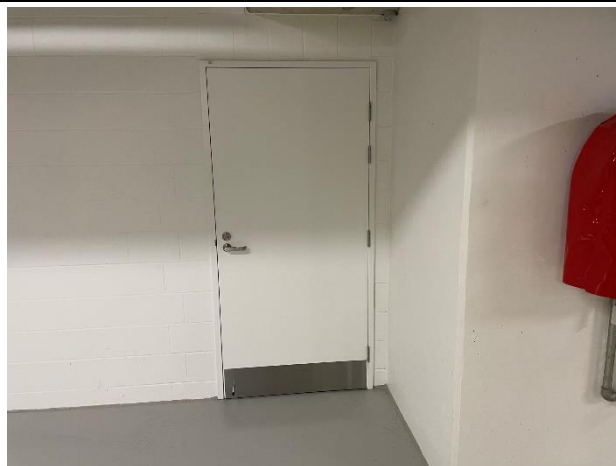
Photo 02. No COMBUSTIBLE LIQUID placard at entrance to Diesel Tank Room.
