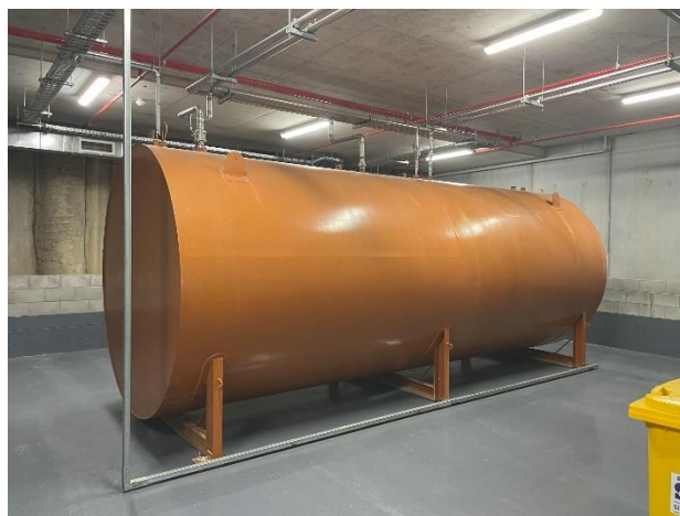
Photo 04. Diesel tanks in Diesel Tank Room.
