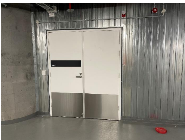
Photo 03. No Class 2.2 placard at entrance to Chiller Room.
