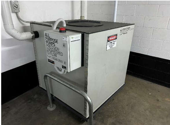
Photo 19. B, Carpark, adjacent northern stairs, sewer pump pit.
