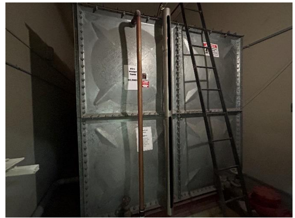
Photo 28. L34, North side, Water Tank Room, fire water tank.
