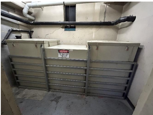
Photo 17. B, Grease Trap Room 1, grease trap.
