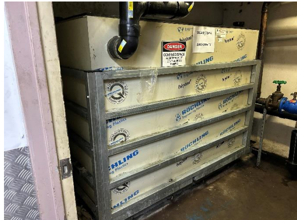
Photo 18. B, Grease Trap Room 2, grease trap.
