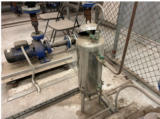
Photo 07. Unlabelled dosing pot in L34 Tenant Plant Room.
