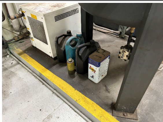
Photo 06. Chemicals not provided with secondary spill containment in Chiller Room. Unlabelled container.
