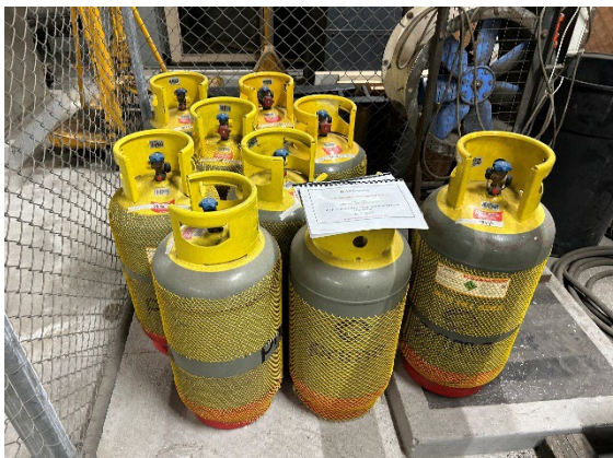
Photo 09. Unsecured recovered refrigeration gas cylinders in Chiller Room.
