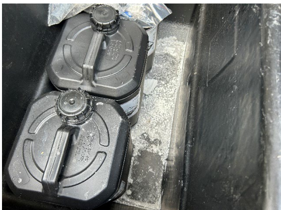
Photo 03. Leaked chemical in secondary container in L34 external cooling tower area.
