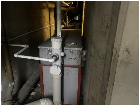
Photo 09. B1, wall cavity between parking bay 5 and 6, grease trap x 2
