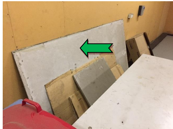
Photo 10 Interior: level 16, plant room, diesel storage area, stored panel – non-asbestos containing fibre cement sheet.
