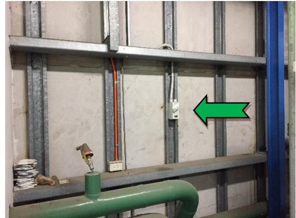
Photo 4 Interior: level 16, plant room, internal walls – non-asbestos containing fibre cement sheet.
