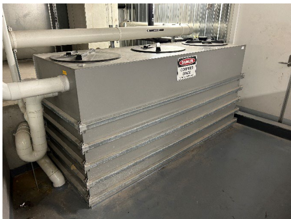
Photo 05. L4, Grease Trap Room, grease trap.
