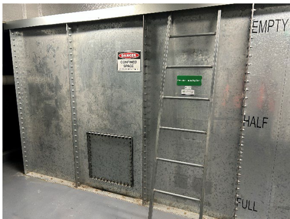
Photo 03. L4, Tank Room, rain water tank.
