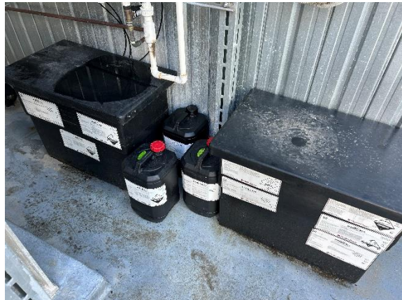
Photo 02. Chemical storage in Level 13 Cooling Tower Area. Chemical containers stored without secondary containment.
