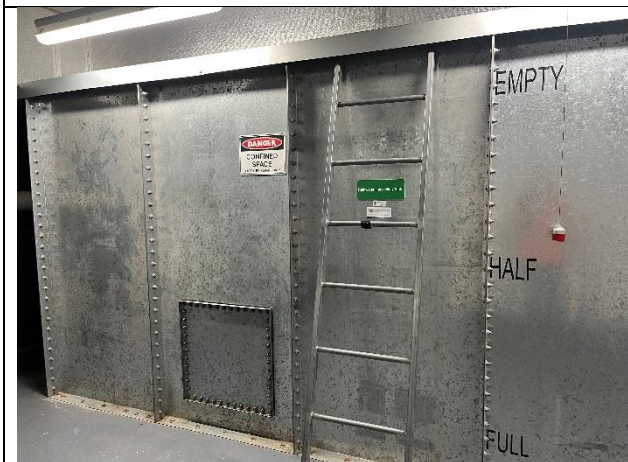
Photo 03. L4, Tank Room, rain water tank.
