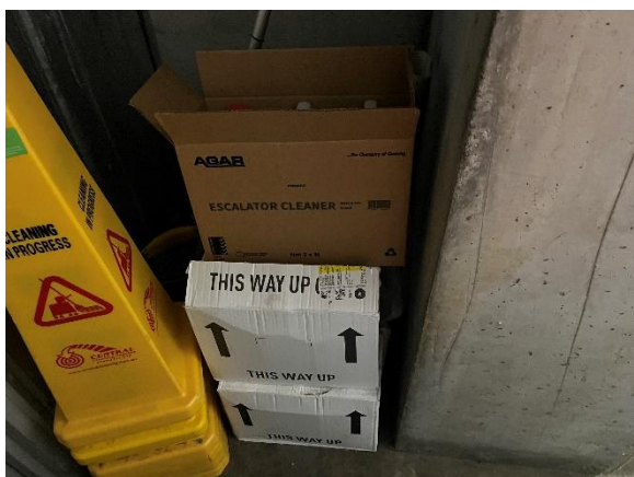
Photo 05. Chemical storage in Level 3 Cleaners Store Room. Chemicals not stored within secondary containment.
