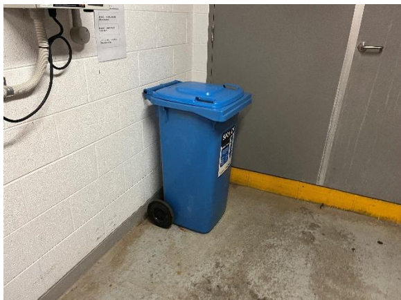
Photo 01. Spill kit in Fire Pump Room.
