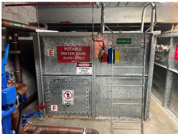
Photo 05. L3, Water Tank Room, adjacent Store Room 7, potable water tank.
