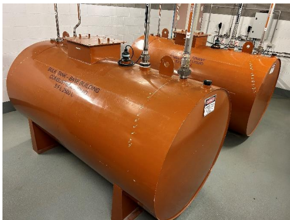
Photo 03. L3, Diesel Tank Room, base building and tenant tanks.
