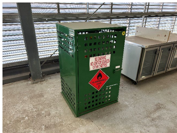
Photo 03. LPG storage in Level 12 Plant Room.
