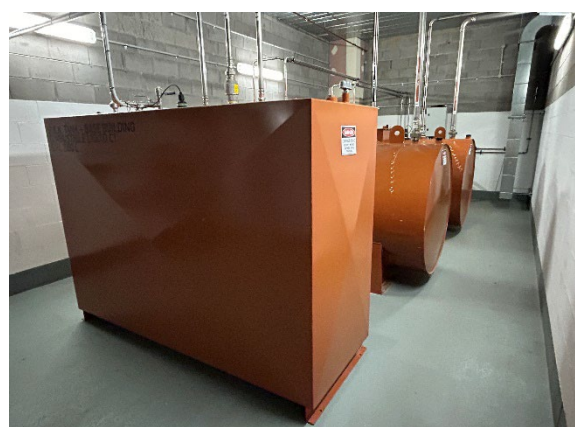
Photo 06. Diesel tanks.
