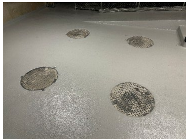
Photo 06. Ground, Retail Garbage Room, 4 x sewer pits
