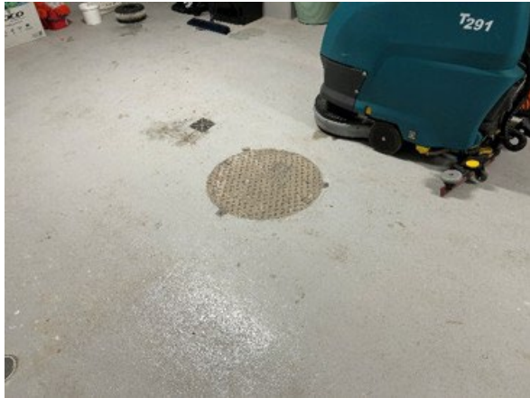
Photo 07. Ground, Refuse and Cleaners Room, 1 x sewer pit
