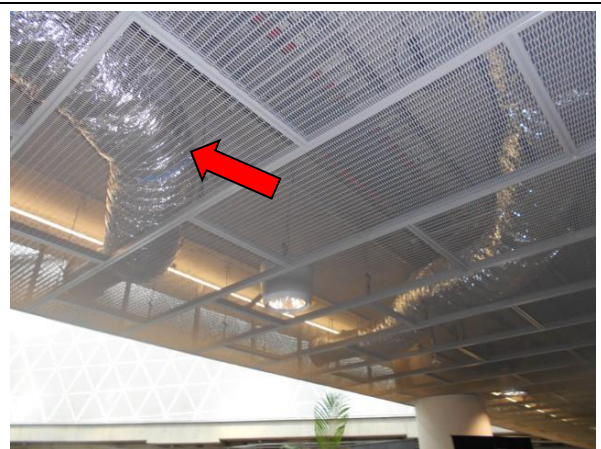
Photo 9: Office Levels, Ceiling Space– SMF to flexible ductwork insulation
