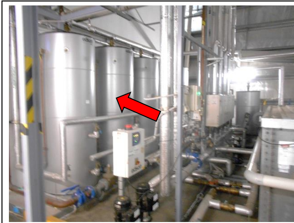
Photo 6: Level 15, Plant Room– SMF internal insulation to hot water units
