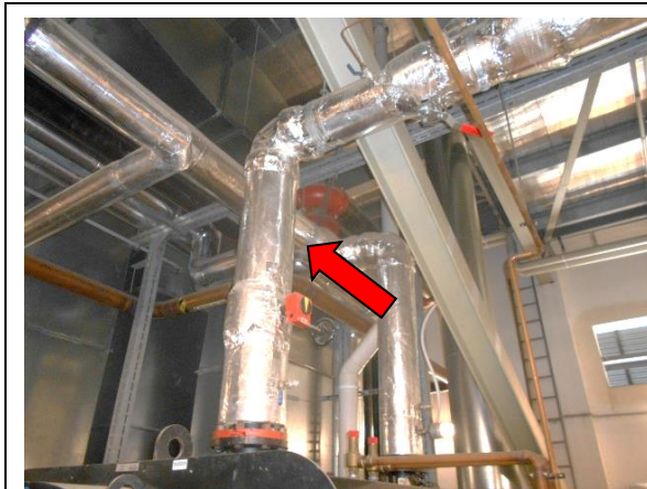
Photo 4: Roof Level, Boiler Room – SMF to pipework insulation
