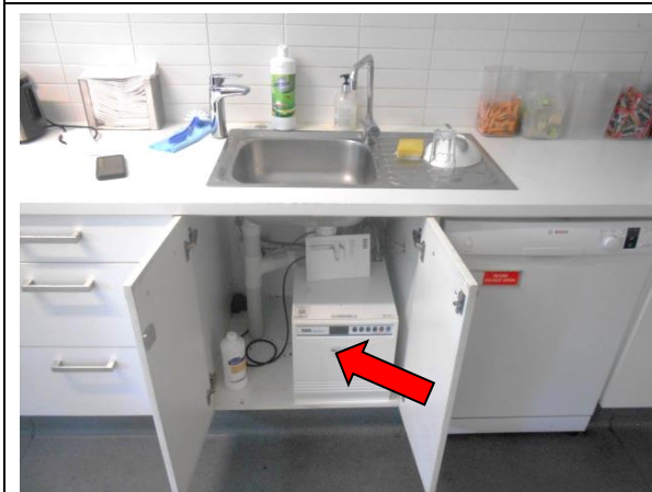
Photo 8: Office Levels, Kitchenettes– SMF internal insulation to hot water units
