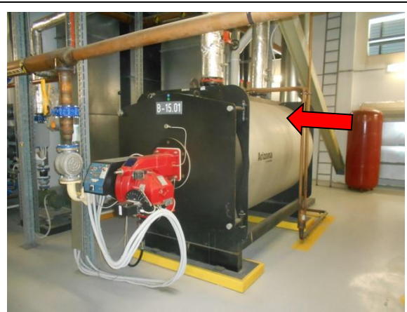
Photo 5: Roof Level, Boiler Room – SMF to internal areas of boiler
