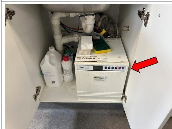
Photo 9: Office Levels, Kitchenettes- SMF internal insulation to hot water units
