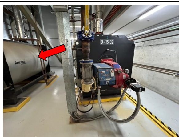
Photo 6: Roof Level, Boiler Room – SMF to internal areas of boiler
