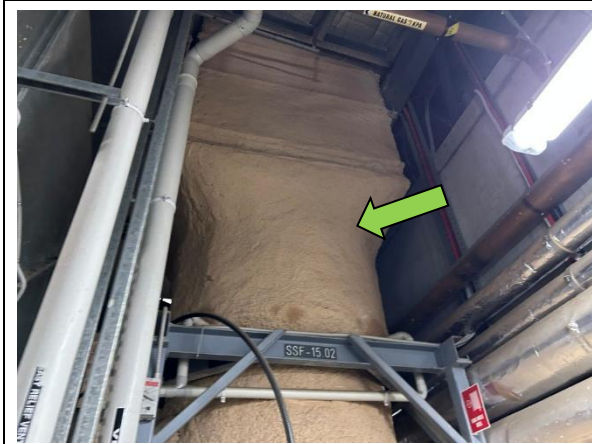
Photo 3 & 4: Level 15, Plant Room, Ductwork, Sprayed Insulation – Non-asbestos insulation material
