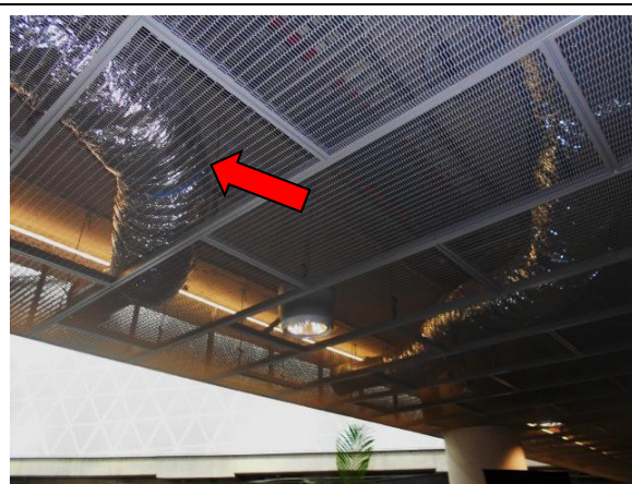
Photo 10: Office Levels, Ceiling Space- SMF to flexible ductwork insulation
