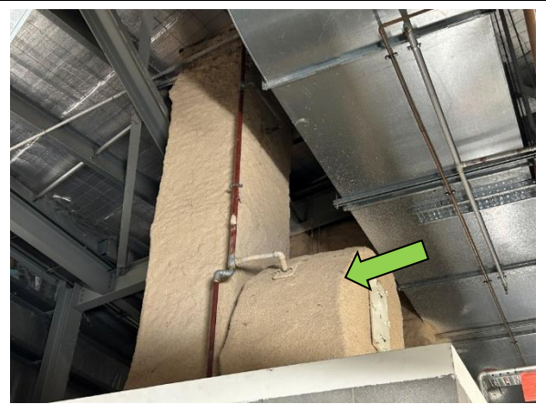
Photo 3 & 4: Level 15, Plant Room, Ductwork, Sprayed Insulation – Non-asbestos insulation material
