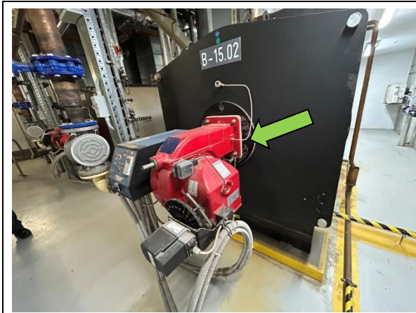
Photo 1: Level 15, Plant Room, Boiler Room, Motor to Boiler – Non-asbestos containing gaskets
