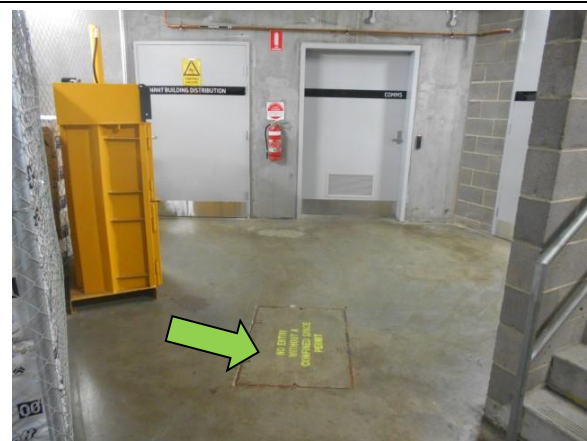
Storm water pit in on Level P2 is secured & appropriately signposted
