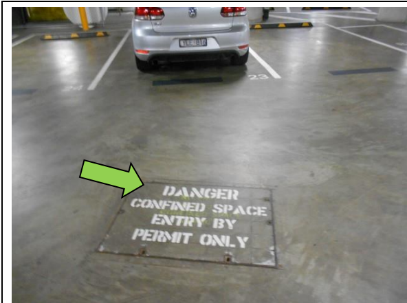
Storm water pit in on Level P1 is secured & appropriately signposted
