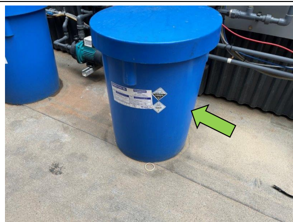
Appropriate secondary containment (bunding) for the cooling tower chemicals
