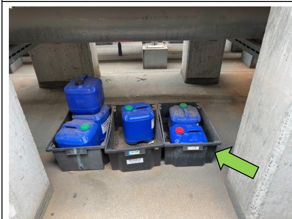
Appropriate secondary containment (bunding) for the cooling tower chemicals
