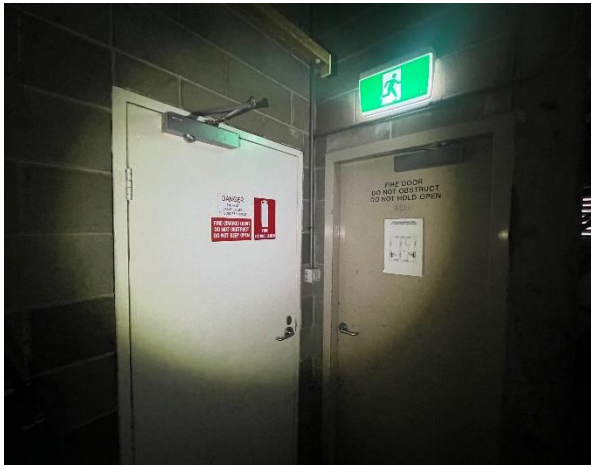
Line ID 94.3: Internal, L2-3, L5-13 and 15-21, Lift Lobby and Electrical Service Room, Fire Entry Door, Fire Door Core - Suspected Asbestos
