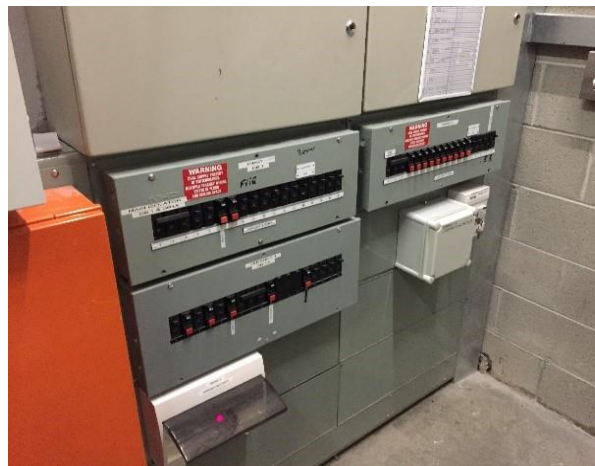
Line ID 68: Internal, L21, Plant Room, Electrical Services Cupboard, Arc Shields - Suspected Asbestos
