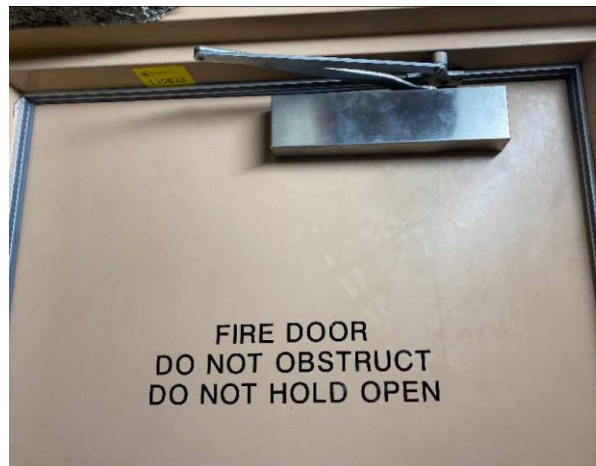
Line ID 110: Internal, L14, Plant Room, Fire Doors Throughout, Brown (Light) Paint - Lead Detected (0.15% w/w)
