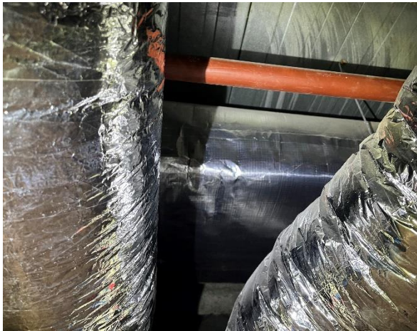
Line ID 160: Internal, L2-3, L5-13 and 15-21, Lift Lobby and Electrical Service Room, Rigid and Flexible Ductwork, Insulation Material - Suspected SMF
