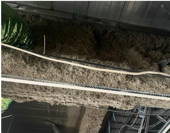
Line ID 65.1: Internal, L20, Main Office Areas, Throughout the Underside of the Ceiling to Concrete Columns, Sprayed Vermiculite - No Asbestos Detected
