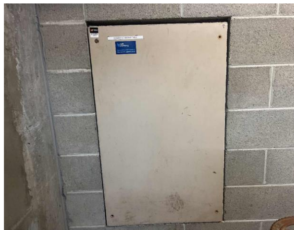
Line ID 70: Internal, L22, Plant Room, Hatch Door to Domestic Water Tank, Vermiculite - No Asbestos Detected
