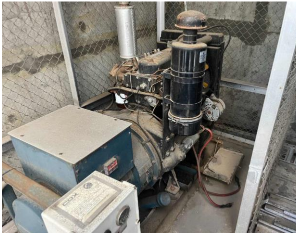
Line ID 1: External, Roof, East Plant Area, Generator or Motor for Motorised Basket, Gaskets - Suspected Asbestos
