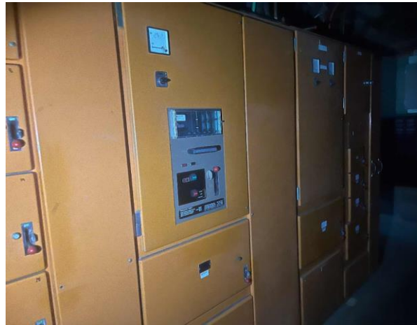
Line ID 88: Internal, L23, Plant Room, Within Electrical Cupboards, HRC Fuses - Suspected Asbestos
