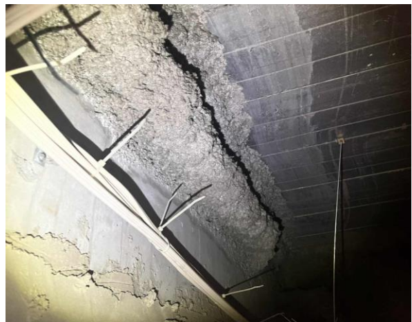
Line ID 65: Internal, L20, Main Office Areas, Throughout the Underside of the Ceiling to Concrete Columns, Sprayed Vermiculite - No Asbestos Detected
