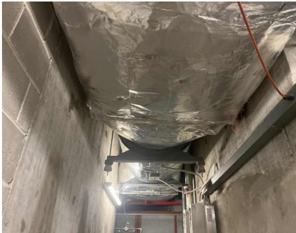
Line ID 155: Internal, L23, South Air Handling Unit AHU-7, Ductwork Foil Lined Insulation, Insulation Material - Suspected SMF
