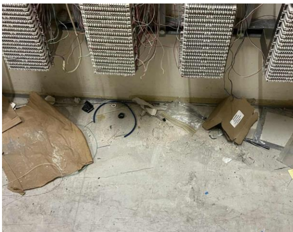
Line ID 12: Internal, B2, MDF Room, To Ledges and Floor Below Penetration to Floor Above, Vermiculite Debris - No Asbestos Detected
