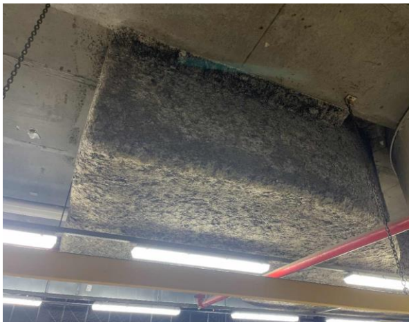
Line ID 17: Internal, GF, Car Park Plant Room, To Large Ductwork, Sprayed Vermiculite - No Asbestos Detected
