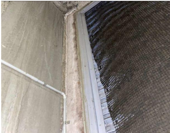
Line ID 123: Internal, GF, External Plant Room, West Ductwork Room Construction Joints, Ceramic Fibre - Suspected SMF
