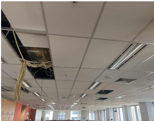
Line ID 164.2: Internal, L2-3, L5-13 and 15-21, Main Office Areas, Throughout Office Areas, Compressed Ceiling Tiles - Suspected SMF
