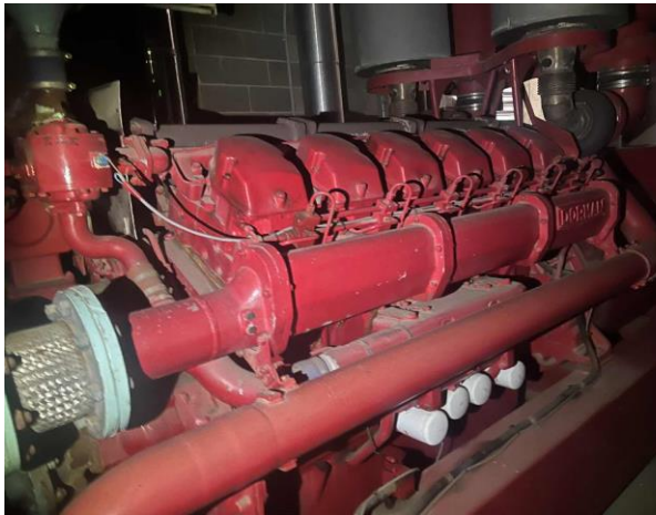
Line ID 114: Internal, L23, Plant Room, To Generator, Red Paint - Lead Detected (1.4% w/w)
