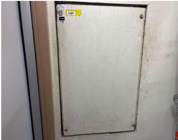
Line ID 52: Internal, L14, Plant Room, Hatch Door to Riser, Vermiculite - No Asbestos Detected
