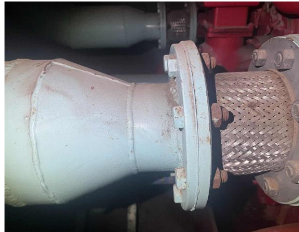
Line ID 84: Internal, L23, Plant Room, Green Pipes to Generator Flange Gaskets, Green Gasket Material - No Asbestos Detected
