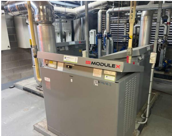
Line ID 147: Internal, L22, Plant Room, Modules Boilers Internals, Insulation Material - Suspected SMF
