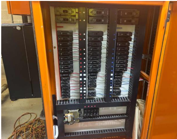
Line ID 76: Internal, L22, Plant Room, Within Electrical Cupboards, HRC Fuses - Suspected Asbestos
