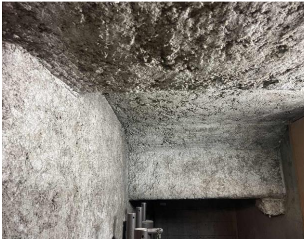
Line ID 139.2: Internal, L14, Plant Room, To Walls, Ductwork and Steel Beams, Sprayed Vermiculite - SMF Detected
