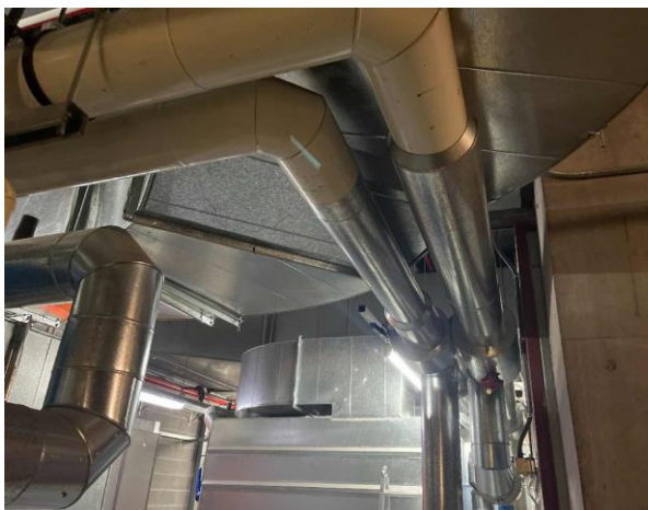
Line ID 119: Internal, GF, External Plant Room, AC Ductwork, Insulation Material - Suspected SMF
