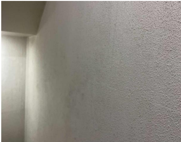
Line ID 93: Internal, L23, South Stairwell, To Concrete Walls, Textured Coating - No Asbestos Detected
