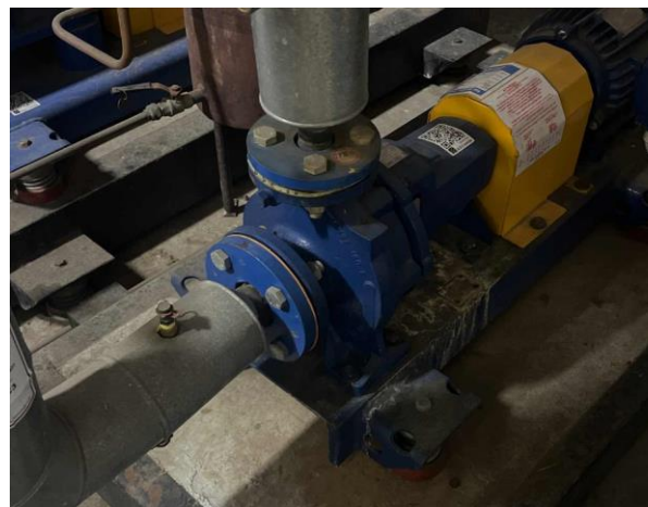
Line ID 75: Internal, L22, Plant Room, To Pipe Work of Pump Machinery, Orange Gasket Material - No Asbestos Detected
