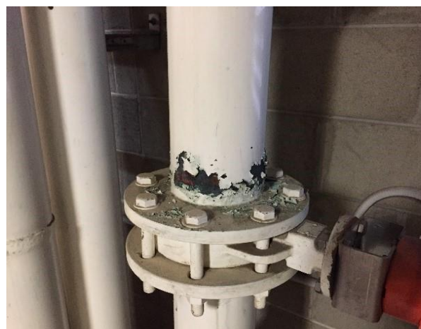
Line ID 113: Internal, L23, Plant Room, Pipe work, White Paint - Lead Detected (0.005% w/w)
