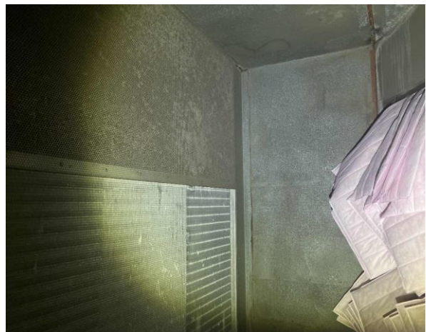
Line ID 154: Internal, L23, South Air Handling Unit AHU-7, AHU-7 Wall Lining, Insulation Material - Suspected SMF
