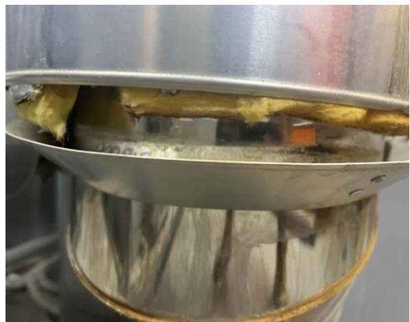
Line ID 144.1: Internal, L22, Plant Room, Exhaust Units from Boilers, Insulation Material - Suspected SMF
