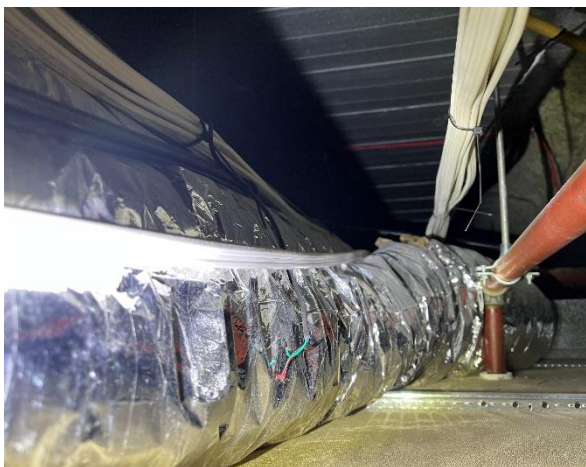
Line ID 160.2: Internal, L2-3, L5-13 and 15-21, Lift Lobby and Electrical Service Room, Rigid and Flexible Ductwork, Insulation Material - Suspected SMF
