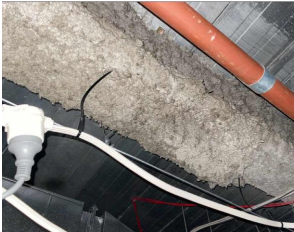
Line ID 101: Internal, L3, Main Office Areas, Throughout the Underside of the Ceiling to Concrete Columns, Sprayed Vermiculite - No Asbestos Detected
