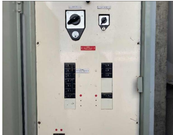
Line ID 2: External, Roof, East Plant Area, Switchboard Adjacent Cooling Tower Tank, HRC Fuses - Suspected Asbestos
