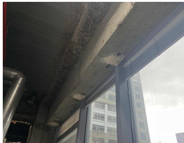
Line ID 54.1: Internal, L14, Plant Room, To Small External Window Frame Supports, Sprayed Vermiculite - No Asbestos Detected
