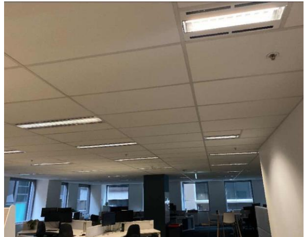
Line ID 164.1: Internal, L2-3, L5-13 and 15-21, Main Office Areas, Throughout Office Areas, Compressed Ceiling Tiles - Suspected SMF
