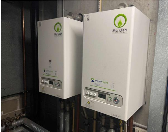
Line ID 145: Internal, L22, Plant Room, Hot Water Units, Insulation Material - Suspected SMF
