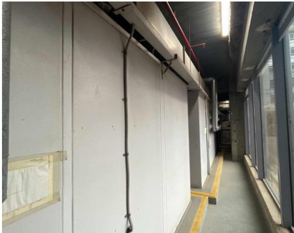
Line ID 131: Internal, L14, Plant Room, Air Handling Unit Wall Lining, Insulation Material - Suspected SMF
