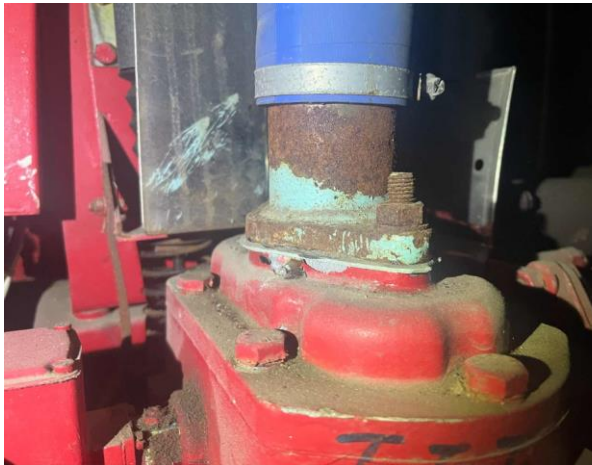
Line ID 87: Internal, L23, Plant Room, Top Flange to Generator, Light Green Gasket Material - No Asbestos Detected
