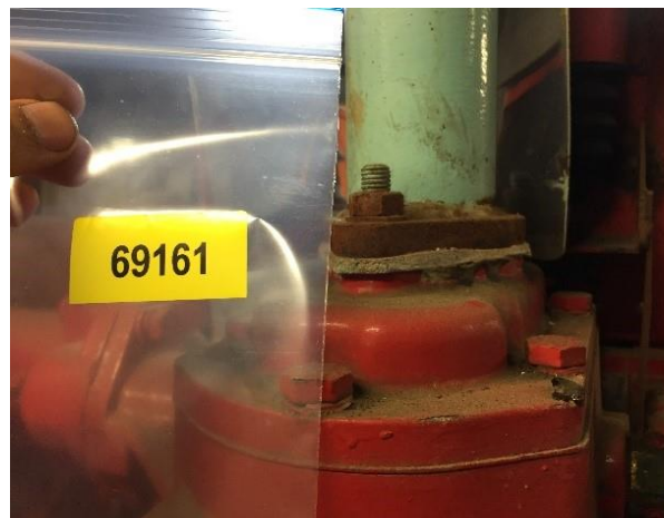
Line ID 86: Internal, L23, Plant Room, To Machinery, Grey Gasket Material - Chrysotile Asbestos Detected
