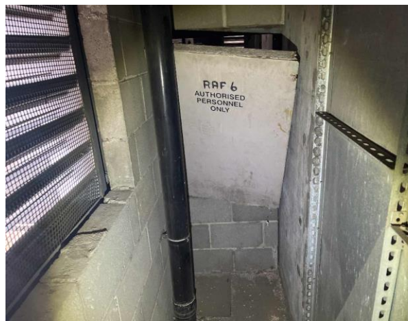
Line ID 90.2: Internal, L23, South Air Handling Unit AHU-7, To Hatch Door Internals to RAF6, Vermiculite - No Asbestos Detected
