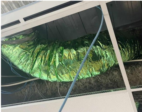
Line ID 163.1: Internal, L2-3, L5-13 and 15-21, Main Office Areas, Flexible Ductwork, Insulation Material - Suspected SMF
