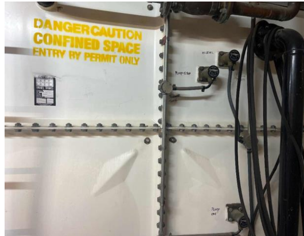
Line ID 72: Internal, L22, Plant Room, To Panels of Water Tank, Mastic Sealant (grey) - No Asbestos Detected
