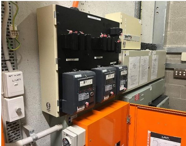
Line ID 95.1: Internal, L2-3, L5-13 and 15-21, Lift Lobby and Electrical Service Room, Grey Switchboards, HRC Fuses - Suspected Asbestos
