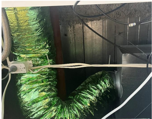
Line ID 165.2: Internal, L2-3, L5-13 and 15-21, Male Toilet, Ceiling Void to Rigid and Flexible Ductwork, Insulation Material - Suspected SMF
