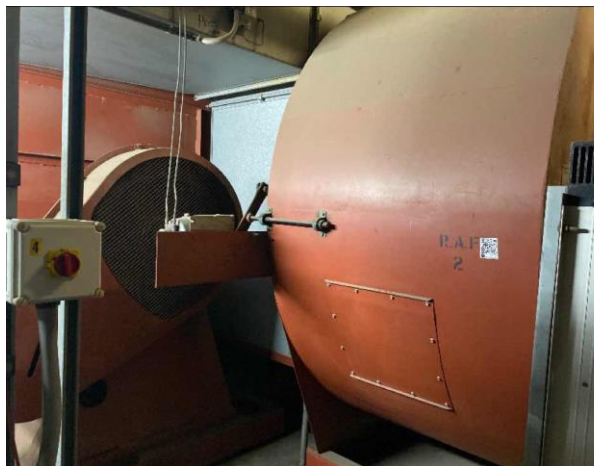
Line ID 111: Internal, L14, Plant Room, Return Air Flow Units, Red (Dark) Paint - Lead Detected (<0.005% w/w)
