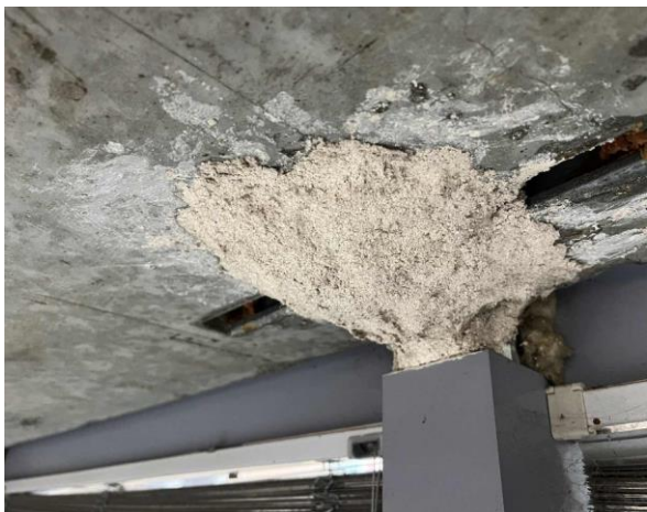
Line ID 54: Internal, L14, Plant Room, To Small External Window Frame Supports, Sprayed Vermiculite - No Asbestos Detected
