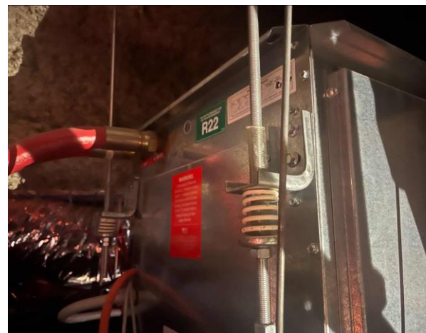
Line ID 174.3: Internal, L2-3, L5-13 and 15-21, Main Office, Ceiling Void Ductwork, R22 Hydrochlorofluorocarbon (HCFC) - ODS Refrigerant
