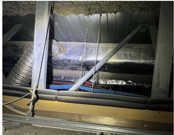
Line ID 163.2: Internal, L2-3, L5-13 and 15-21, Main Office Areas, Flexible Ductwork, Insulation Material - Suspected SMF
