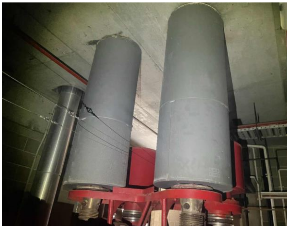
Line ID 151: Internal, L23, Plant Room, Generator Exhausts, External Insulation - Suspected SMF
