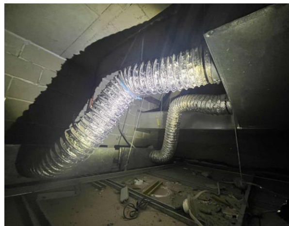
Line ID 158.1: Internal, L2-3, L5-13 and 15-21, Female Toilet, To Rigid and Flexible Ductwork, Insulation Material - Suspected SMF
