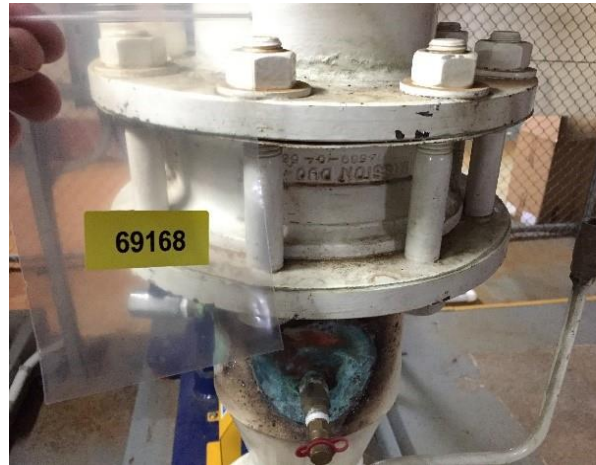
Line ID 11: Internal, B1, Plant Room, Gaskets to Pump Machinery, Green Gasket Material - No Asbestos Detected
