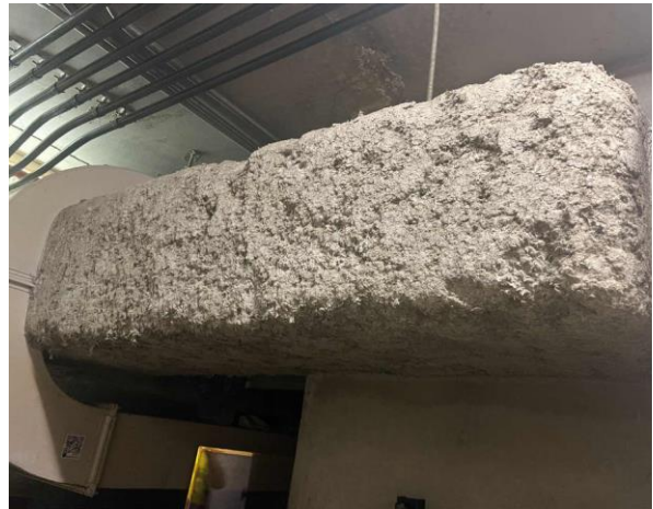
Line ID 14: Internal, B2, Store Room Adjacent Lift Lobby, To Small Ductwork, Sprayed Vermiculite - No Asbestos Detected
