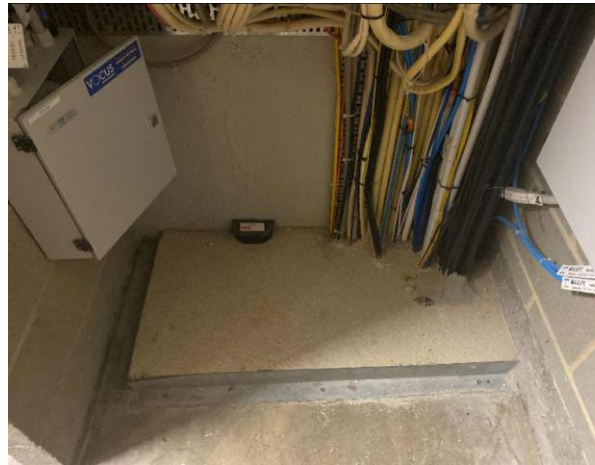
Line ID 32: Internal, L10, Lift Lobby Electrical Services Room, Fire Stop to Penetrations, Vermiculite - No Asbestos Detected
