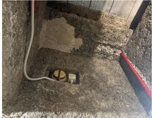
Line ID 139.1: Internal, L14, Plant Room, To Walls, Ductwork and Steel Beams, Sprayed Vermiculite - SMF Detected
