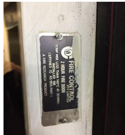
Line ID 56: Internal, L14, Lift Motor Room, Fire Door, Fire Door Core - Suspected Asbestos
