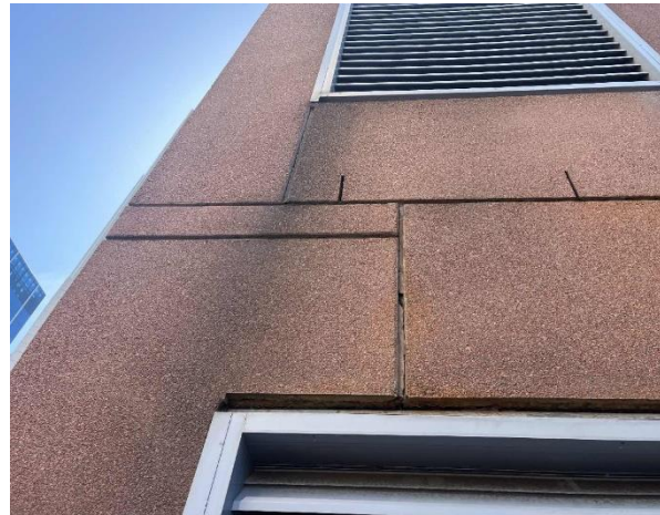
Line ID 6.1: External, Roof, West Plant Area, Expansion Joint Render to Concrete Wall Panels, Render - Chrysotile Asbestos Detected
