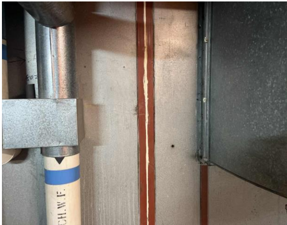
Line ID 47: Internal, L14, Plant Room, Air Handling Unit Panel Sealant, Mastic Sealant (Black & Dark Grey) - No Asbestos Detected
