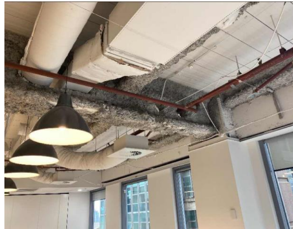
Line ID 104: Internal, L7, Main Office Areas, Fire Rating to Steel Beams in Kitchen and Lunch Area, Sprayed Vermiculite - No Asbestos Detected
