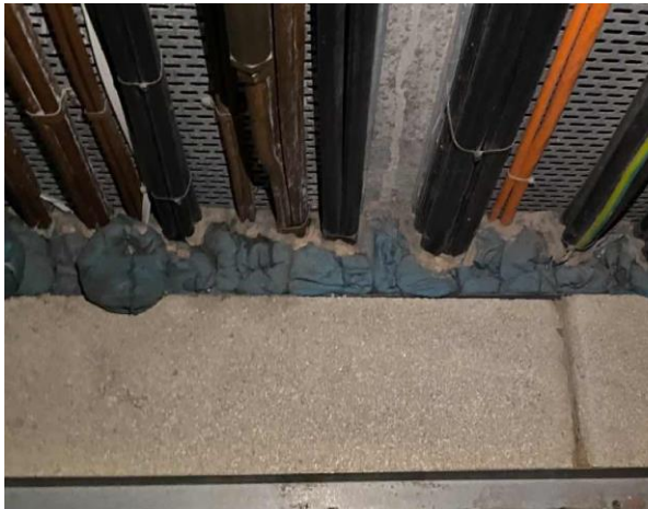
Line ID 161.1: Internal, L2-3, L5-13 and 15-21, Lift Lobby and Electrical Service Room, To Cable Penetrations, Pillow Insulation - Suspected SMF
