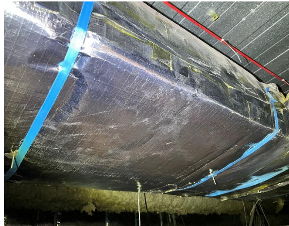
Line ID 162.2: Internal, L2-3, L5-13 and 15-21, Main Office, Rigid Ductwork, Insulation Material - Suspected SMF
