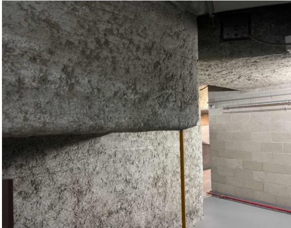
Line ID 139: Internal, L14, Plant Room, To Walls, Ductwork and Steel Beams, Sprayed Vermiculite - SMF Detected
