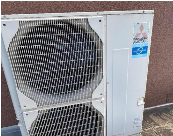
Line ID 168: External, Roof, Throughout, Adjacent Roof Entry Door, R410A Hydrofluorocarbon (HFC) - Non ODS Refrigerant
