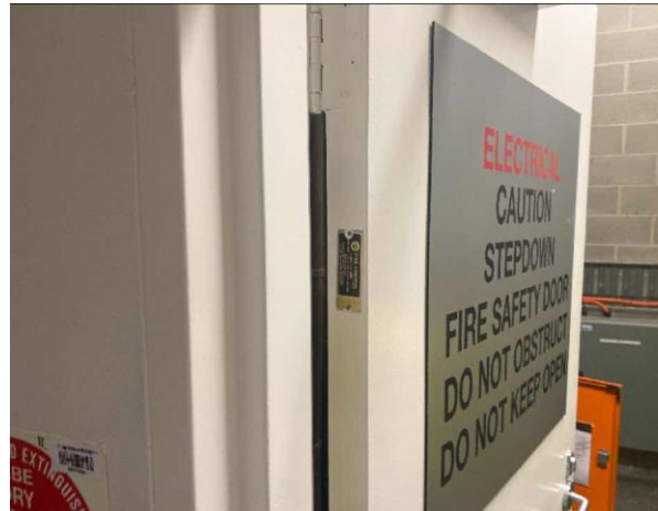
Line ID 94: Internal, L2-3, L5-13 and 15-21, Lift Lobby and Electrical Service Room, Fire Entry Door, Fire Door Core - Suspected Asbestos
