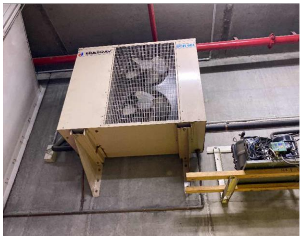
Line ID 171: Internal, GF, Car Park Plant Room, South Wall, Unknown Refrigerant - Suspected ODS
