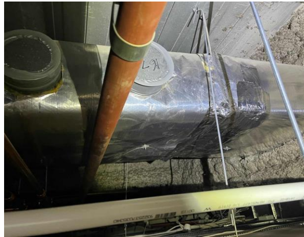
Line ID 66: Internal, L20, Main Office Areas, To Rigid Ductwork, Mastic Sealant (Green) - No Asbestos Detected
