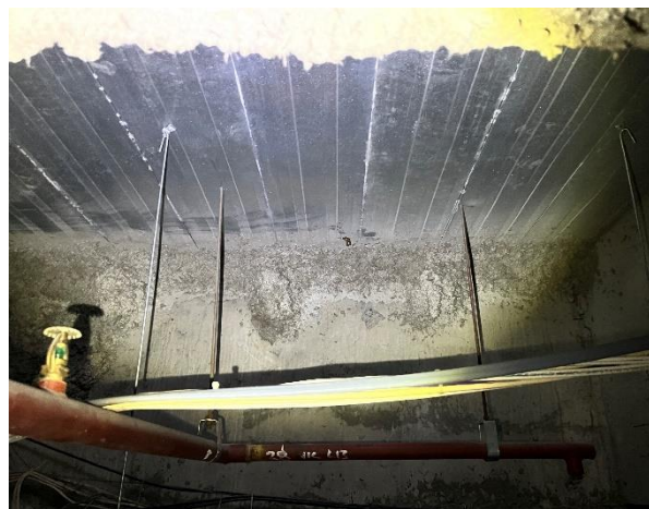
Line ID 35: Internal, L11, Main Office Areas, Throughout the Underside of the Ceiling to Concrete Columns, Sprayed Vermiculite - No Asbestos Detected
