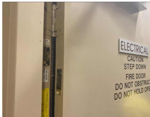
Line ID 94.2: Internal, L2-3, L5-13 and 15-21, Lift Lobby and Electrical Service Room, Fire Entry Door, Fire Door Core - Suspected Asbestos
