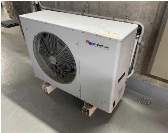
Line ID 172: Internal, L14, Plant Room, East Of Entry Door, R410A Hydrofluorocarbon (HFC) - Non ODS Refrigerant
