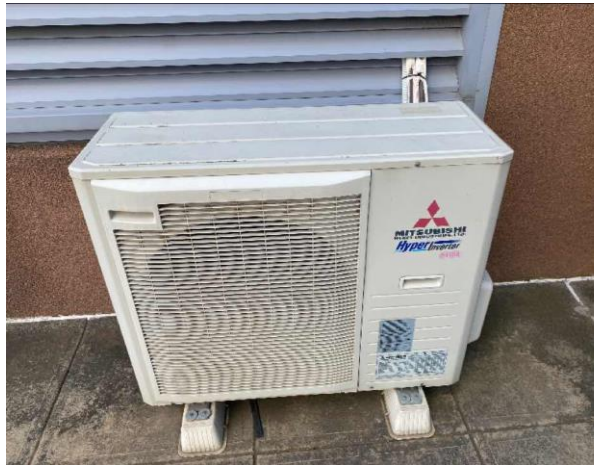
Line ID 169: External, Roof, West Plant Area, West Wall Adjacent Cooling Tower, R410A Hydrofluorocarbon (HFC) - Non ODS Refrigerant
