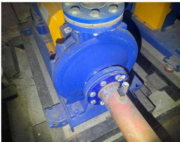
Line ID 74: Internal, L22, Plant Room, To Pipe Work of Pump Machinery, Green Gasket Material - No Asbestos Detected
