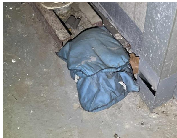
Line ID 149: Internal, L22, Plant Room, To Floor Slab Penetrations, Pillow Insulation - Suspected SMF
