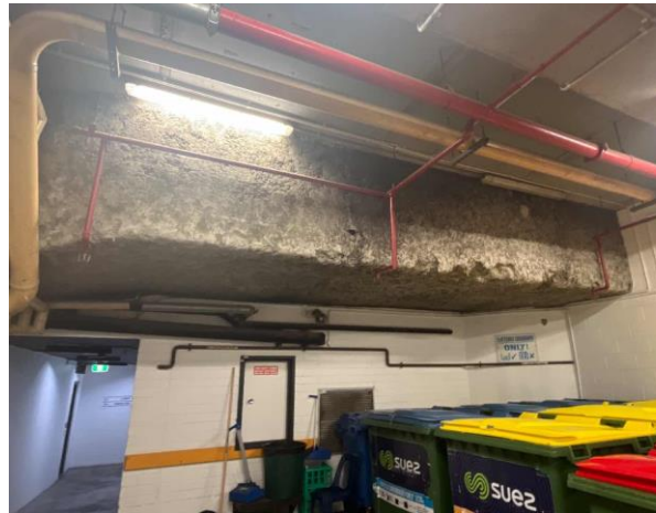
Line ID 30: Internal, GF, Loading Dock, To High Level Ceiling and Ductwork, Sprayed Vermiculite - No Asbestos Detected
