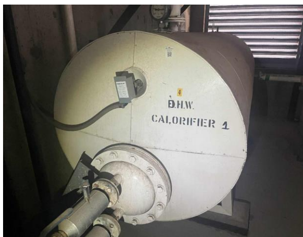
Line ID 112: Internal, L23, Plant Room, Calorifier Metal Casing, Cream Paint - Lead Detected (0.071% w/w)
