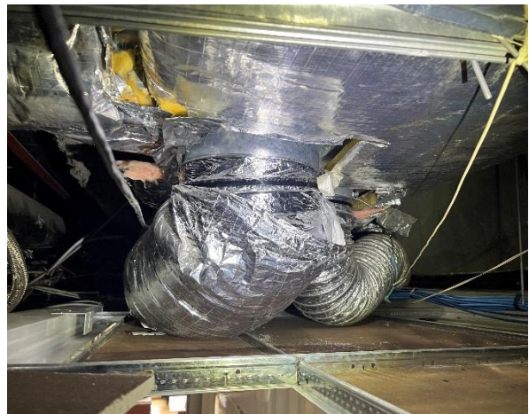
Line ID 165: Internal, L2-3, L5-13 and 15-21, Male Toilet, Ceiling Void to Rigid and Flexible Ductwork, Insulation Material - Suspected SMF
