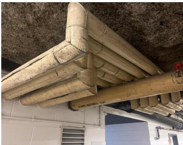
Line ID 125: Internal, GF, Loading Dock, High Level Pipes, Insulation Material - Suspected SMF
