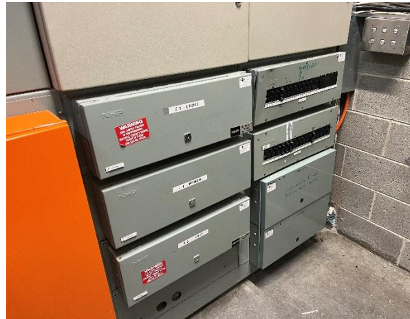
Line ID 95.2: Internal, L2-3, L5-13 and 15-21, Lift Lobby and Electrical Service Room, Grey Switchboards, HRC Fuses - Suspected Asbestos
