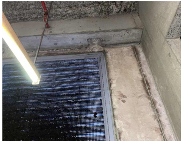
Line ID 124: Internal, GF, External Plant Room, West Ductwork Room Window Frames, Insulation Material - Suspected SMF
