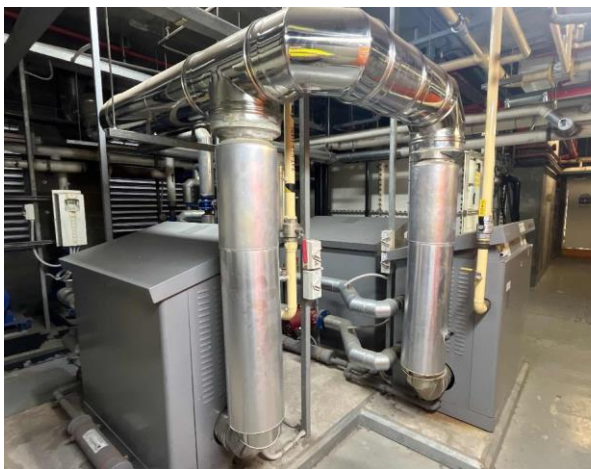
Line ID 144: Internal, L22, Plant Room, Exhaust Units from Boilers, Insulation Material - Suspected SMF
