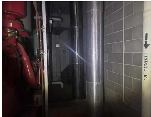
Line ID 152: Internal, L23, Plant Room, Large Diameter Pipes Behind the Generator, Insulation Material - Suspected SMF
