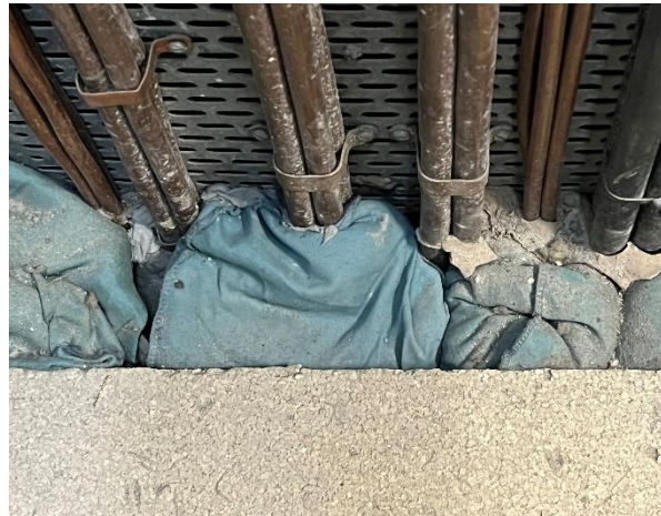
Line ID 99: Internal, L2-3, L5-L13, L15-19 and L21, Lift Lobby Electrical Services Room, Fire Stop to Penetrations, Vermiculite - No Asbestos Detected
