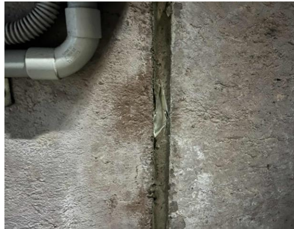
Line ID 132: Internal, L14, Plant Room, Behind Grey Mastic Expansion Joint, Ceramic Fibre - Suspected SMF
