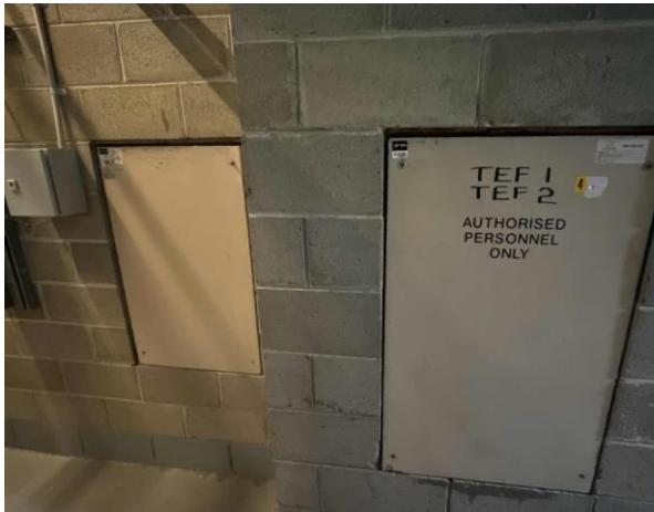
Line ID 71: Internal, L22, Plant Room, Hatch Door to TEF 1 & 2 & Relief Air, Vermiculite - No Asbestos Detected
