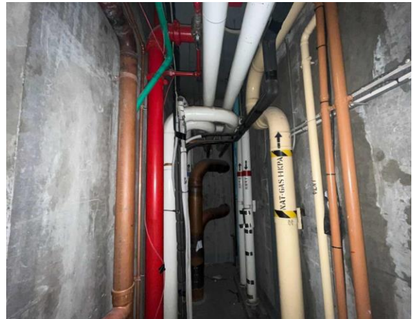
Line ID 148: Internal, L22, Plant Room, Pipe Riser Pipes, Insulation Material - Suspected SMF
