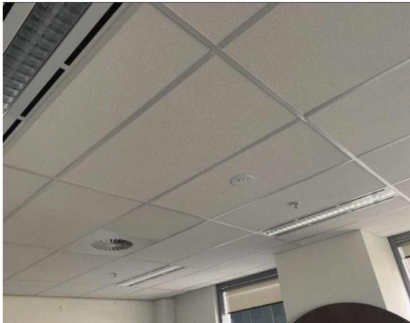
Line ID 164: Internal, L2-3, L5-13 and 15-21, Main Office Areas, Throughout Office Areas, Compressed Ceiling Tiles - Suspected SMF
