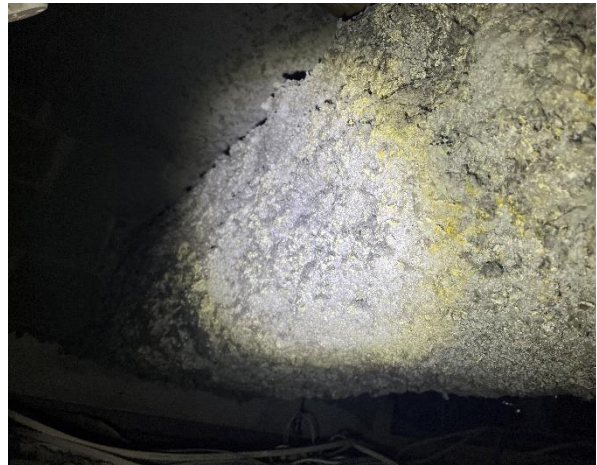
Line ID 37: Internal, L12, Main Office Areas, Throughout the Underside of the Ceiling to Concrete Columns, Sprayed Vermiculite - No Asbestos Detected
