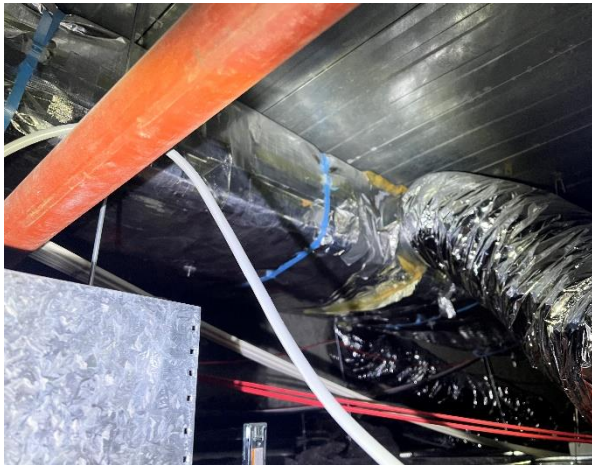
Line ID 165.1: Internal, L2-3, L5-13 and 15-21, Male Toilet, Ceiling Void to Rigid and Flexible Ductwork, Insulation Material - Suspected SMF
