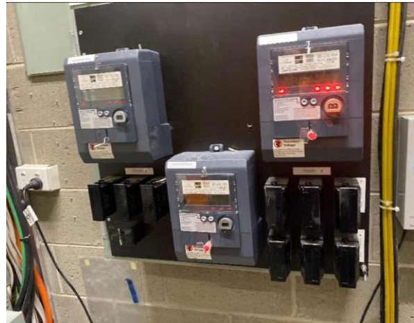
Line ID 102: Internal, L6, Lift Lobby Electrical Services Room, Black Switchboards, HRC Fuses - Suspected Asbestos
