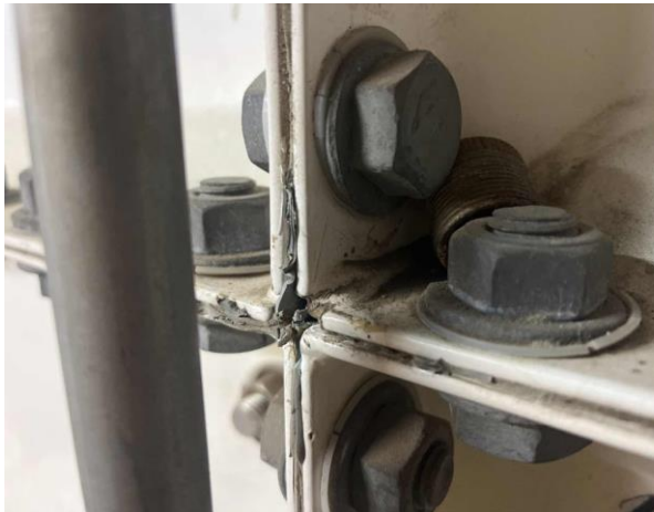
Line ID 72.1: Internal, L22, Plant Room, To Panels of Water Tank, Mastic Sealant (grey) - No Asbestos Detected
