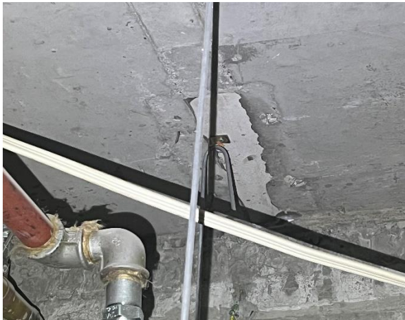
Line ID 63: Internal, L20, Female Toilet, Formwork to the Concrete Soffit within the Ceiling Void, Fibre Cement Sheet - No Asbestos Detected
