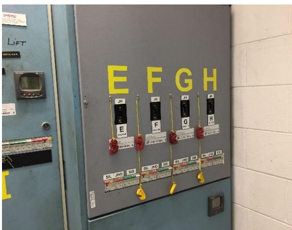
Line ID 79: Internal, L23, Lift Motor Room, Switchboard, Arc Shields - Suspected Asbestos
