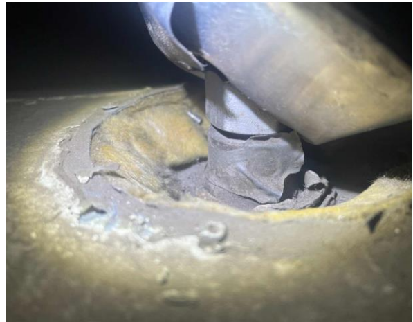
Line ID 150: Internal, L23, Plant Room, Calorifier Insulation, Insulation Material - Suspected SMF
