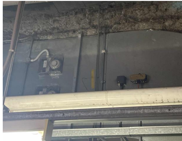
Line ID 27: Internal, GF, External Plant Room, Within AC Ductwork, Heater Bank Insulation - Suspected Asbestos
