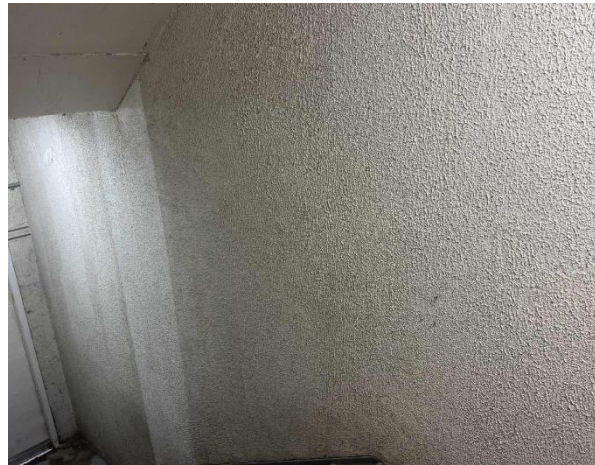
Line ID 22: Internal, GF, External Plant Room, Stairwell to Plant Room, Textured Coating - No Asbestos Detected
