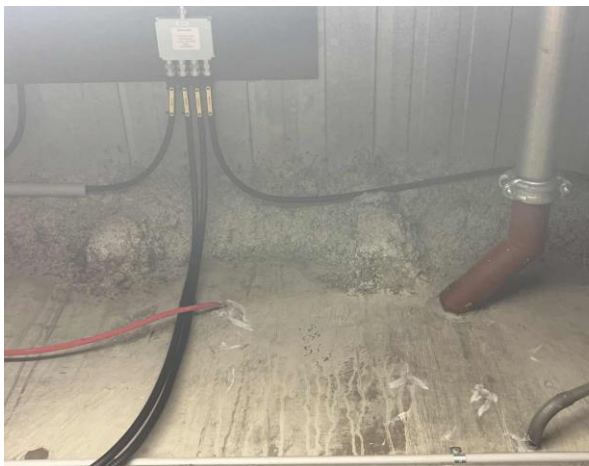
Line ID 55.2: Internal, L14, Plant Room, To Walls, Ductwork and Steel Beams, Sprayed Vermiculite - No Asbestos Detected
