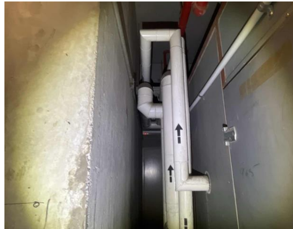
Line ID 156: Internal, L23, South Air Handling Unit AHU-7, Metal Covered Pipes to AHU-7, Insulation Material - Suspected SMF
