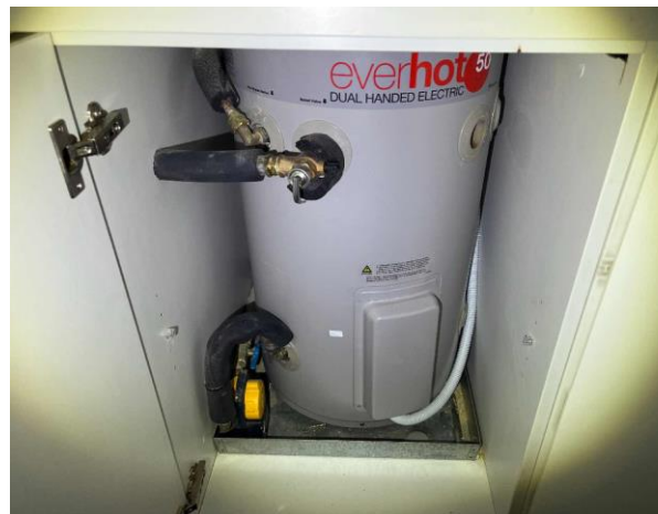
Line ID 157.1: Internal, L2-3, L5-11, L13, and L15-21, Kitchen Area, Hot Water Unit, Insulation Material - Suspected SMF
