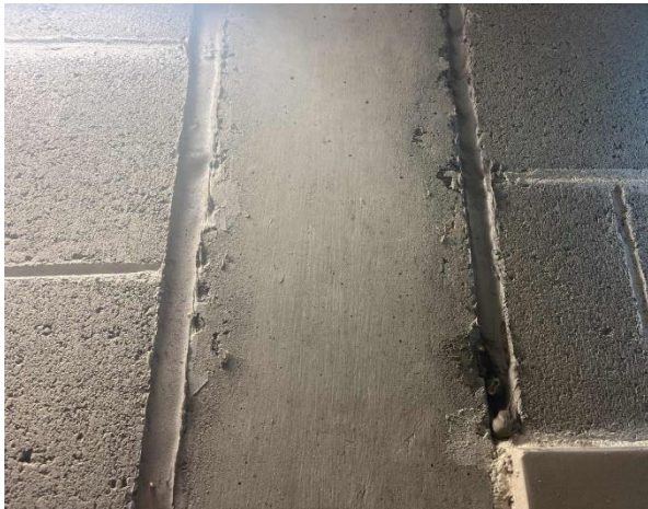
Line ID 89: Internal, L23, South Air Handling Unit AHU-7, Between Brickwork and Concrete, Construction Joint Mastic - No Asbestos Detected
