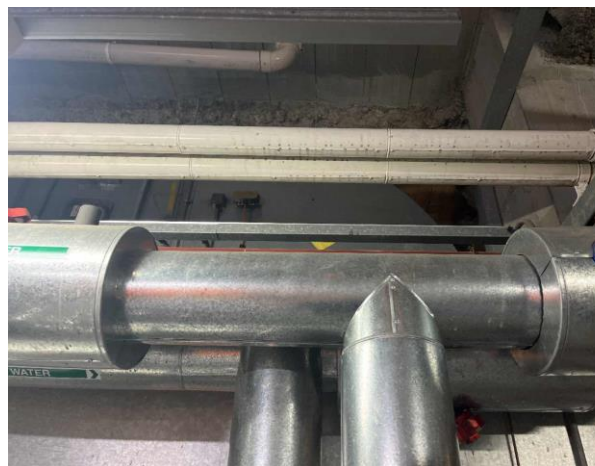
Line ID 120: Internal, GF, External Plant Room, Metal Covered Pipes, Insulation Material - Suspected SMF
