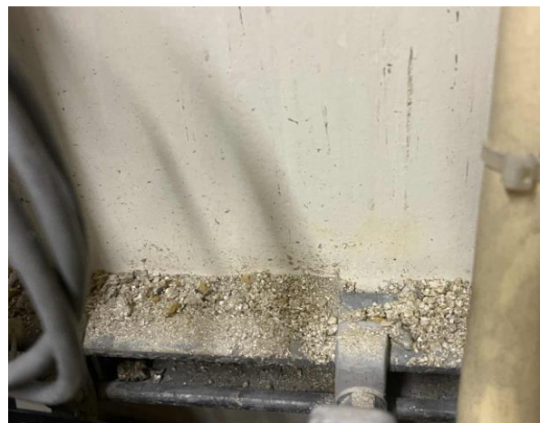
Line ID 12.1: Internal, B2, MDF Room, To Ledges and Floor Below Penetration to Floor Above, Vermiculite Debris - No Asbestos Detected
