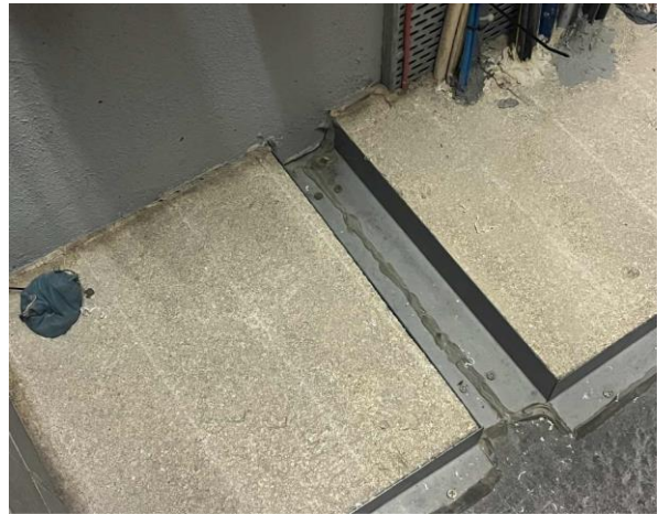
Line ID 64: Internal, L20, Lift Lobby Electrical Services Room, Fire Stop to Penetrations, Vermiculite - No Asbestos Detected
