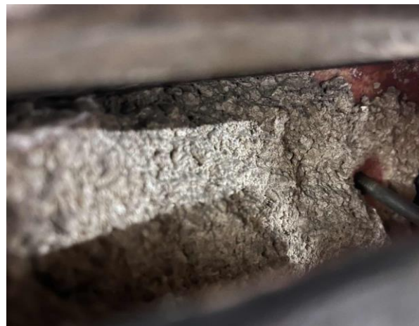
Line ID 28.1: Internal, GF, Loading Dock, Hatch Door to Riser, Vermiculite - No Asbestos Detected
