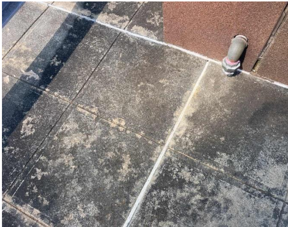
Line ID 7: External, Roof, West Plant Area, White Mastic To Concrete Floor Pavers, Mastic Sealant - No Asbestos Detected
