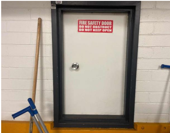
Line ID 29: Internal, GF, Loading Dock, Small Fire Door to Loading Bay, Fire Door Core - Suspected Asbestos
