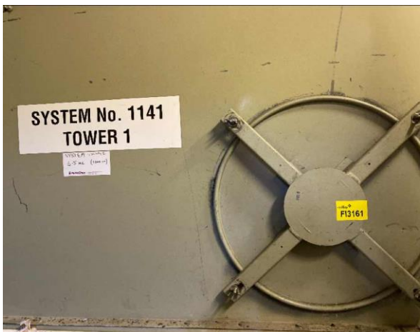
Line ID 107: Internal, GF, External Plant Room, Cooling Tower Tank, Green (Light) Paint - Lead Detected (<0.005% w/w)
