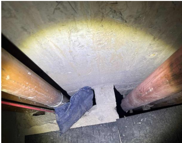
Line ID 36: Internal, L11, Pipe Riser, To Base of Riser, Vermiculite Debris - No Asbestos Detected
