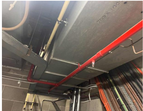
Line ID 143: Internal, L22, Plant Room, AC Ductwork, Insulation Material - Suspected SMF
