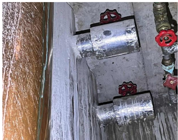
Line ID 128: Internal, L11, Pipe Riser, Pipework Insulation, Insulation Material - Suspected SMF
