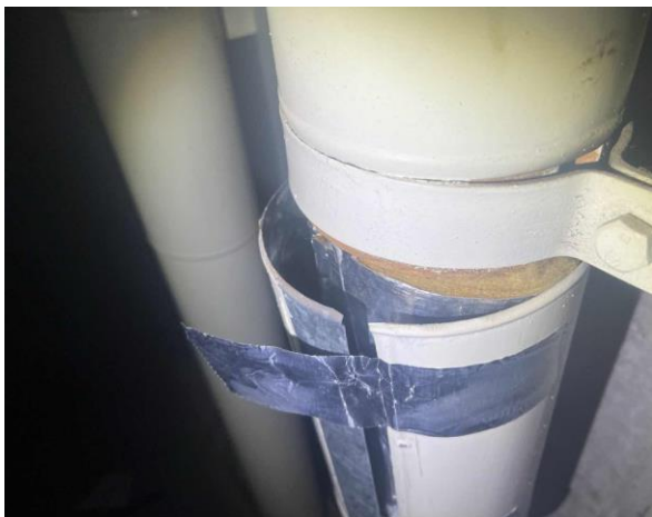
Line ID 148.1: Internal, L22, Plant Room, Pipe Riser Pipes, Insulation Material - Suspected SMF
