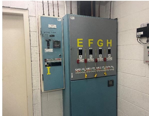
Line ID 95: Internal, L2-3, L5-13 and 15-21, Lift Lobby and Electrical Service Room, Grey Switchboards, HRC Fuses - Suspected Asbestos
