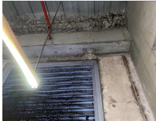
Line ID 25: Internal, GF, External Plant Room, West Ductwork Room Window Grills, To Small External Window Frame Supports, Sprayed Vermiculite - No Asbestos Detected
