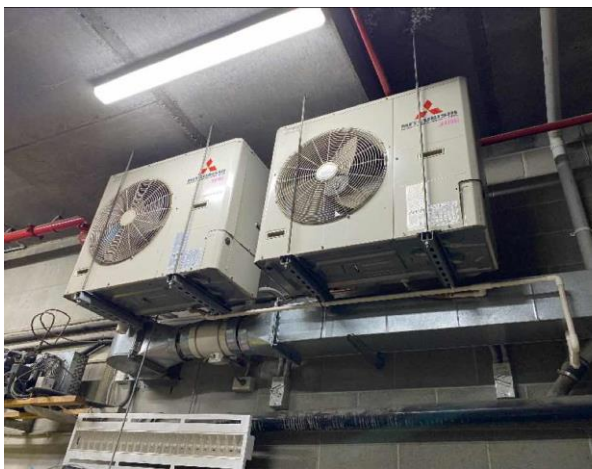
Line ID 170: Internal, GF, Car Park Plant Room, South Wall, R410A Hydrofluorocarbon (HFC) - Non ODS Refrigerant
