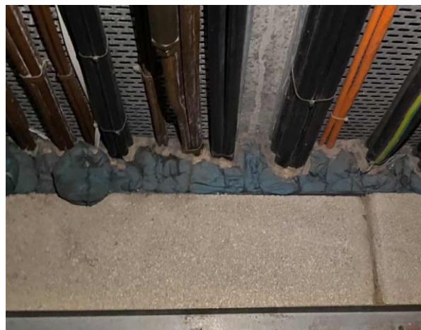
Line ID 99.2: Internal, L2-3, L5-L13, L15-19 and L21, Lift Lobby Electrical Services Room, Fire Stop to Penetrations, Vermiculite - No Asbestos Detected
