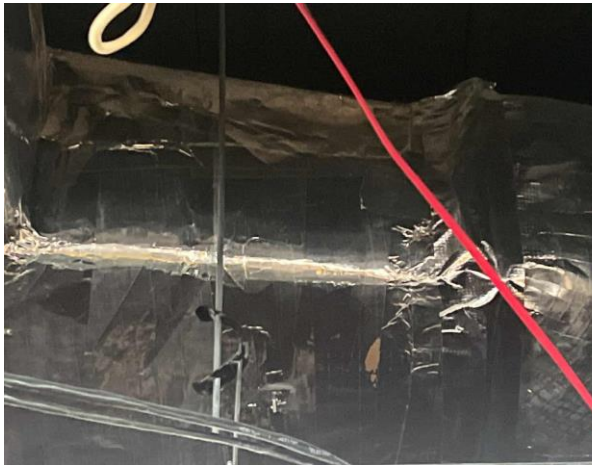
Line ID 162.1: Internal, L2-3, L5-13 and 15-21, Main Office, Rigid Ductwork, Insulation Material - Suspected SMF
