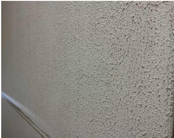
Line ID 81: Internal, L23, North Fire Stairwell, To Concrete Walls, Textured Coating - No Asbestos Detected
