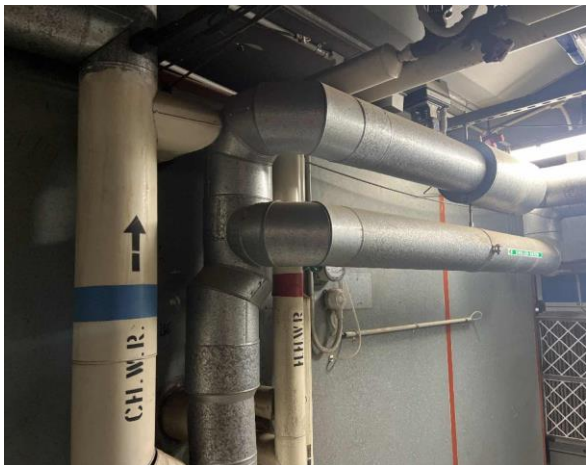
Line ID 135: Internal, L14, Plant Room, Metal Covered Pipes, Insulation Material - Suspected SMF
