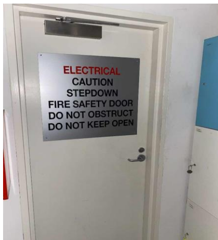
Line ID 94.1: Internal, L2-3, L5-13 and 15-21, Lift Lobby and Electrical Service Room, Fire Entry Door, Fire Door Core - Suspected Asbestos
