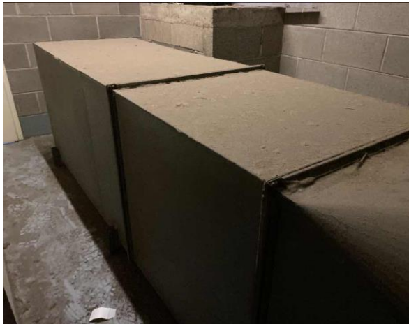
Line ID 26: Internal, GF, External Plant Room, West Exhaust Air Rooms, Ductwork Mastic - No Asbestos Detected
