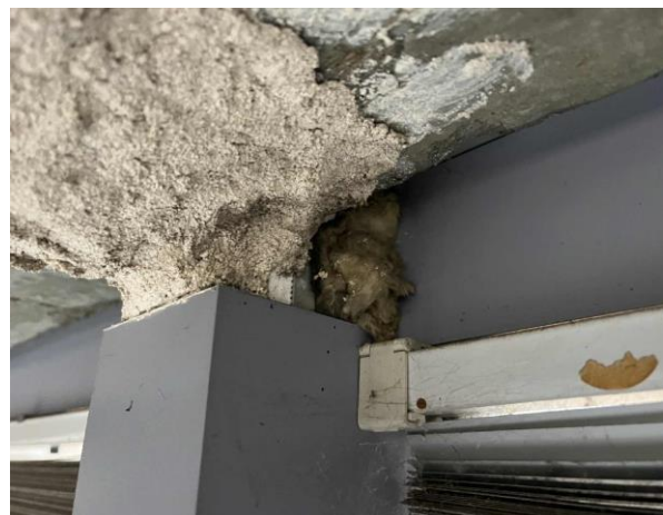
Line ID 138: Internal, L14, Plant Room, To Outer Window Frame Supports, Insulation Material - Suspected SMF
