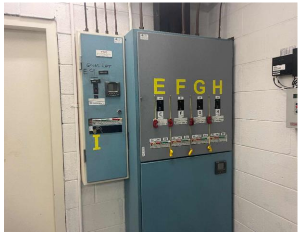
Line ID 78: Internal, L23, Lift Motor Room, Lift Motor Electrical Boards, HRC Fuses - Suspected Asbestos
