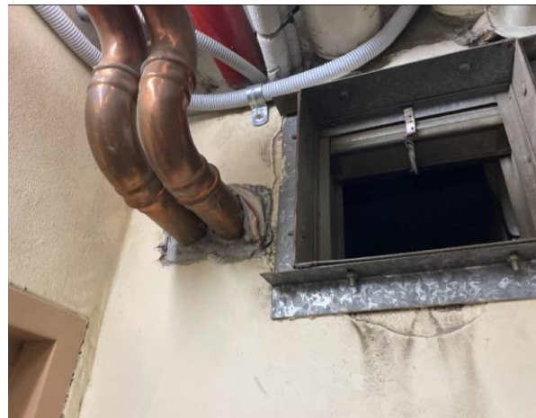
Line ID 136: Internal, L14, Plant Room, Pipework Adjacent Main Entry Door, Pillow Insulation - Suspected SMF
