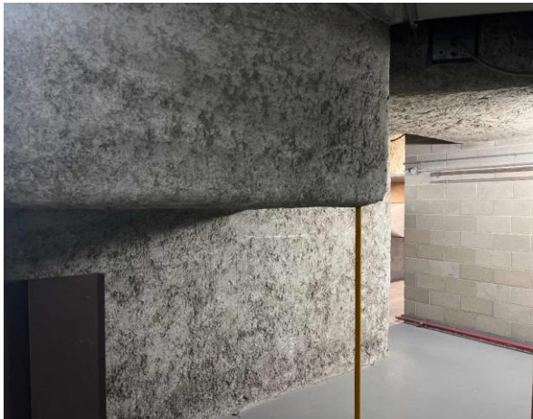
Line ID 55: Internal, L14, Plant Room, To Walls, Ductwork and Steel Beams, Sprayed Vermiculite - No Asbestos Detected
