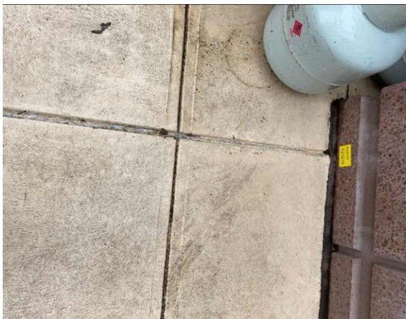
Line ID 67: Internal, L21, External Balcony, Grey Floor Mastic, Construction Joint Mastic - No Asbestos Detected
