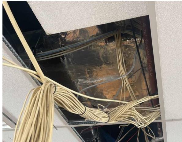
Line ID 162: Internal, L2-3, L5-13 and 15-21, Main Office, Rigid Ductwork, Insulation Material - Suspected SMF
