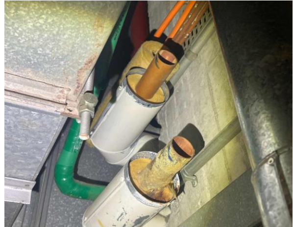
Line ID 146: Internal, L22, Plant Room, Metal Covered Redundant Pipe Work Painted White, Insulation Material - Suspected SMF
