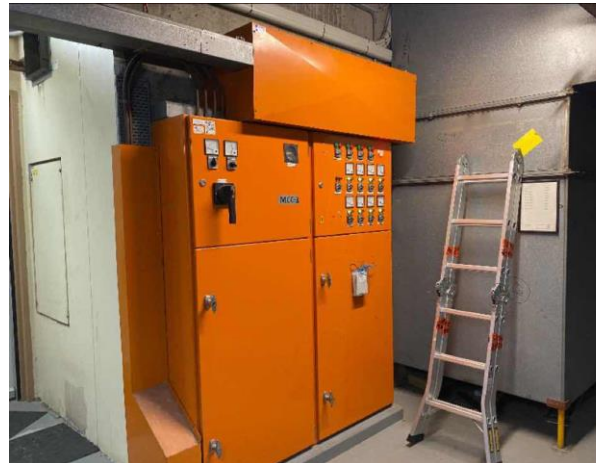
Line ID 53: Internal, L14, Plant Room, Switchboard Adjacent Main Entry Door, HRC Fuses - Suspected Asbestos
