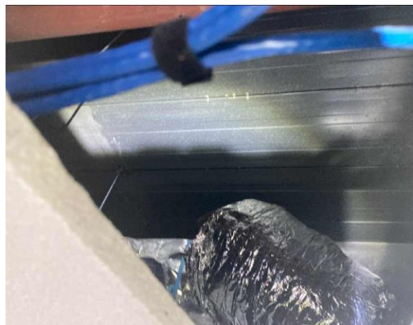
Line ID 163: Internal, L2-3, L5-13 and 15-21, Main Office Areas, Flexible Ductwork, Insulation Material - Suspected SMF
