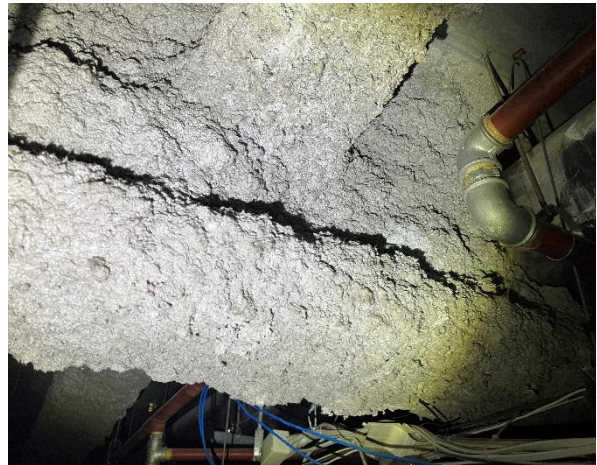
Line ID 62: Internal, L2, L5, L8, L9, L15, L19 and L21, Main Office Areas, Throughout the Underside of the Ceiling to Concrete Columns, Sprayed Vermiculite - No Asbestos Detected
