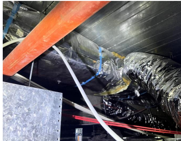
Line ID 160.1: Internal, L2-3, L5-13 and 15-21, Lift Lobby and Electrical Service Room, Rigid and Flexible Ductwork, Insulation Material - Suspected SMF
