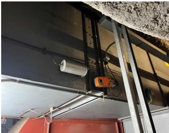
Line ID 48: Internal, L14, Plant Room, Around the Heater Core to the Ductwork, Heater Bank Insulation - Suspected Asbestos
