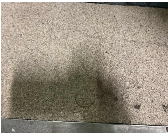
Line ID 64.1: Internal, L20, Lift Lobby Electrical Services Room, Fire Stop to Penetrations, Vermiculite - No Asbestos Detected
