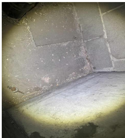
Line ID 90.1: Internal, L23, South Air Handling Unit AHU-7, To Hatch Door Internals to RAF6, Vermiculite - No Asbestos Detected
