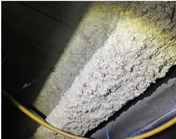
Line ID 60: Internal, L17, Main Office Areas, Throughout the Underside of the Ceiling to Concrete Columns, Sprayed Vermiculite - No Asbestos Detected
