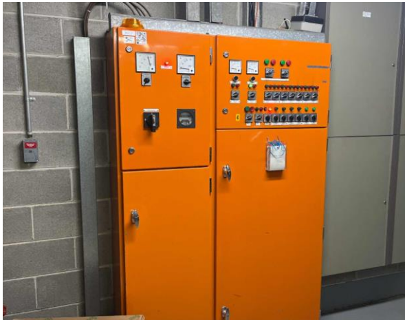
Line ID 21: Internal, GF, External Plant Room, Electrical Cupboards, HRC Fuses - Suspected Asbestos
