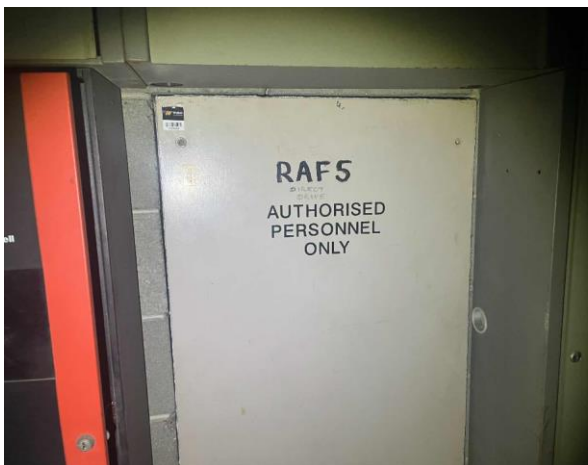
Line ID 85: Internal, L23, Plant Room, Hatch Doors throughout the Plant Room, Vermiculite - No Asbestos Detected
