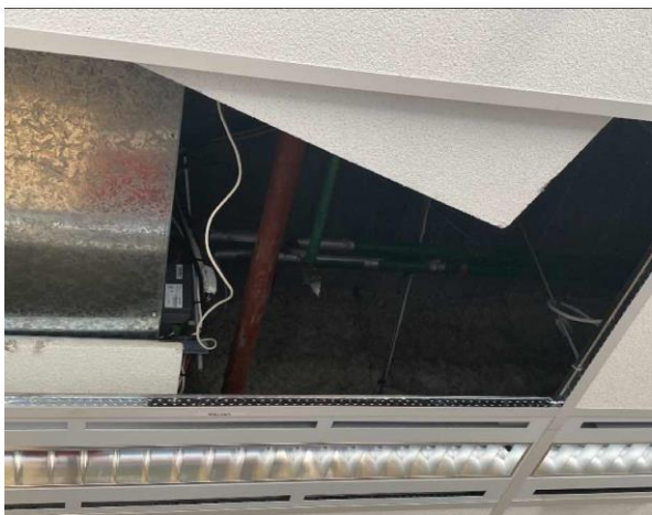
Line ID 33: Internal, L10, Main Office Areas, Throughout the Underside of the Ceiling to Concrete Columns, Sprayed Vermiculite - No Asbestos Detected
