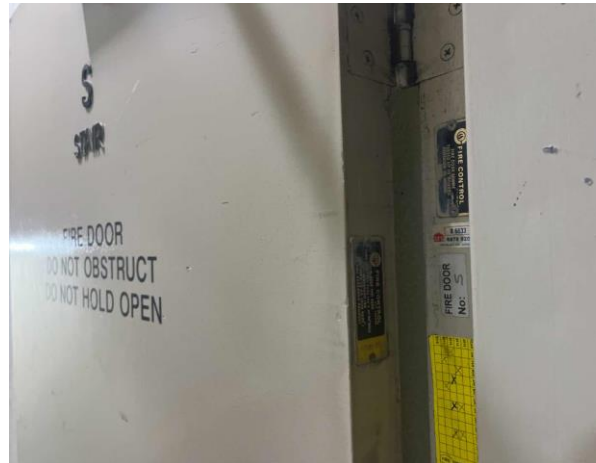
Line ID 92: Internal, L23, South Stairwell, Fire Doors, Internal Fire Door Core - Suspected Asbestos
