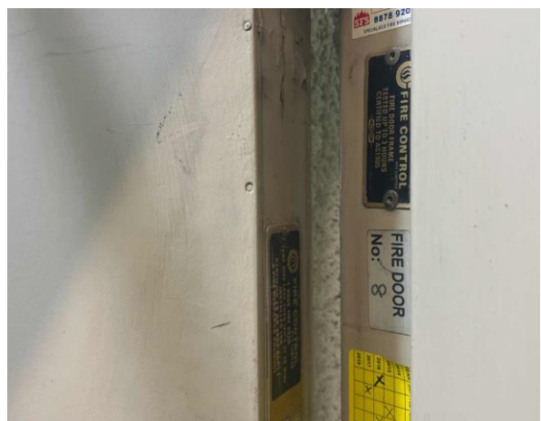
Line ID 80: Internal, L23, North Fire Stairwell, Fire Doors , Internal Fire Door Core - Suspected Asbestos
