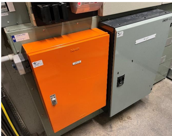
Line ID 95.3: Internal, L2-3, L5-13 and 15-21, Lift Lobby and Electrical Service Room, Grey Switchboards, HRC Fuses - Suspected Asbestos
