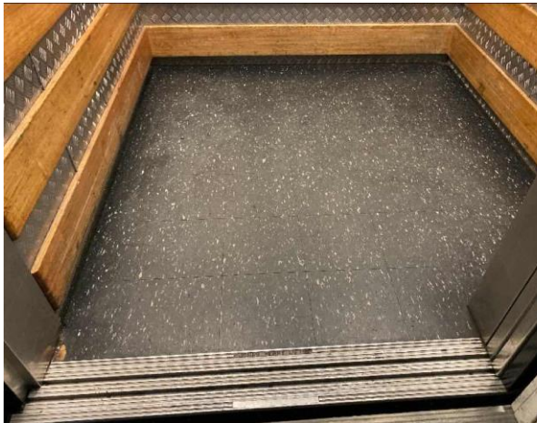
Line ID 31: Internal, Goods Lift, Floor, Black Speckled Floor Tiles, Vinyl Floor Tiles - No Asbestos Detected
