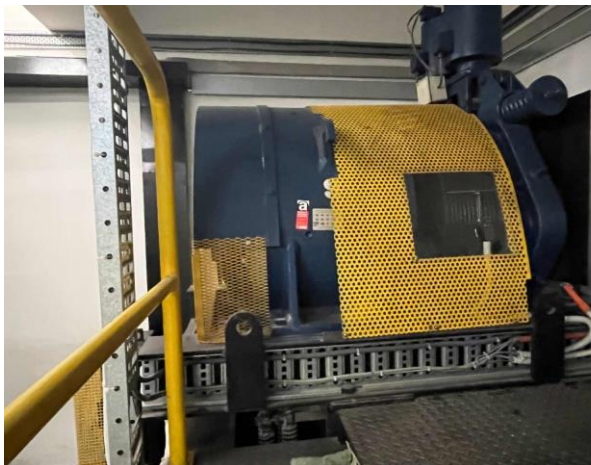
Line ID 77.1: Internal, L23, Lift Motor Room, Lift Motor Brake Pads, Friction Material - No Asbestos Detected
