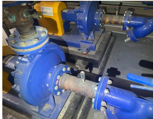
Line ID 73: Internal, L22, Plant Room, To Pipe Work of Pump Machinery, Blue Gasket Material - No Asbestos Detected
