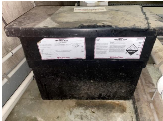
Photo 08. Level 22 Plant Room, cooling tower chemicals.
