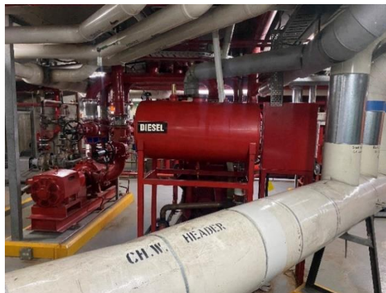
Photo 02. Level 23 Sprinkler Pump Room, Diesel Fuel Storage.
