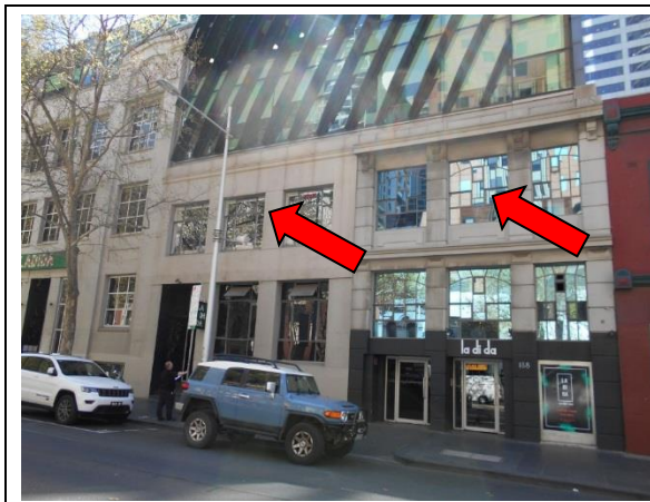
Exterior, Original Façade, Windows – Asbestos containing mastic sealant
