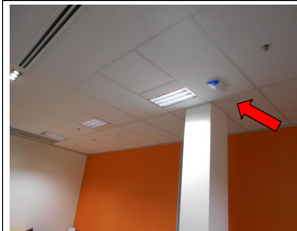
Photo 5: Level 2, Office Area, Ceiling – SMF compressed ceiling tiles
