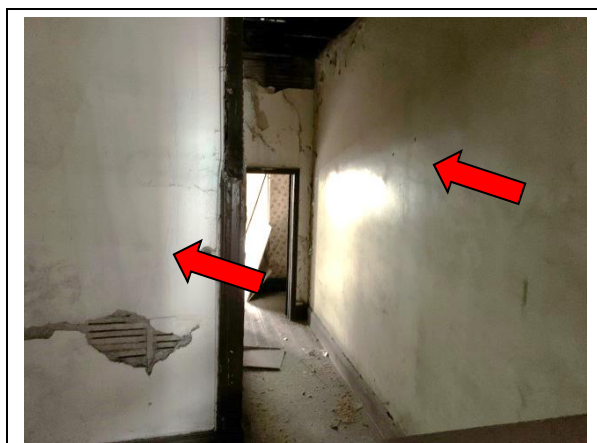
Photo 7: Lord of the Fries Building – Level 1, Walls (positive lead paint sample on the white paint)
