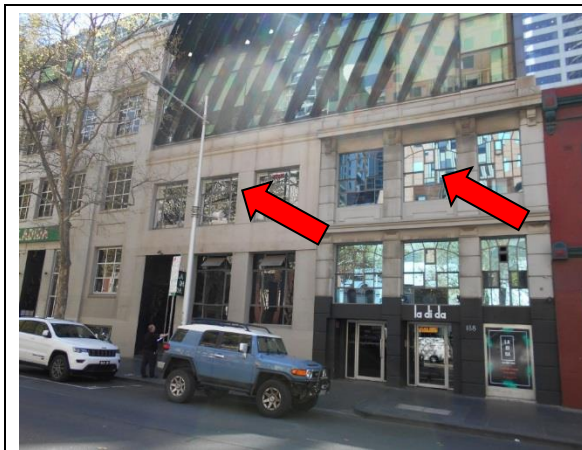
Photo 1: Exterior, Original Façade, Windows – Asbestos containing mastic sealant
