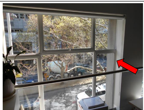
Photo 2: Interior, Original Façade, Windows – Asbestos containing mastic sealant (Photo taken from Level 2)
