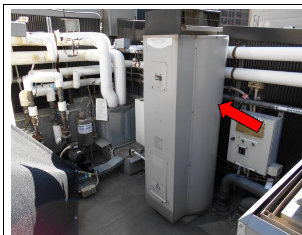
Photo 3: Level 4, Roof Area, Adjacent Chiller – SMF internal insulation to hot water heater
