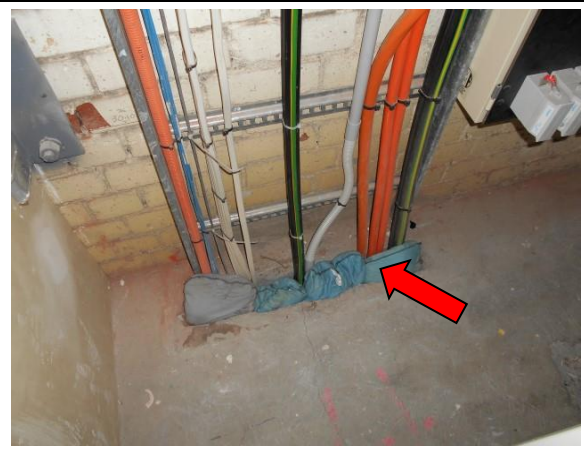
Photo 6: All Levels, Electrical Cupboards, Penetrations – SMF pillow insulation
