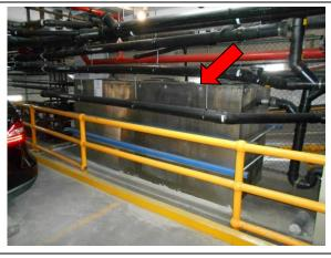
No confined space signage was installed on grease traps on Level B2
