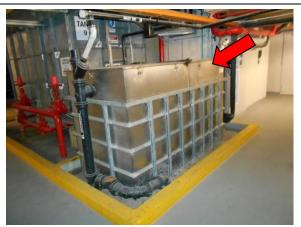
No confined space signage was installed on grease traps on Level 37
