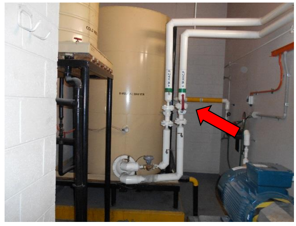
Photo 11: Level 37, Plant Room, Calorifier – SMF internal insulation
