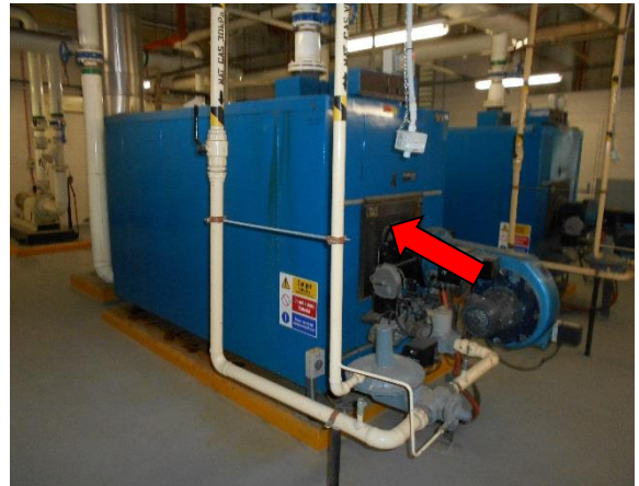
Photo 4: Level 51, Plant Room, Boiler Room Boiler, Inlet Manifold – Asbestos containing gasket
