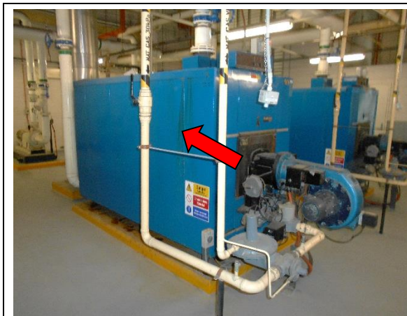
Photo 6: Level 51, Plant Room, Boiler Room – SMF internal insulation to boilers
