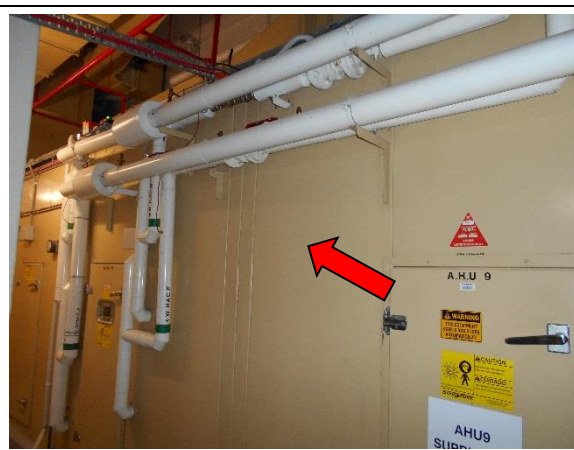
Photo 13: Level 37, Air Handling Units (positive lead paint sample on the yellow paint)
