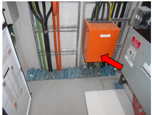
Photo 9: All Levels, Electrical Riser Cupboards – SMF pillow insulation
