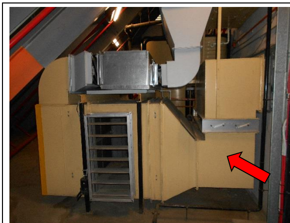
Photo 12: Level 53, Throughout, Ductwork (positive lead paint sample on the yellow paint)
