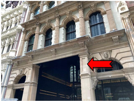
Photo 1 Exterior: throughout façade – suspected asbestos containing mastic.
