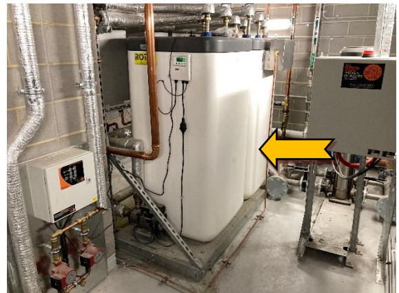
Photo 4 Interior: loading dock, hot water heater – suspected SMF internal insulation material.
