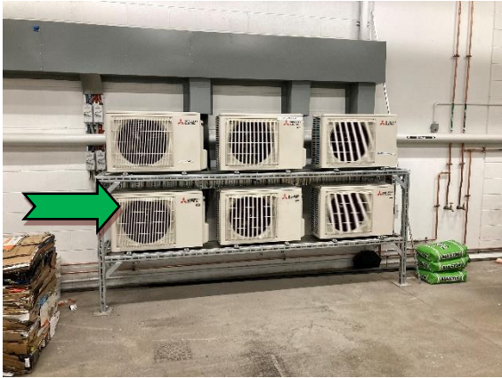
Photo 7 Interior: loading dock, air conditioning units – non ODS refrigerant.
