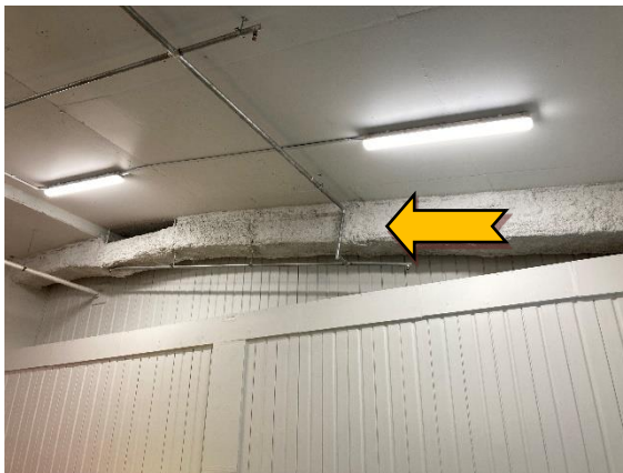
Photo 3 Interior: throughout, air conditioning ductwork – suspected SMF external insulation material.
