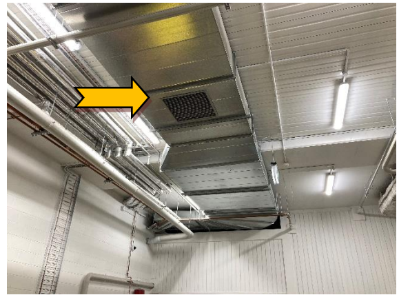
Photo 2 Interior: throughout, air conditioning ductwork – suspected SMF containing internal insulation material.
