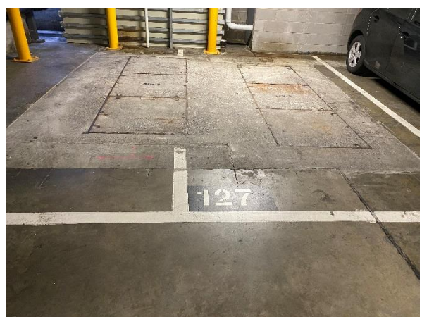
Photo 24. Basement, parking bay 126 and 127, grease interceptor pit x 2
