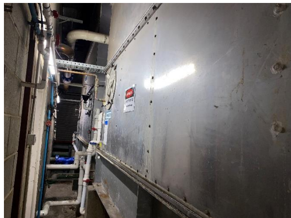
Photo 03. 4 RSQ, Plant Room, cooling tower x 3
