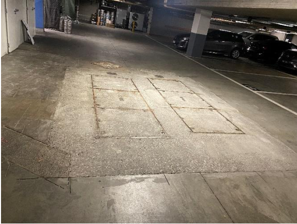
Photo 19. Basement, adjacent parking bay 112, grease interceptor pit x 2
