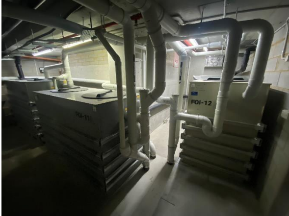
Photo 31. Basement, adjacent parking bay 60, above ground grease trap x 3
