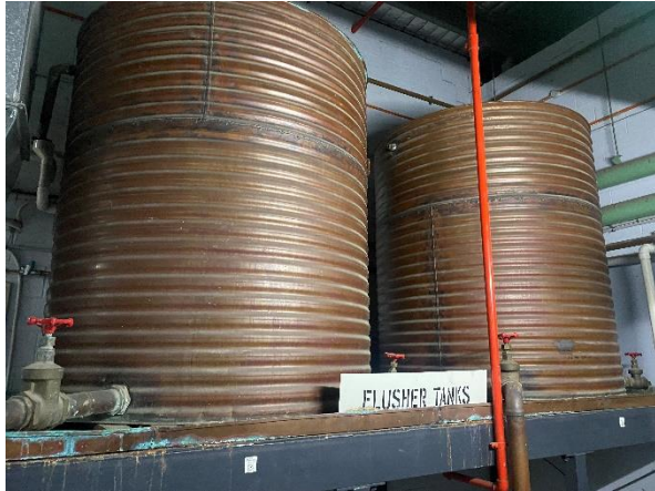
Photo 07. 6 RSQ, Plant Room, flusher water tank x 2
