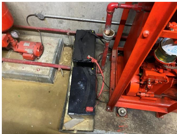
Photo 02. 1 Southbank Boulevard, basement, fire pump room, lead acid batteries.
