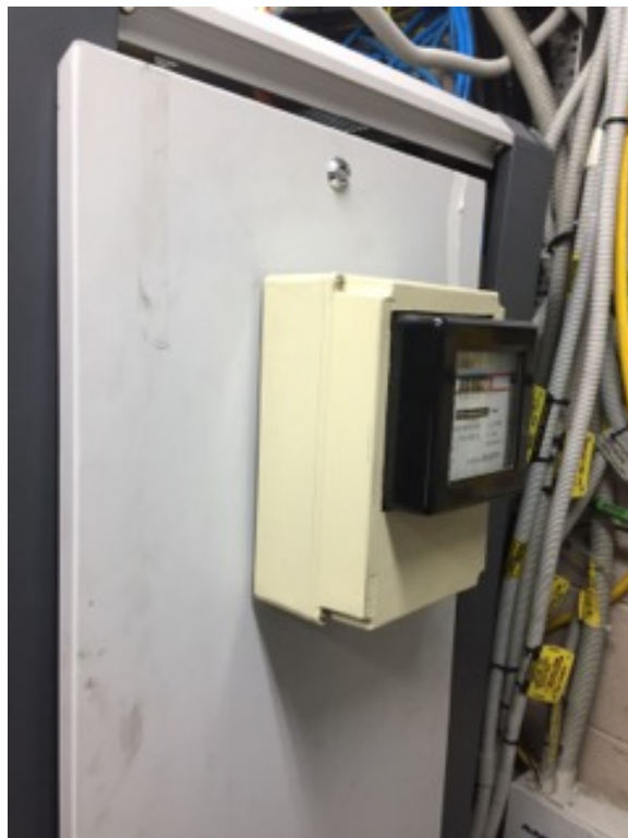
MDF Room – UeComm rack, unsafe power supply
