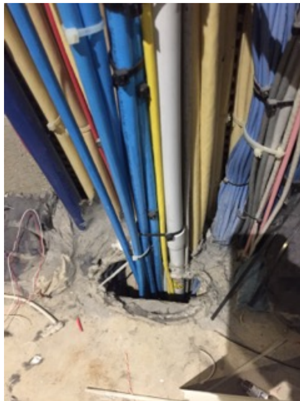
Riser L2 – rubbish, missing fire stopping
