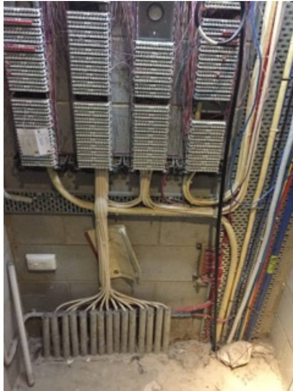
Riser L6 – firestopping missing
