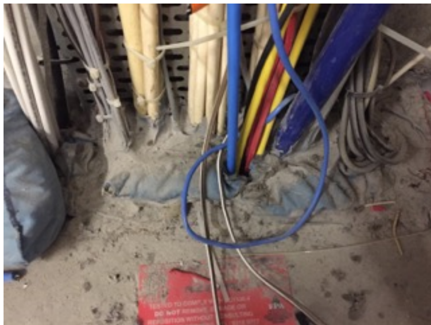
Riser L8 – missing fire stopping
