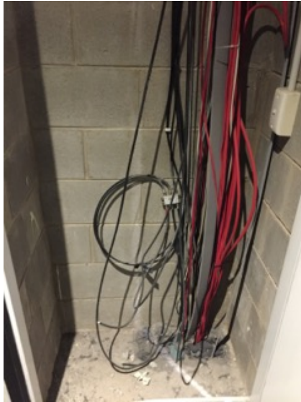
Riser L2 - missing fire stopping, redundant cables
