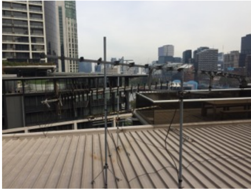
Roof – unknown digital TV yagi antennas
