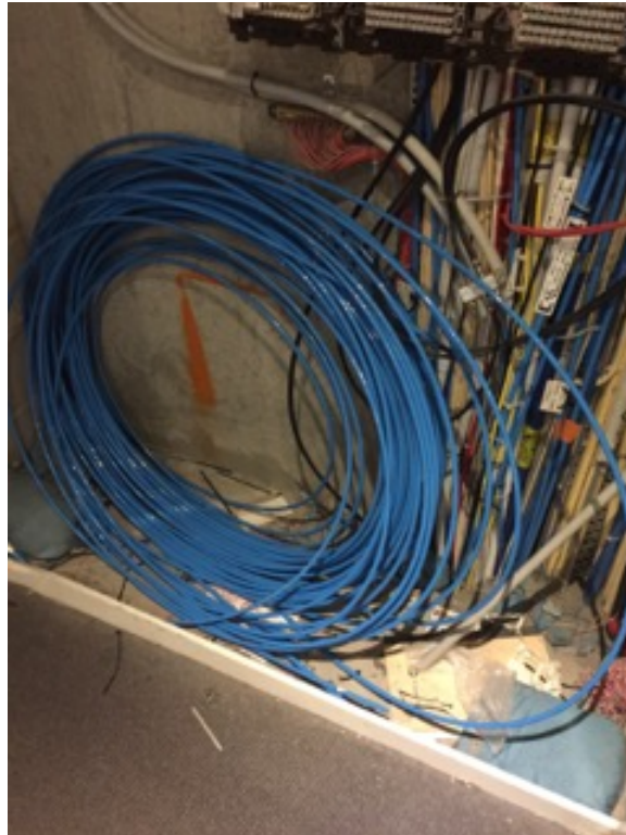
Riser L4 – redundant cabling
