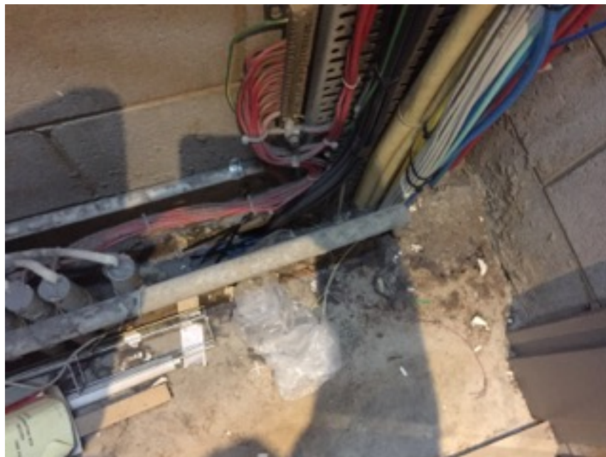
Riser L4 - rubbish, fire stopping missing
