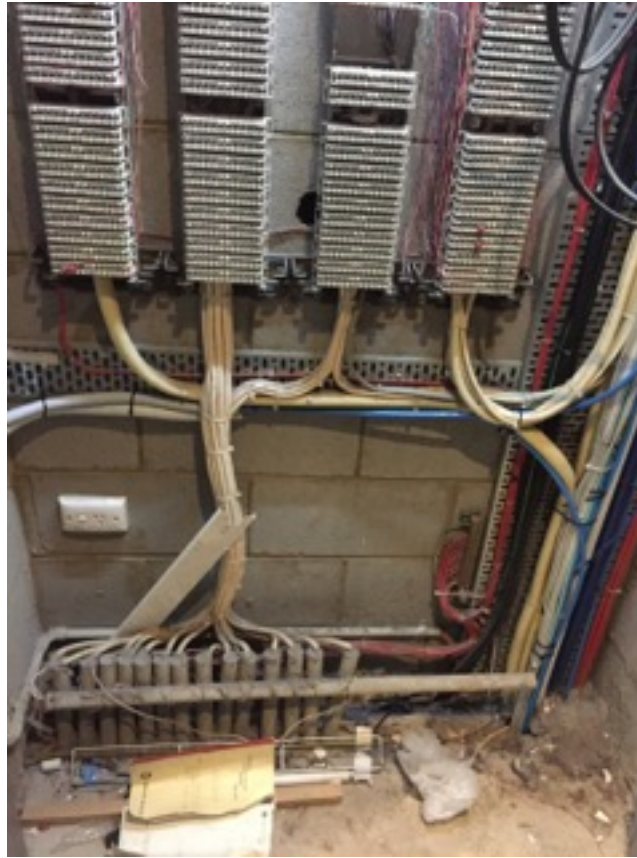
Riser L4 – rubbish, fire stopping missing
