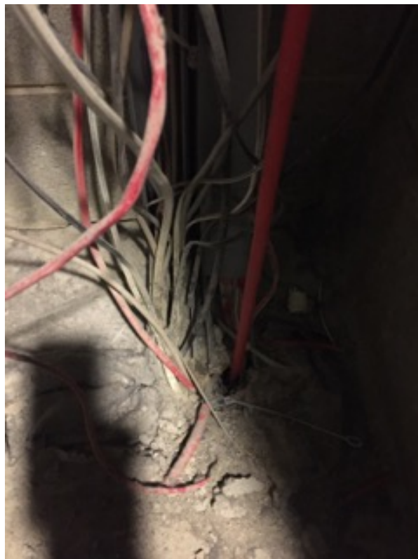
Riser L4 – missing fire stopping, redundant cables
