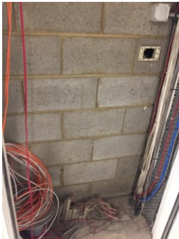
Riser G – redundant cabling, fire stopping missing
