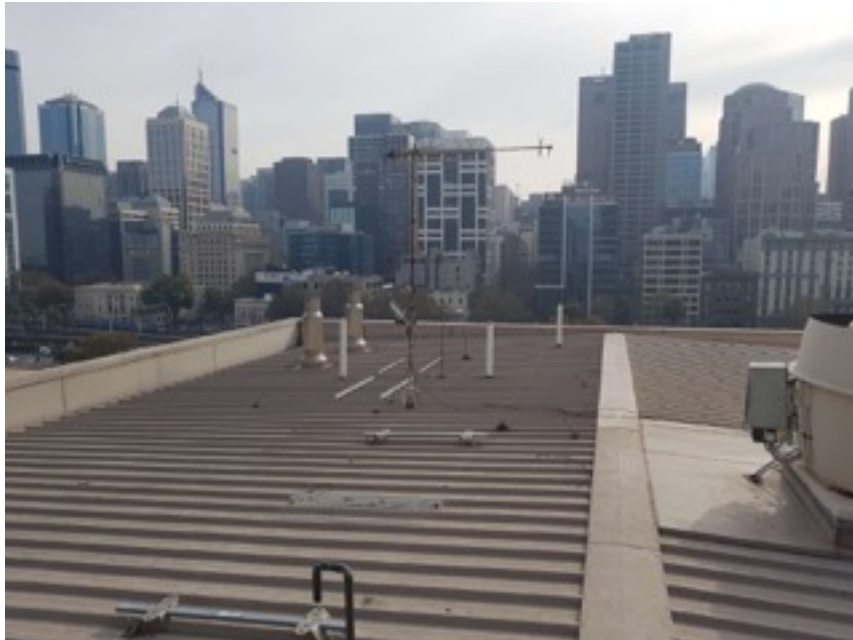
Roof – Unknown digital TV yagi antennas
