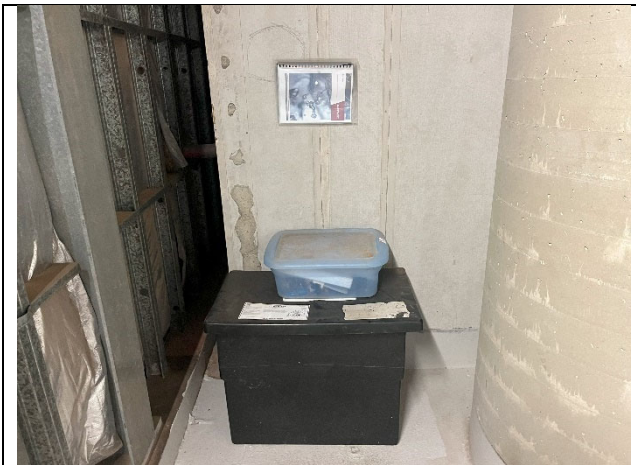
Photo 01. Chemicals in secondary containment, and SDS folder in the Level 32 Plant Room.
