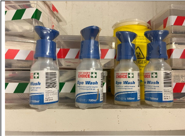
Photo 13. Basement level, Basement Recycling Room 2, eye wash bottles.
