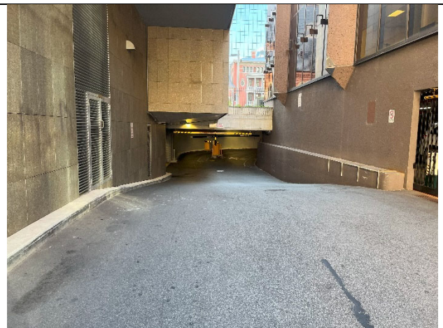
Photo 16. Vehicle entrance to the site with no HAZCHEM placard.
