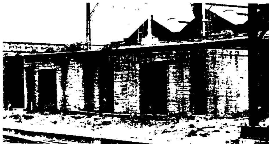
Fig. 53 Loco Workshops - Bomb Shelter During the Second World War, several reinforced concrete box-type bomb shelters were erected in convenient locations around the workshops. Fortunately, they were never required.
