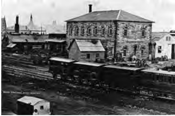
Figure 2.11 The first Sydney yard, which was located further towards the current location of Central Station. (Source: State Rail Authority Archives)
