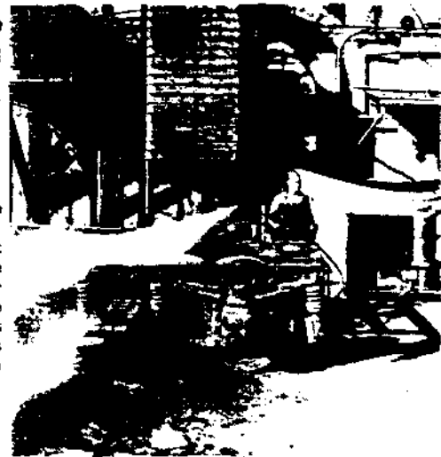
Fig. 33. Carriage Workshops Outside Bay 16. Cleaning a carriage bogey using what appears to be a portable high pressure water unit, the hydraulic power unit for the Carriage Workshops is in the background. The accumulator with its heavy iron weights is halfway up its travel, indicating the system is in operation.
