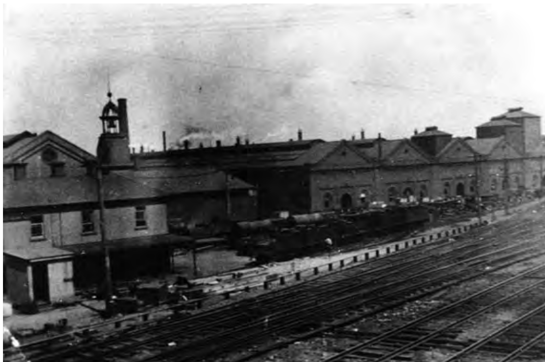
Figure 2.19 View of the works manager's office and the locomotive workshops some time between 1905 and 1922. The New Locomotive Shop has been constructed, but the Works Manager's Office has not yet been extended. (Source: State Rail Authority Archives)
