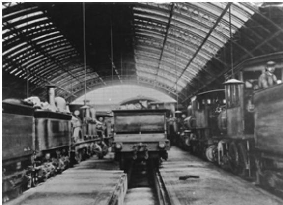
Figure 2.13 Interior of the Engine Running Sheds. (Source: State Rail Authority Archives)
