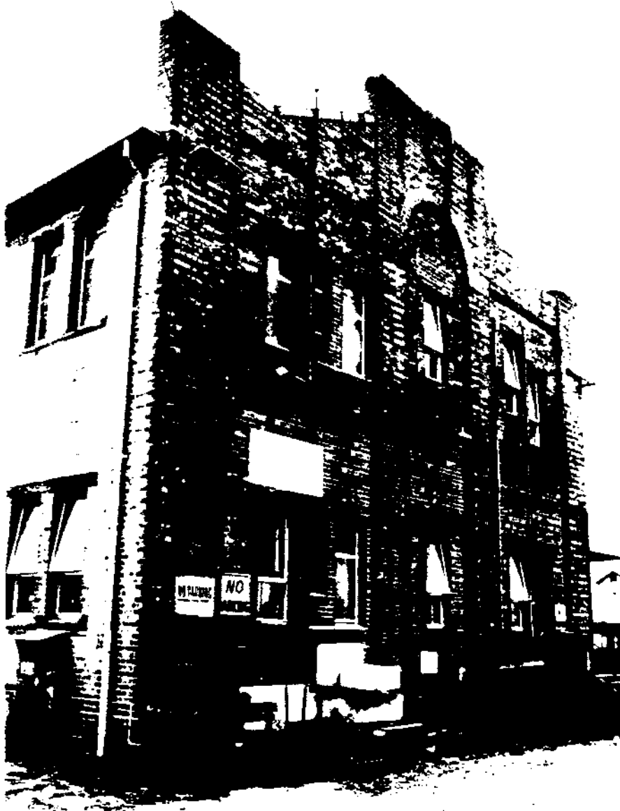
Fig. 39. Carriage Workshops - Stores Building.
