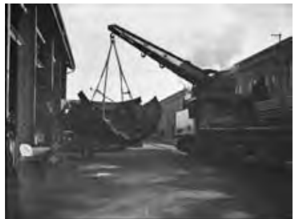
2.16 Outside the Large Erecting Shed in 1938. (Source: Hood Collection, State Library of NSW)
