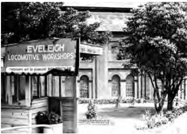
Figure 2.27 Entrance to the Locomotive Workshops from Cornwallis Street in 1986, showing the New Locomotive Workshops in the background. (Source: Don Godden & Associates)
