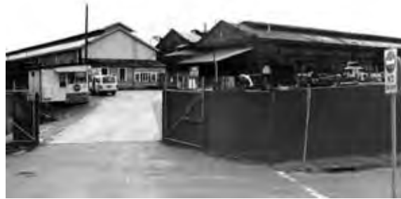
Figure 2.26 The locomotive workshops from Garden Street in 1986. The oliver smiths shop is the building on the left. (Source: Don Godden & Associates)
