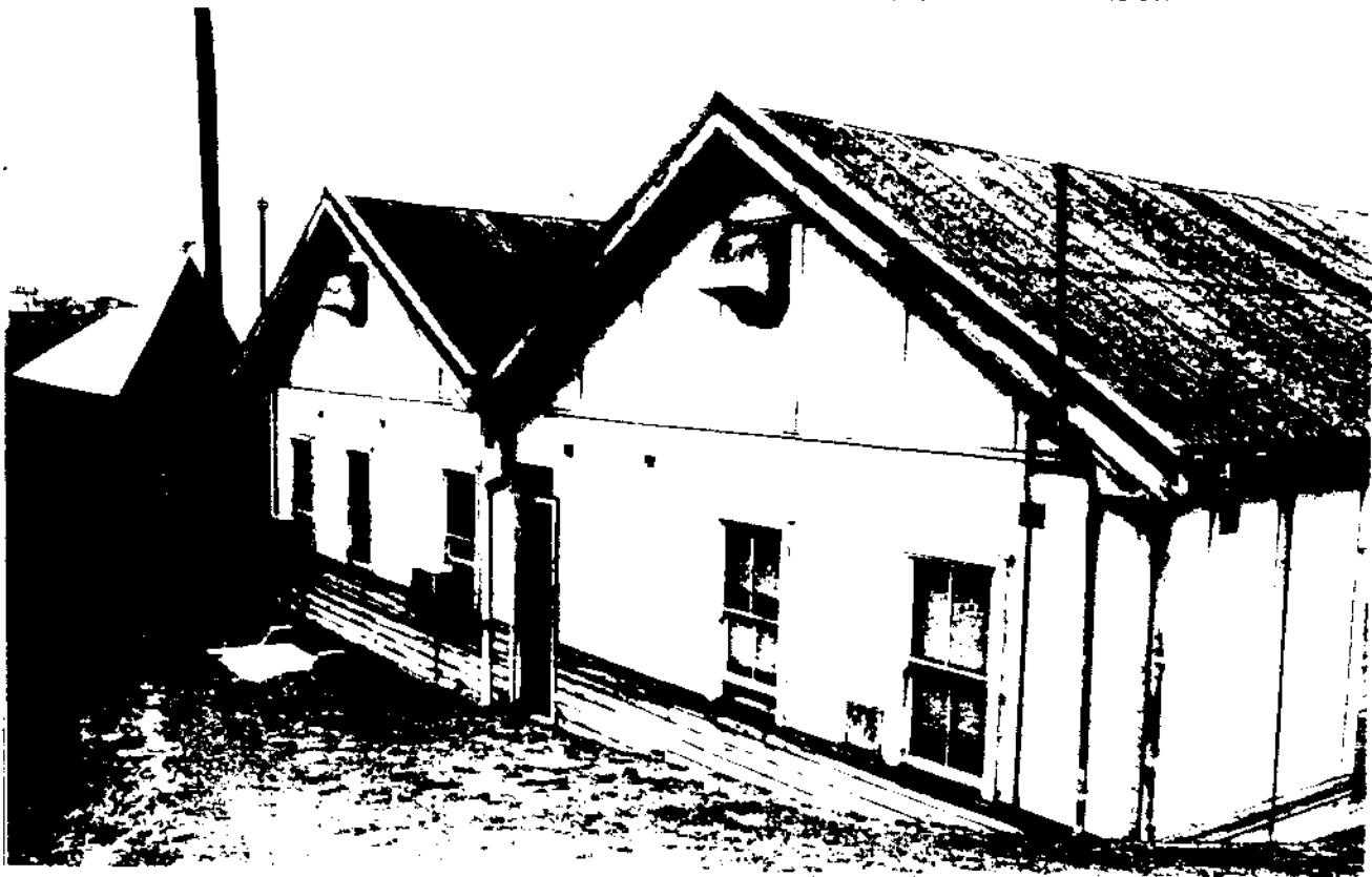
Fig. 49. Carriage Workshops, Train Equipment Stores. Erected during the 1920's as a drawing office and unspecified workshop, these buildings have housed a variety of uses leading to their present use as Train Equipment Stores. (C2 36)
