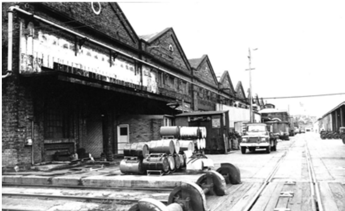
Figure 2.24 The locomotive workshops in 1986, showing the traverser between the locomotive workshops and the large erecting shed. The building just visible on the right was the old Wheel Press Shop. (Source: Don Godden & Associates)
