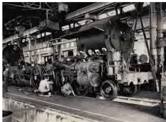
Figure 2.30 Construction of a C3806 locomotive at the Eveleigh Locomotive Workshops in April 1945, most likely in the Large Erecting Shed. (Source: State Records NSW)
