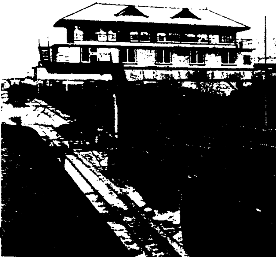
Fig. 45. Eveleigh Railway Yard, Illawarra Junction Signal Box. Following the quadruplication of the suburban rail lines and the completion of the construction of the Illawarra lines, the Eveleigh Railway Yard became a complicated array of tracks, sidings and junctions leading to the Central Station terminal. The management and safe-working of the yard was conducted from the elevated Illawarra Junction Signal Box. (A9)
