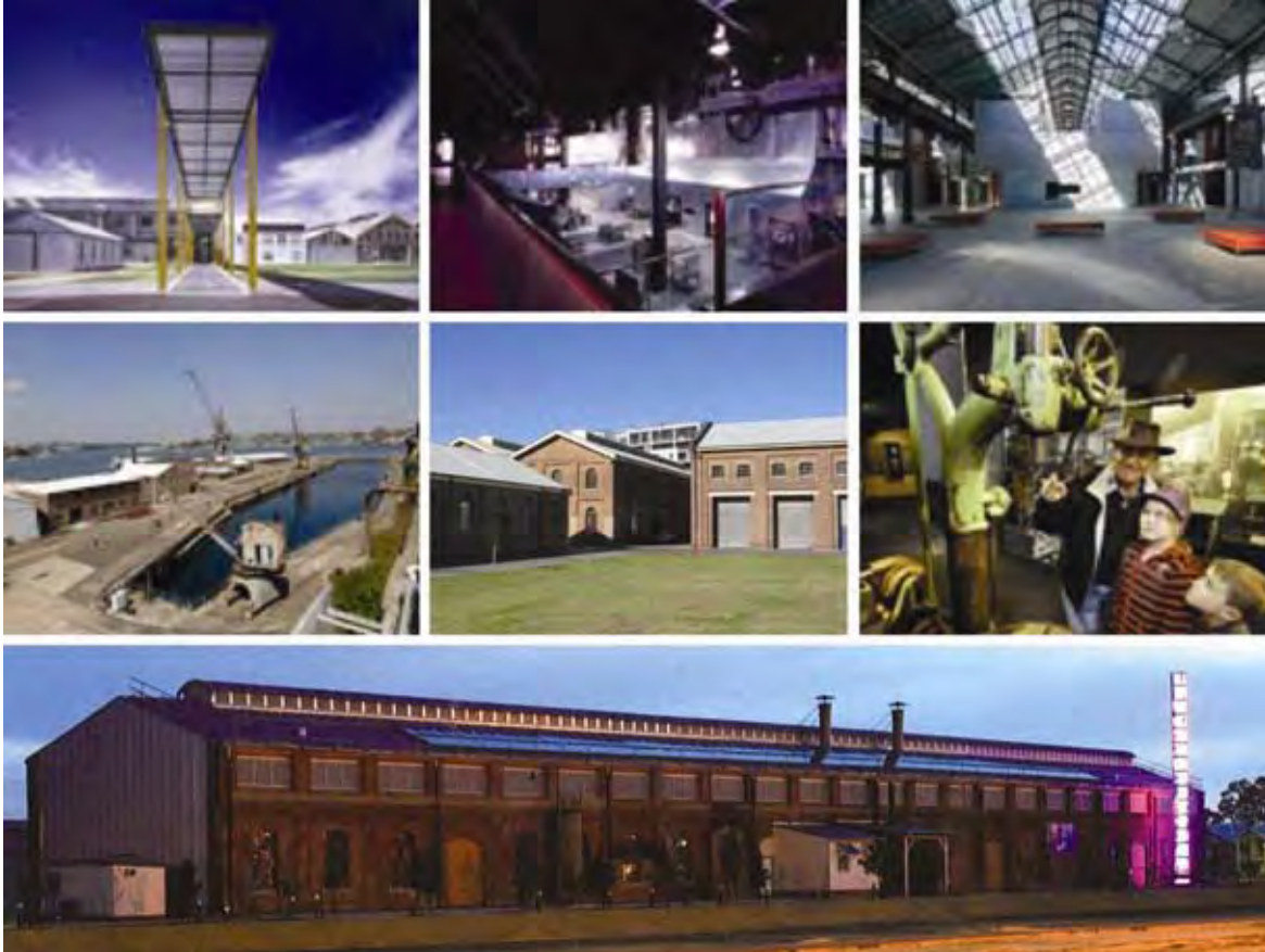
Figures (left to right) 3.30 Queen Victoria Museum and Art Gallery, former Launceston Railway Workshops (Source: Department of the Environment and Heritage, Adaptive Reuse, The Queen Victoria Museum and Art Gallery, 2004); 3.31 Canberra Glassworks; 3.32 CarriageWorks, North Eveleigh (Source: Architecture Australia, CarriageWorks, John De Mannicor, Jul/Aug 2007); 3.33 Cockatoo Island (Source: Sydney Harbour Federation Trust, < http://www.cockatooisland.gov.au/ >); 3.34 Civic Railway Workshops, Honeysuckle (Source: GML 2008); 3.35 The workshops rail museum Queensland, North Ipswich (Source: Queensland Museum < http://www.theworkshops.qm.qld.gov.au/ >); 3.36 Midlands Atelier (Source: Heritage Matters brochure, Heritage Council of Western Australia, 2010)
