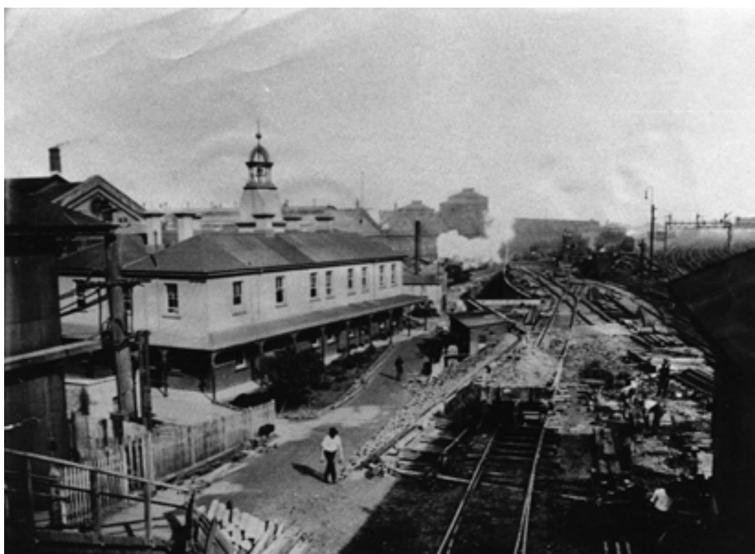
Figure 2.20 View of the works manager's office and the locomotive workshops pre-1940s. The locomotive dive has been constructed. (Source: State Rail Authority Archives)
