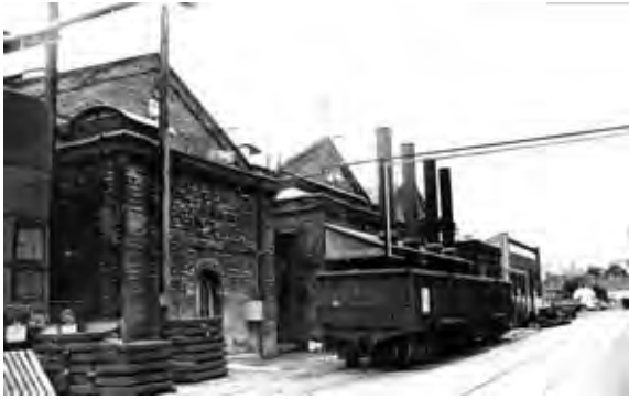
Figure 2.25 The locomotive workshops in 1986. The New Locomotive Shop can be seen in the distance. (Source: Don Godden & Associates)
