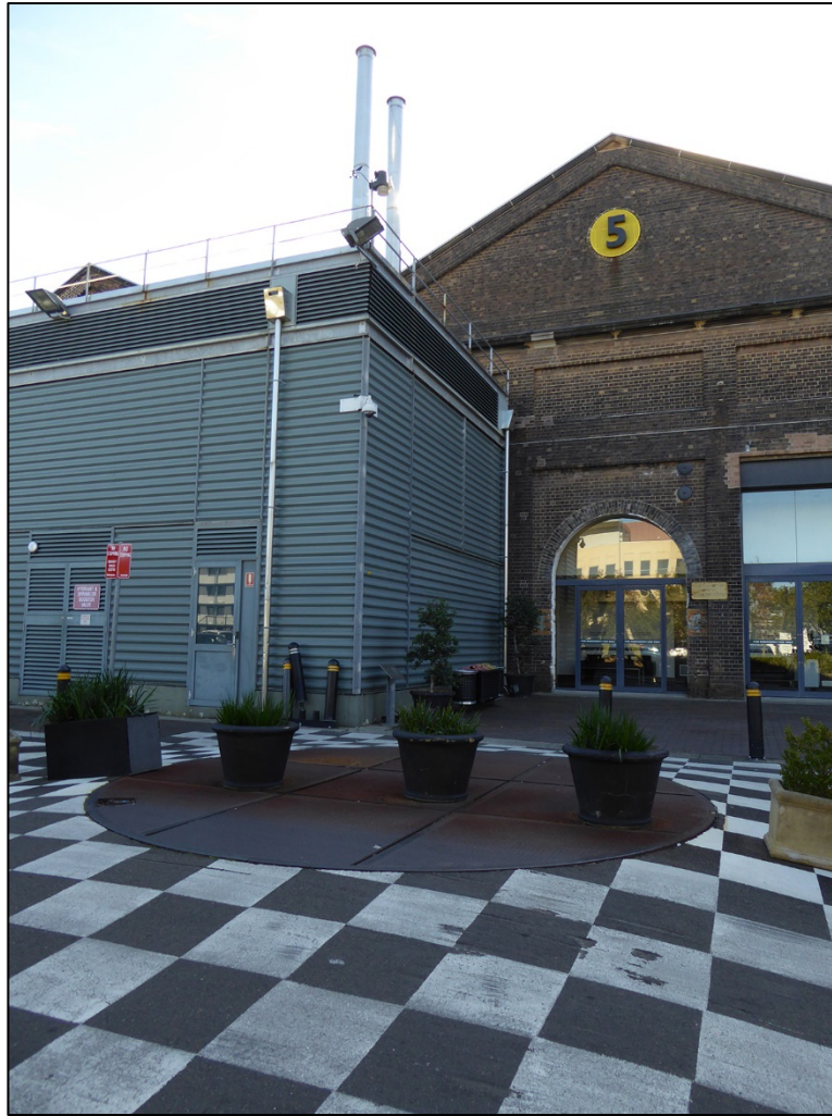
FIGURE 47: TURNTABLE IN FRONT OF BAY 5, CURRENTLY BEING USED AS A SPEED HUMP/LOCATION FOR POTS. (SOURCE: CURIO PROJECTS 2016)
