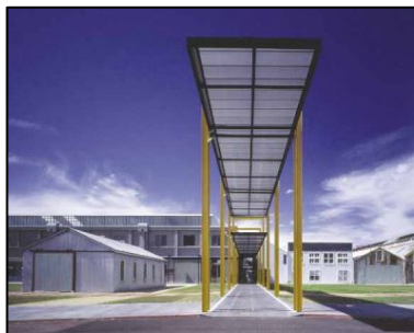
FIGURE 25: QUEEN VICTORIA MUSEUM AND ART GALLERY, FORMER LAUNCESTON WORKSHOPS (SOURCE: ADAPTIVE REUSE, DEPARTMENT OF ENVIRONMENT AND HERITAGE, 2004:11)
