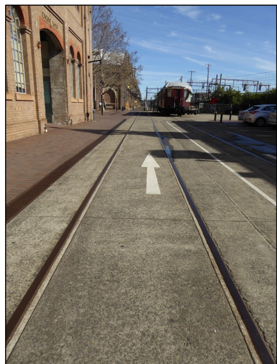
FIGURE 63: CURRENT RAILWAY TRACKS BETWEEN INNOVATION PLAZA AND ENTRY GARDEN (SOURCE: CURIO 2016)
