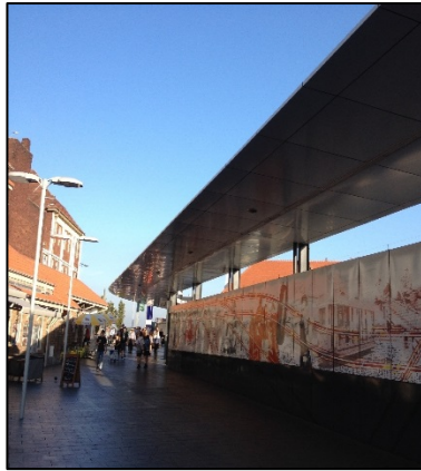
FIGURE 28: HERITAGE INTERPRETATION AT NEWTOWN STATION (SOURCE: SHR LISTING)
