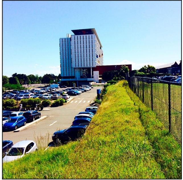
FIGURE 41: VIEW ACROSS TOP OF THE FOUNDRY WALL, WEST, MEDIA CITY BUILDING IN BACKGROUND. (SOURCE: CURIO PROJECTS 2016)
