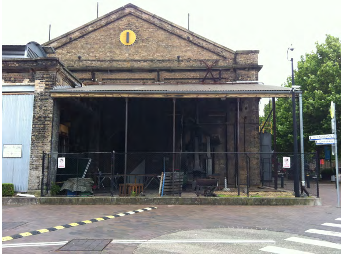
Figure 4 – Looking north into the Bay 1 Annex. Innovation Plaza is visible on the very right of photograph.
