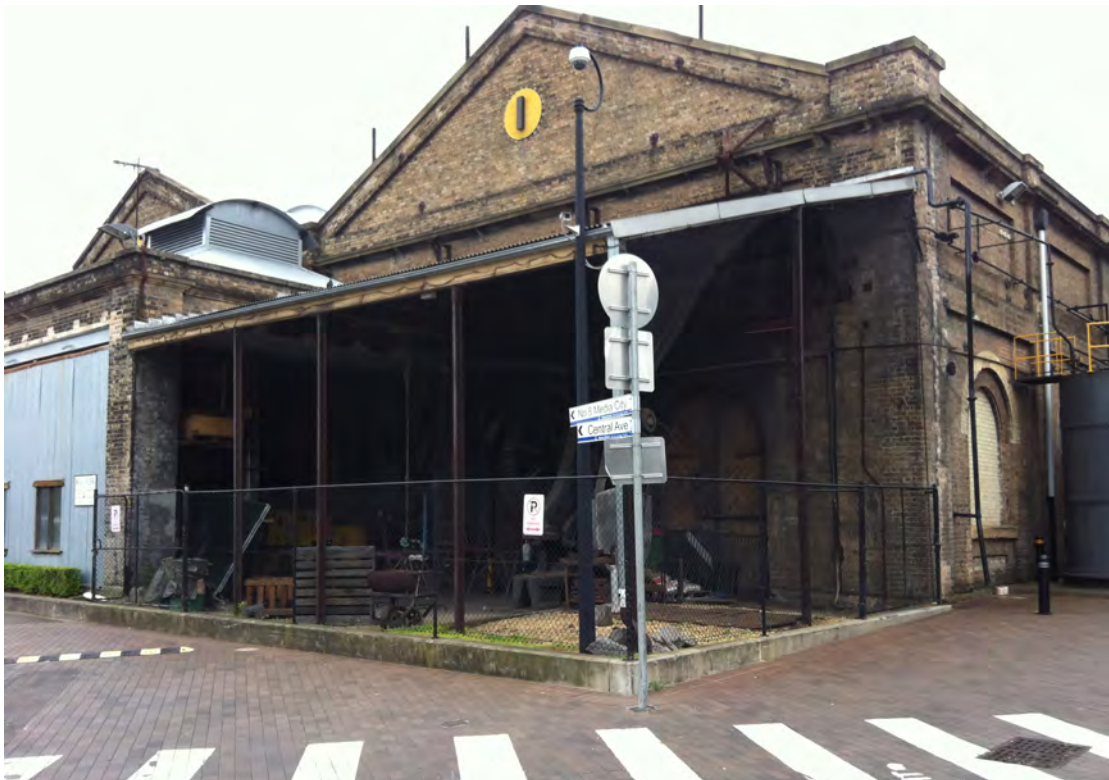
Figure 6 – Looking north-west into the Bay 1 Annex.
