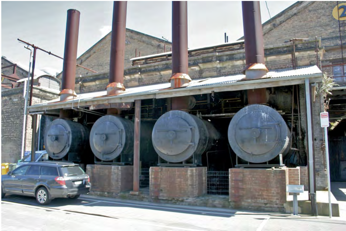
Figure 3 – Looking north into the Boiler Area in front of Bay 2.
