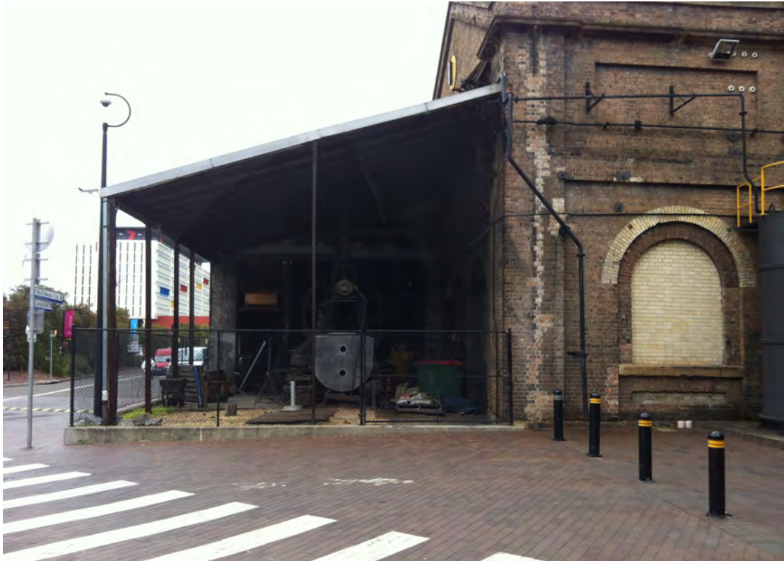
Figure 5 – Looking west from Innovation Plaza into the side of the Bay 1 Annex.
