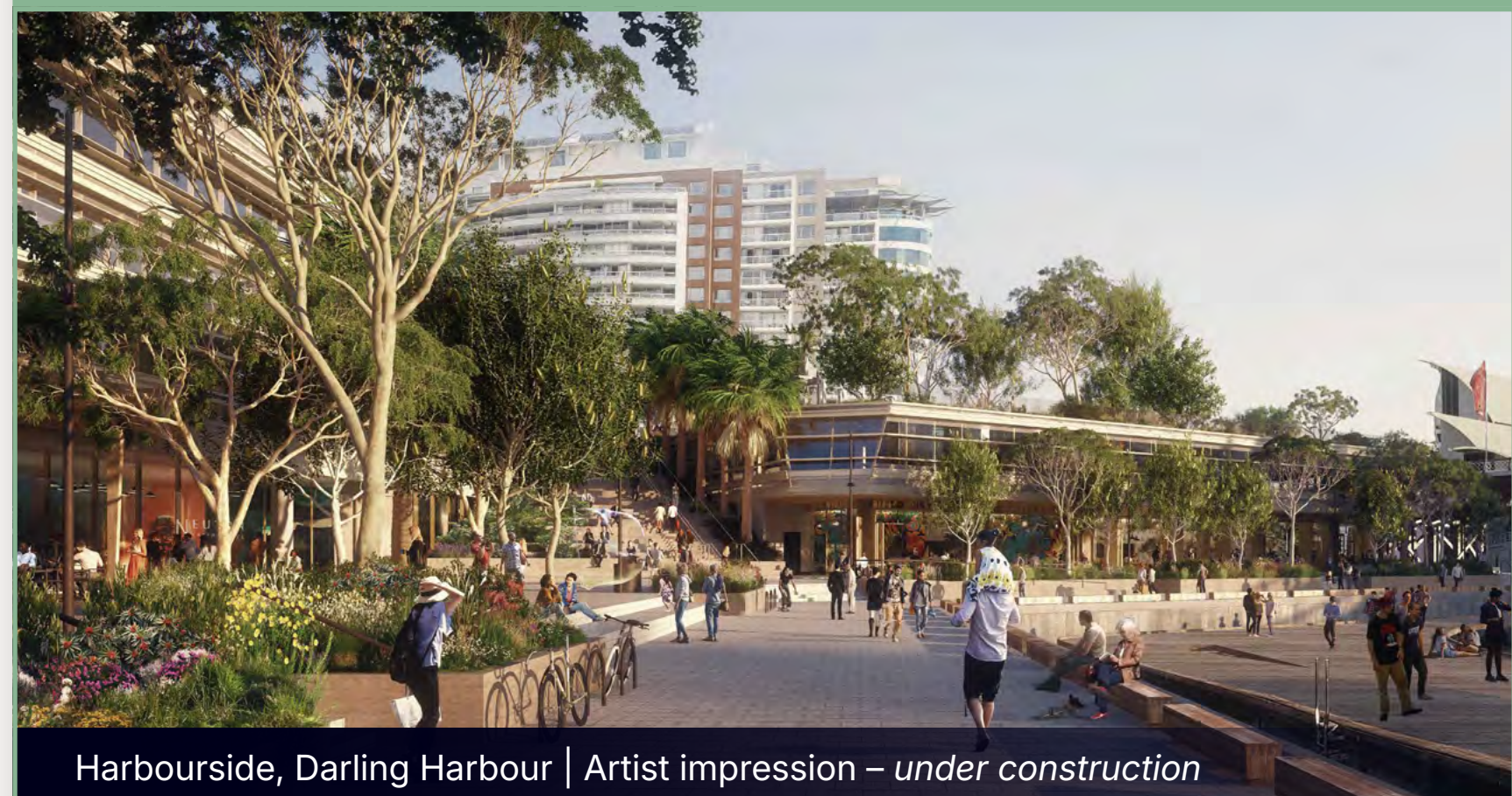
Harbourside, Darling Harbour | Artist impression – under construction
