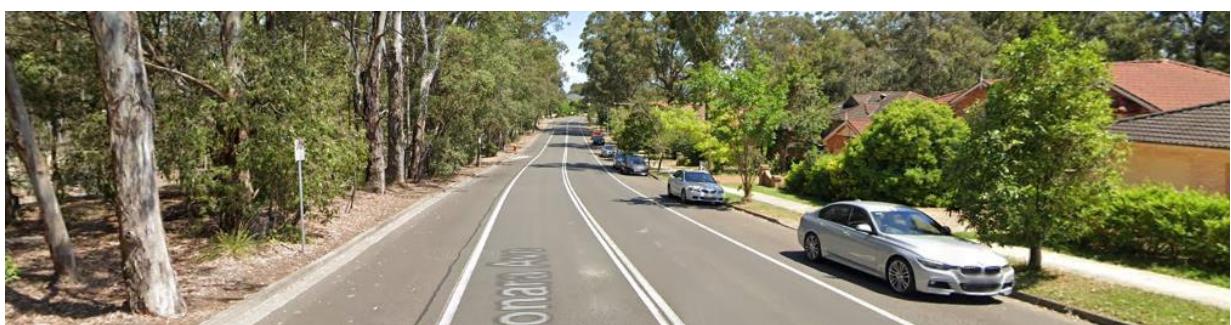
Figure 5: Coonara Avenue Westbound
