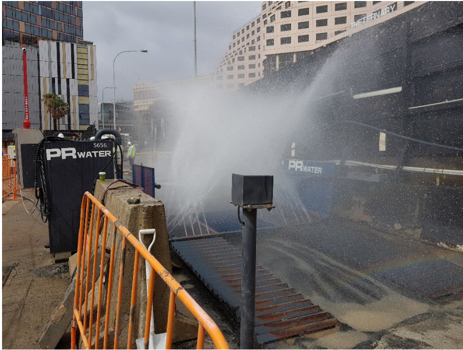
Photo 19: New truck and wheel wash at the site's exit. 23/01/24
