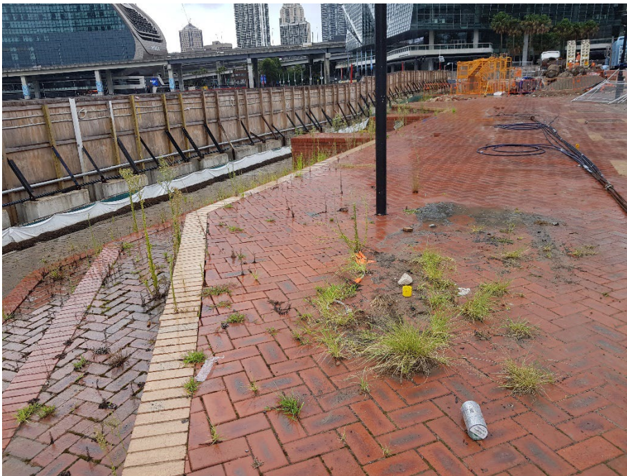
Photo 26: View to the southeast along the eastern site boundary hoarding showing the sediment controls that were maintained during the preceding week. The site level is lower along some parts of the eastern boundary 23/01/24
