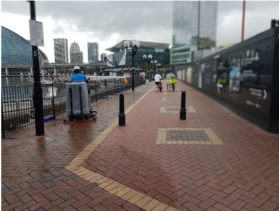
Photo 7: Looking south along the public boardwalk. A site worker is cleaning the boardwalk with a small street sweeper cleaning machine. 16/01/24
