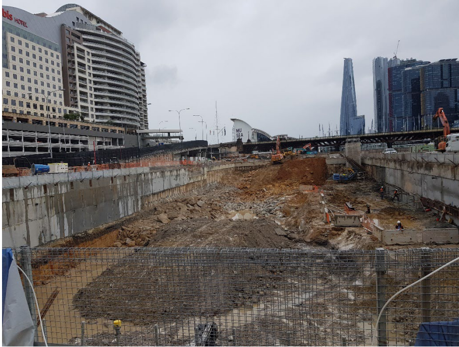
Photo 33: View to the north across the basement excavation. 23/01/24
