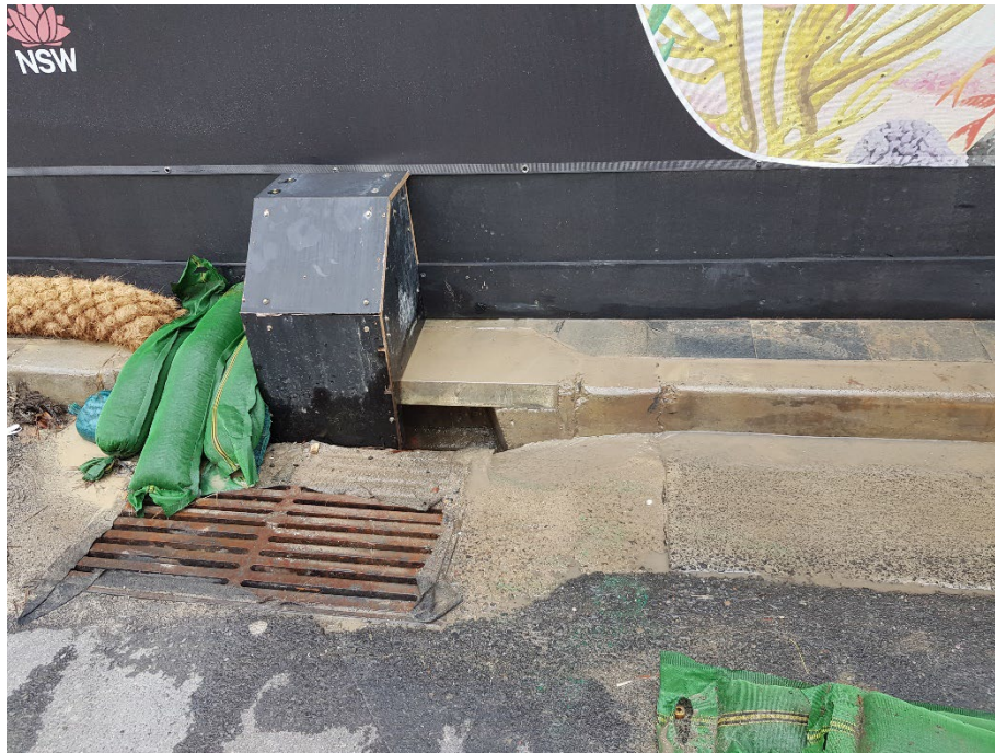
Photo 13: The street stormwater drain where the treated water from the Dewatering Treatment Plant discharges to the PMNSW stormwater system. Sediment controls were in place. 09:44 16/01/24
