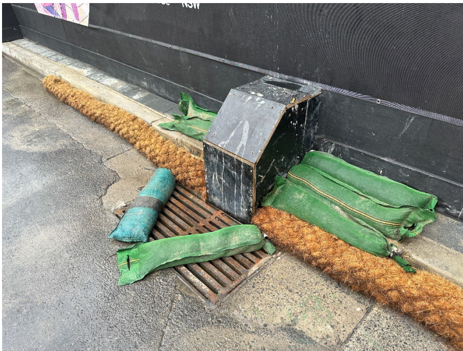
Photo 16: The same stormwater drain a week later with additional sediment controls. 23/01/24
