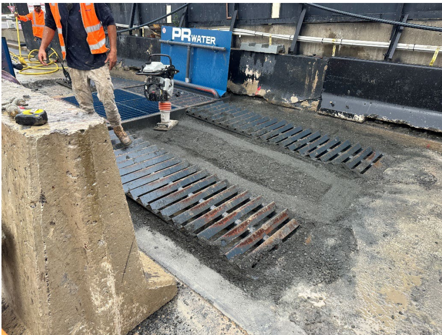
Photo 18: Stabilised truck entry under construction. 23/01/24
