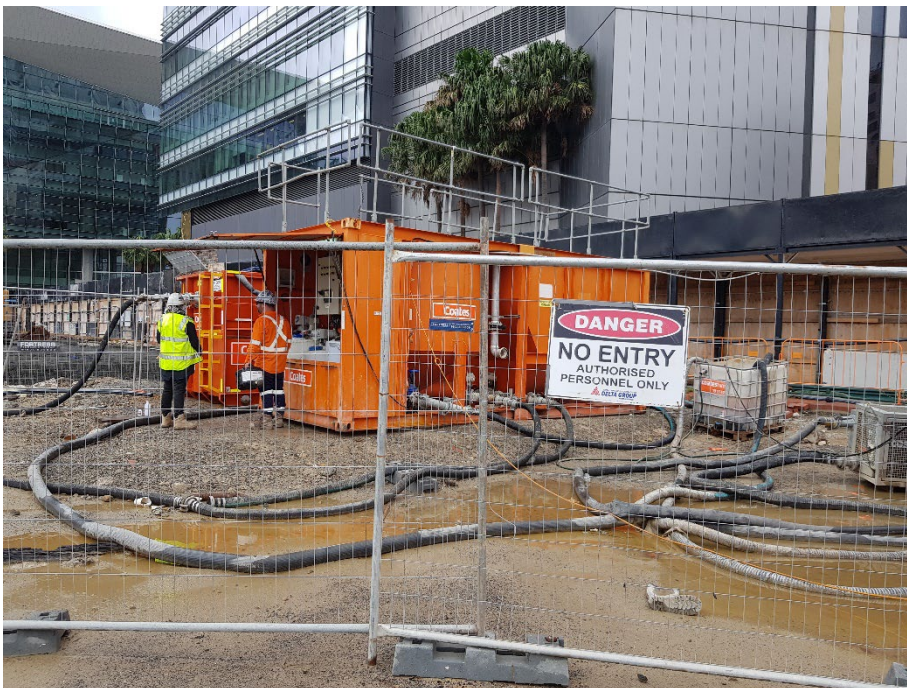
Photo 30: Coates Environmental Engineer and Electrician maintaining the Dewatering Treatment Plant. 23/01/24
