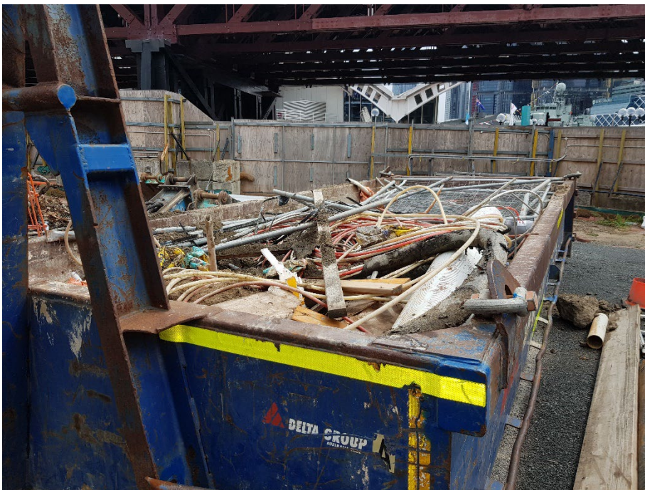
Photo 36: A waste skip of general solid waste containing miscellaneous construction waste. 23/01/24
