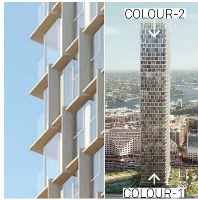
FA-02 PROFILED ALUMINIUM OR SIMILAR ELEMENTS. TEXTURED MATTE FINISH. GRADIENT EFFECT.
