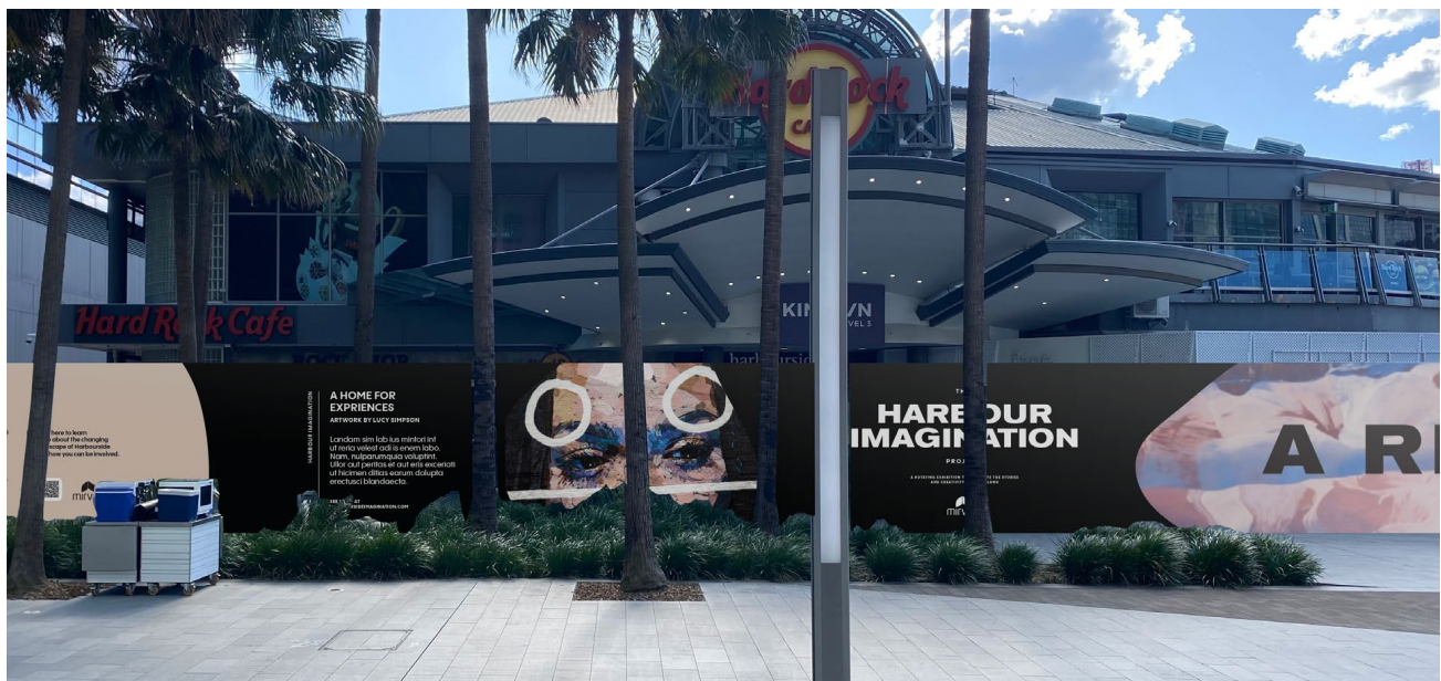
Figure 3 Draft Hoarding branding example in-situ
