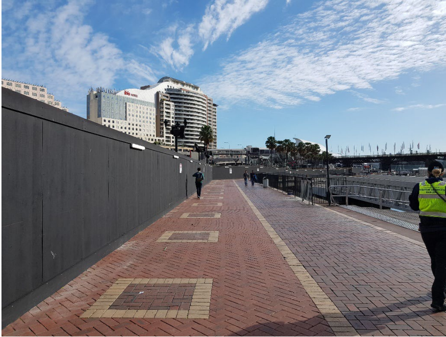
Photo 7: Public way along the eastern site boundary with hoarding, looking towards the north with Cockle Bay on the right.
