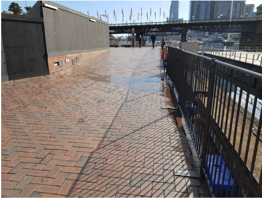
Photo 5: Public way along the eastern site boundary with hoarding, looking towards Pyrmont Bridge. Minor water seepage from the site draining towards Cockle Bay on the right.
