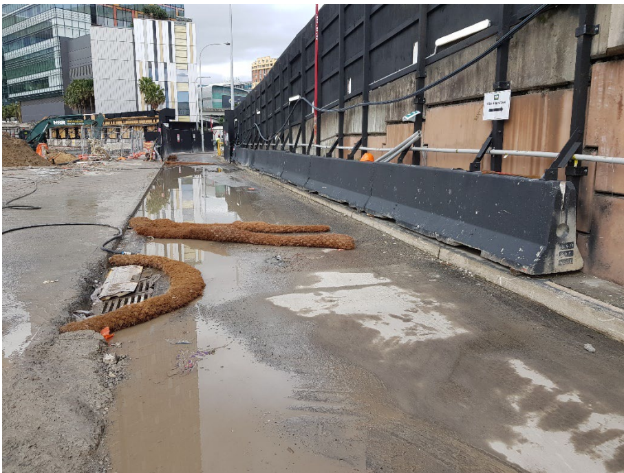
Photo 14: Bunding around stormwater drains near the exit, looking towards the south.
