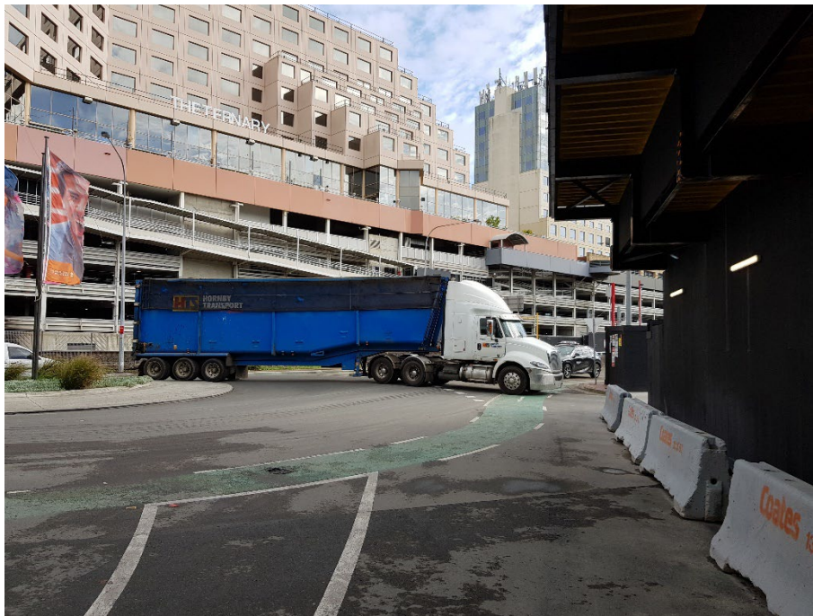
Photo 10: Truck heading towards the main site entrance from Darling Drive roundabout.
