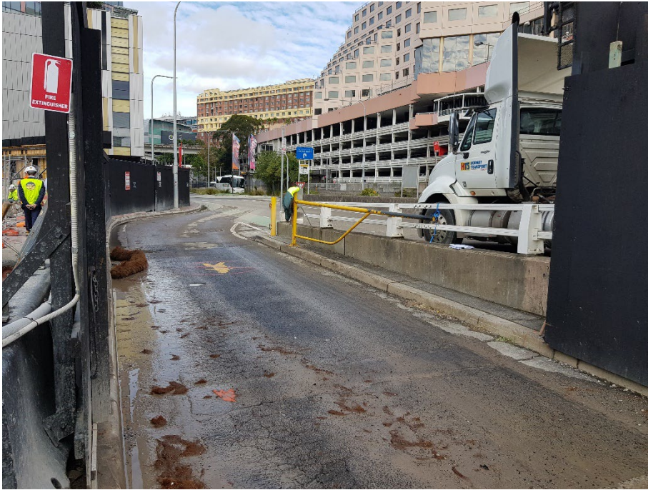
Photo 13: Western site entrance and exit to Darling Drive.
