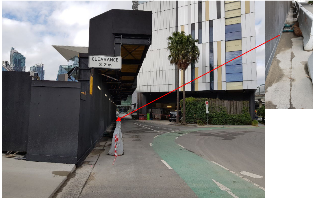
Photo 11: View to the south from the main site entrance on Darling Drive with Sofitel on the right of the laneway. Stormwater drain with sediment protection.
