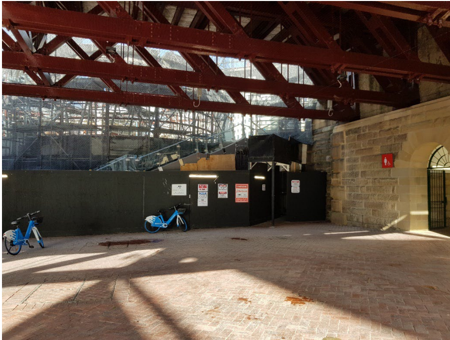
Photo 1: View of the northern site boundary from under Pymont Bridge.
