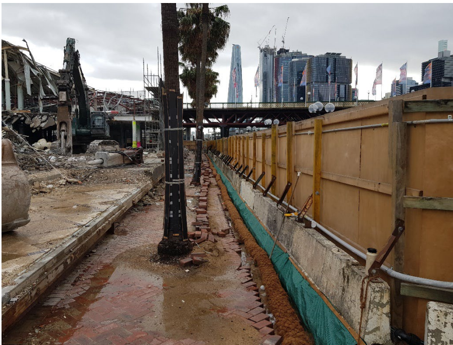
Photo 16: Tree protection along the eastern boundary of the site. Trees are scheduled for transplanting. Sediment fencing along eastern boundary on the right.
