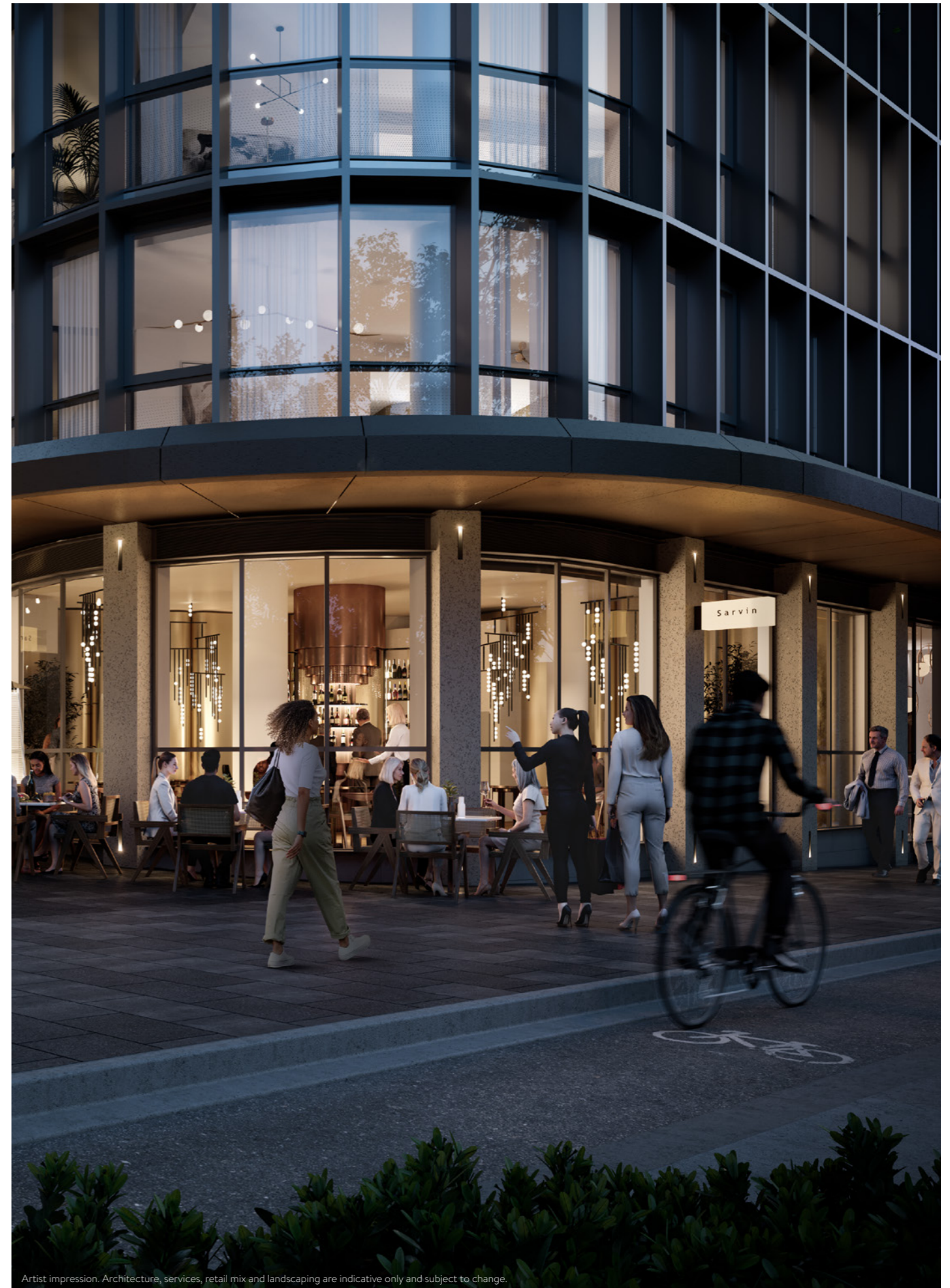
Artist impression. Architecture, services, retail mix and landscaping are indicative only and subject to change.
