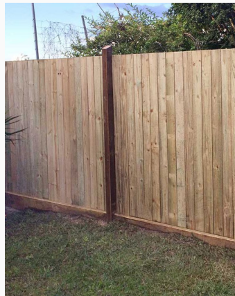
Type 1 - Timber Paling Fence
