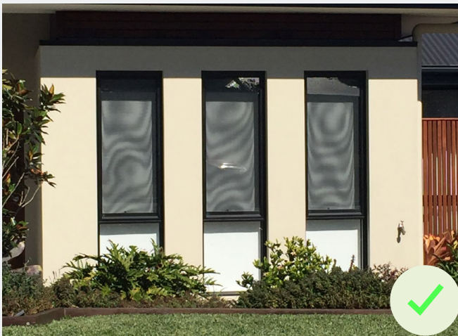
Any security screen visible to the street must be of a simple profile
