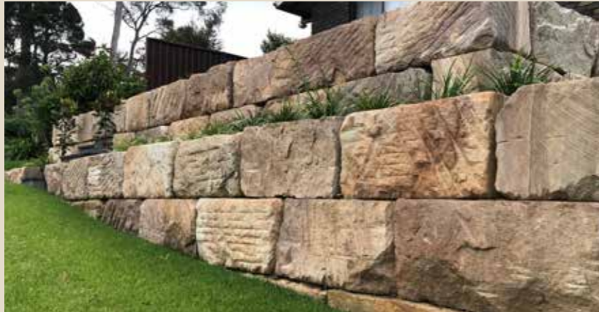
Figure 2 – Sandstone log retaining wall
