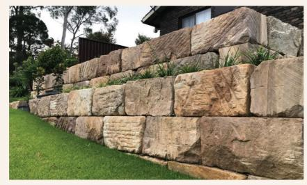
Figure 2 - Sandstone log retaining wall
