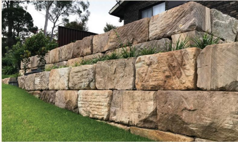
Figure 2 - Sandstone log retaining wall
