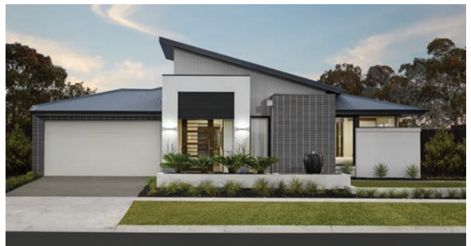
Skillion Roof - Metricon Homes (Botanica)
