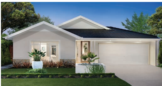
Gable Roof - Porter Davis Homes
