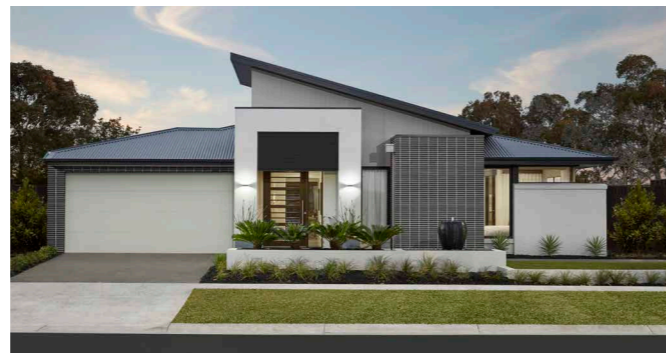
Skillion Roof - Metricon Homes (Botanica)
