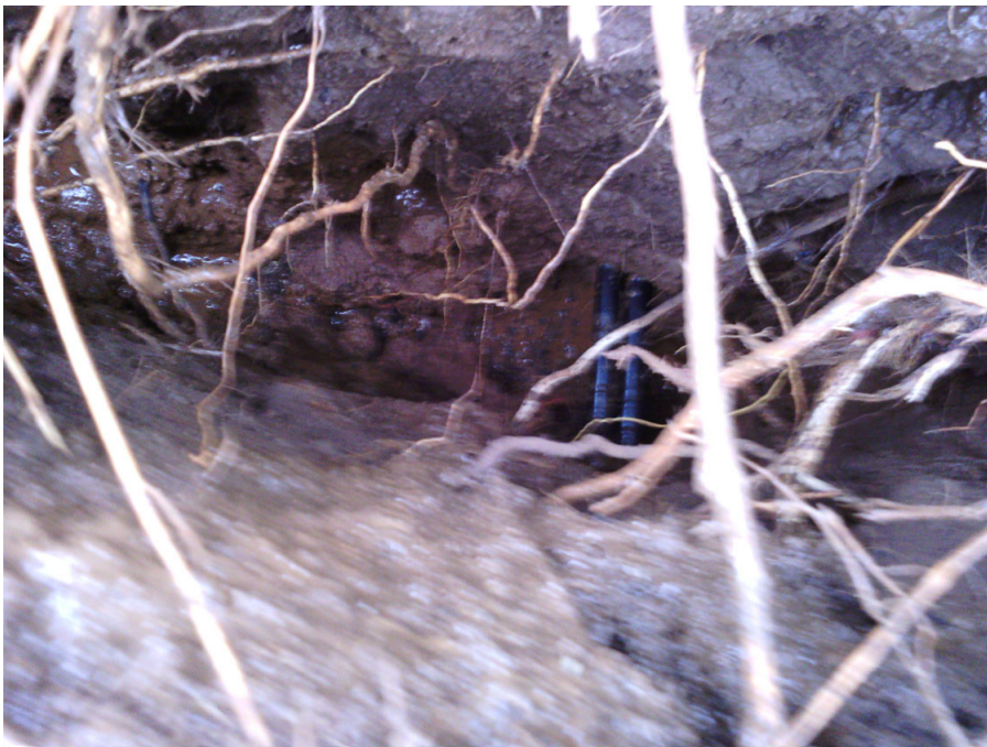
PH 7 - 2 x Direct buried comms cables
