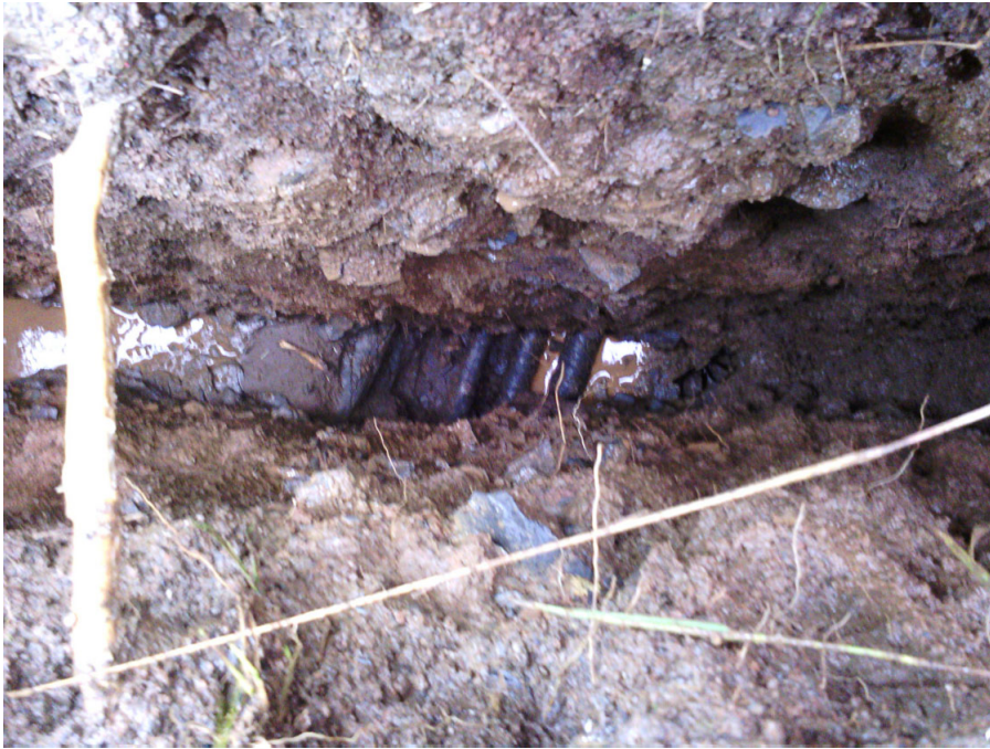
PH 11 - 3 x Direct buried cables
