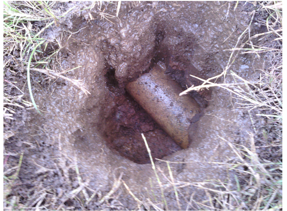
PH 1 - 100mm Water - Asbestos
