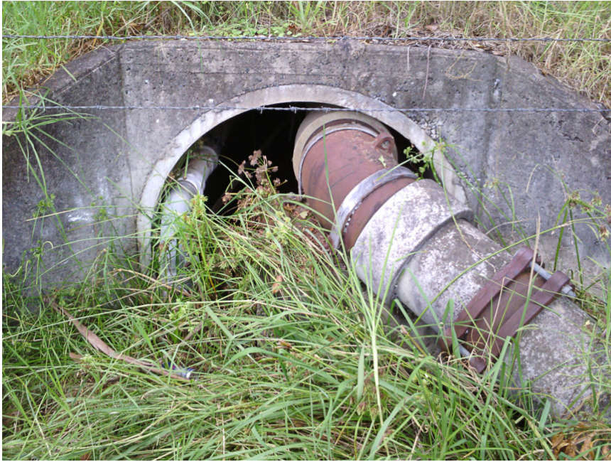
17. 250mm Water and Redundant 100mm Water, Comms turns inside Culvert
