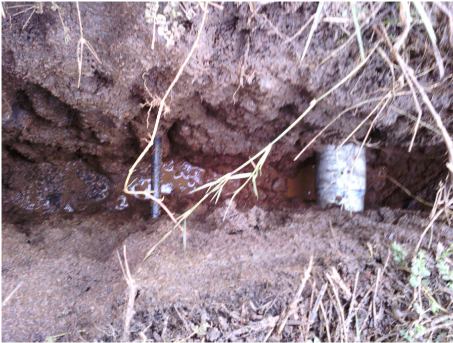
PH 8 - 100mm Comms and direct buried cable
