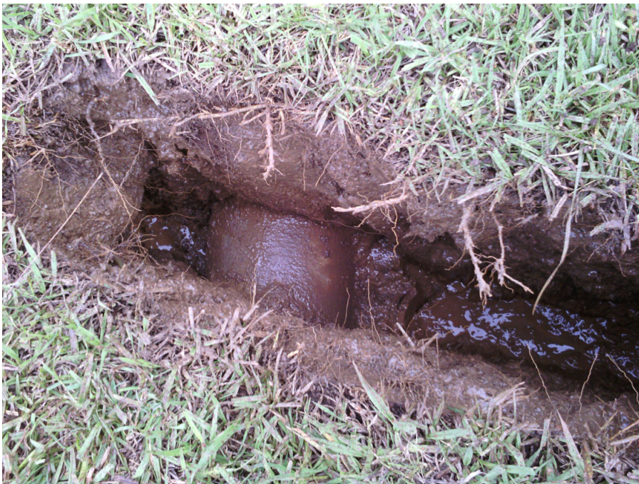
PH 5 - 250mm Water - Asbestos
