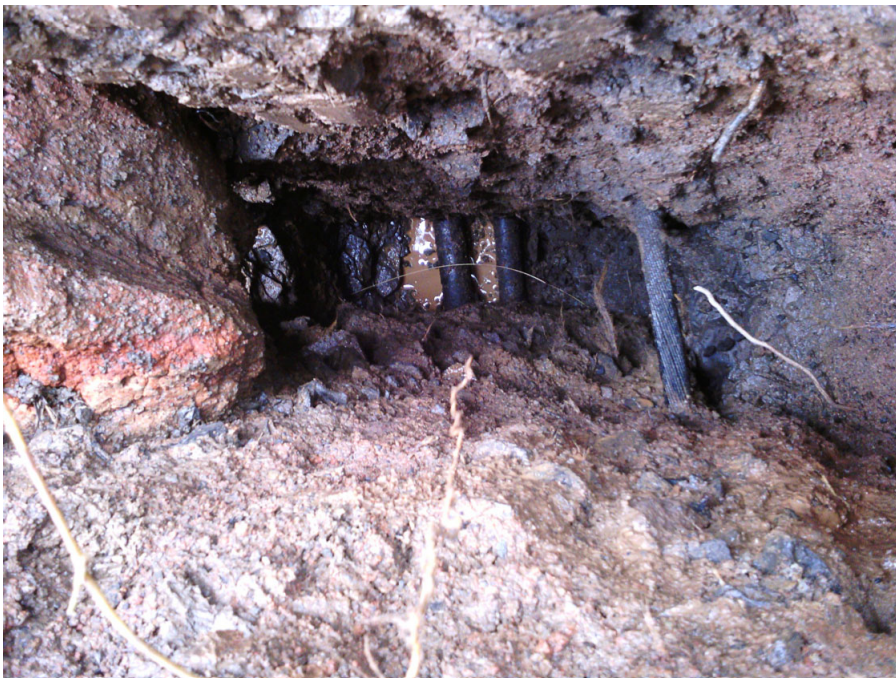
PH 10 - 3 x Direct buried cables
