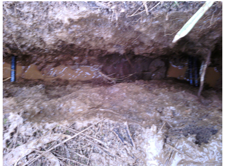
PH 7 - 3 x Direct buried comms cables
