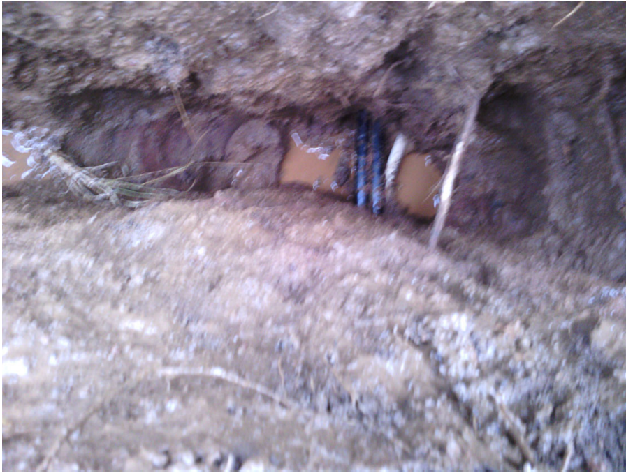
PH 6 - 2 x Direct buried comms cables
