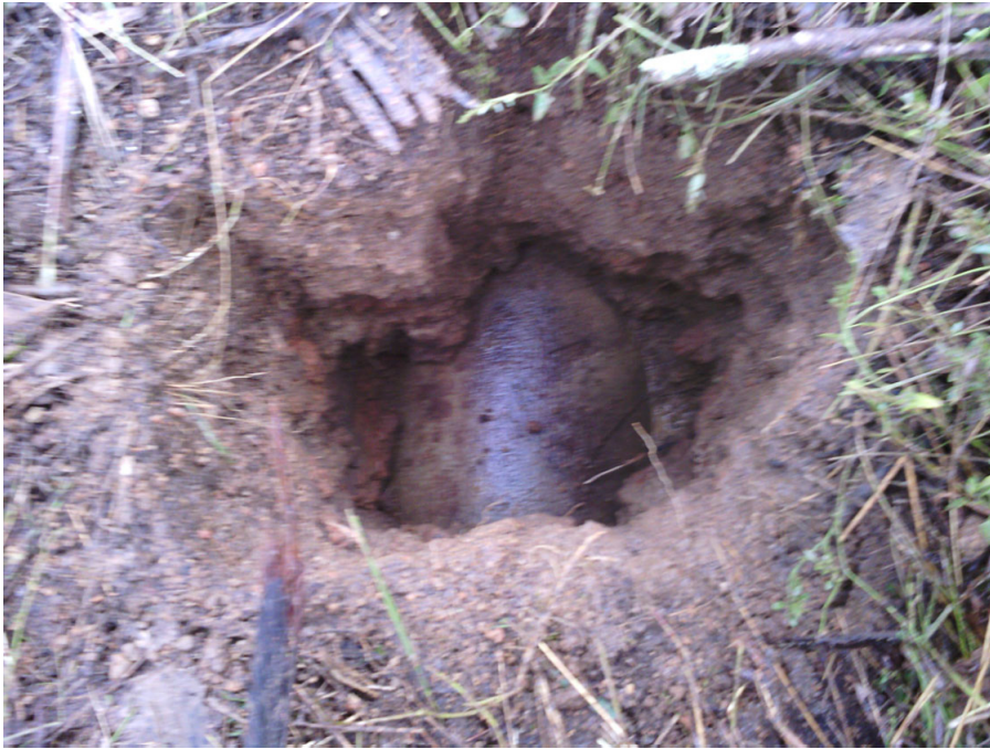
PH 3D - 250mm Water - Asbestos
